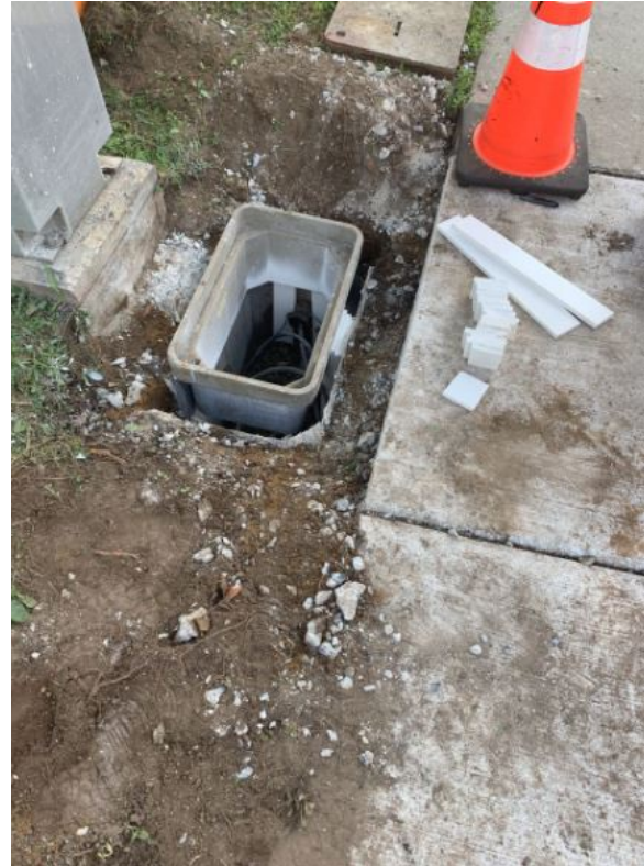
Figure 5: Existing junction box replaced and lowered
