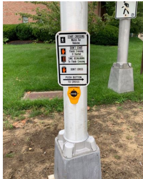
Figure 3: Push button installed
