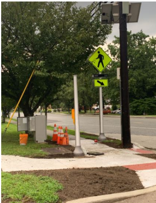
Figure 2: Push button pole and crosswalk sign
