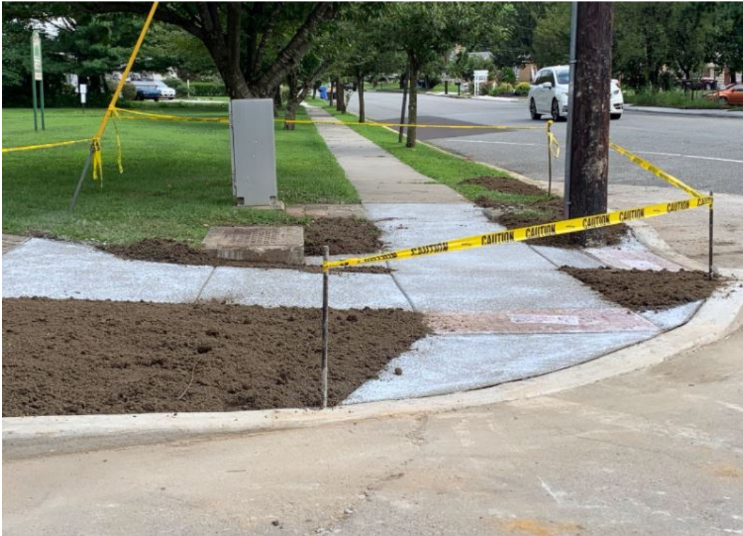
Figure 1: Concrete curb ramp placed
