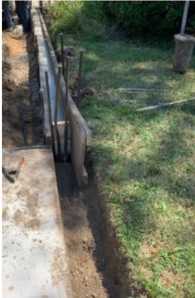
Figure 4: Concrete curb placed
