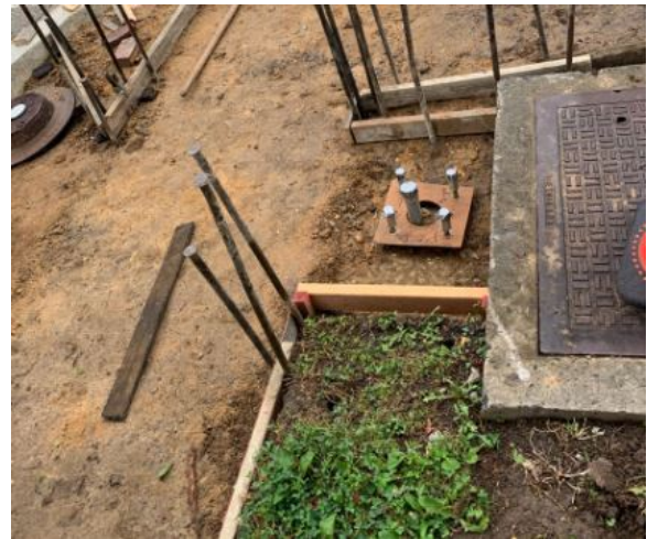
Figure 5: Curb ramp forms and PED push button foundation
