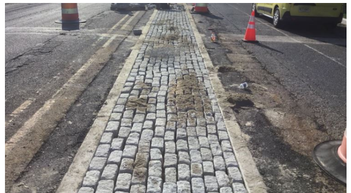
Figure 3: Cobblestone paver installation
