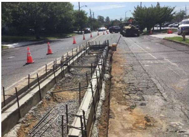
Figure 2: Concrete edge restraint placed
