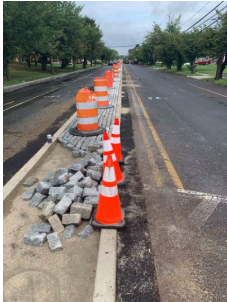
Figure 1: Concrete center island construction
