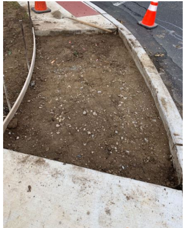
Figure 5: Preparation for concrete sidewalk placement
