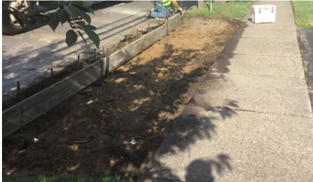
Figure 4: Preparation for concrete driveway placement
