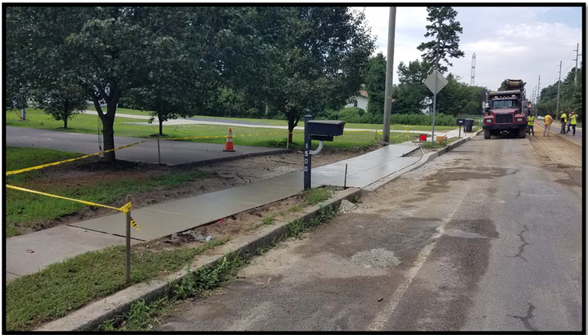
Photograph 1 – Concrete sidewalk and driveway apron poured at 1500 Jarvis Road.
