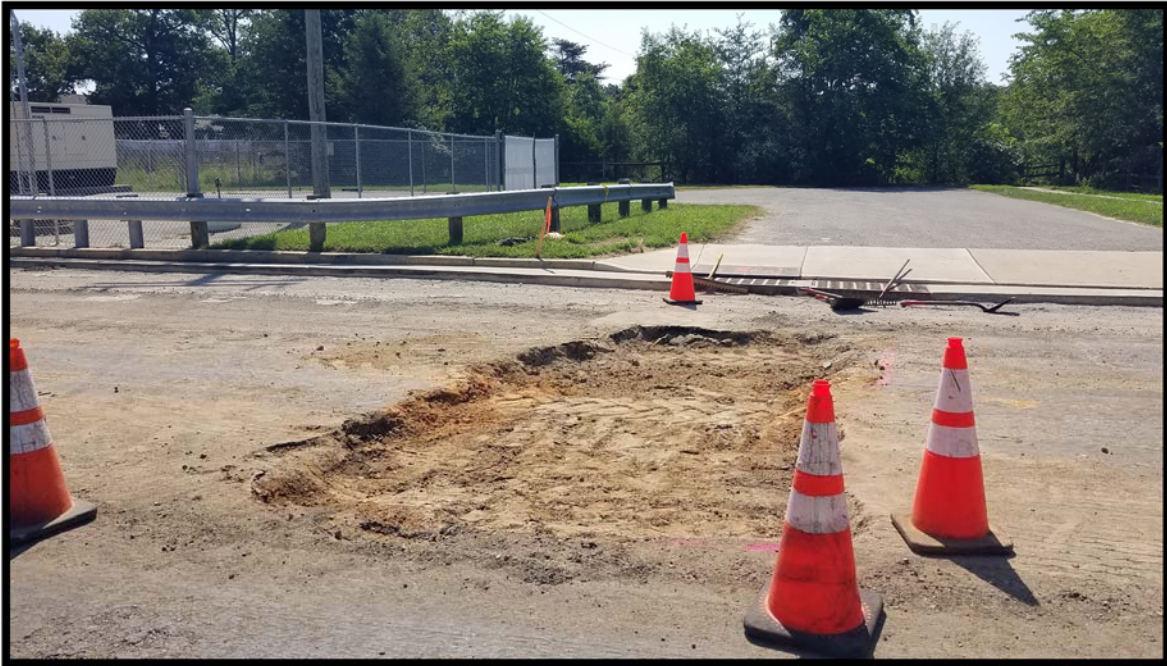
Photograph 6 – Excavation for base repairs near GTMUA Pump Station.
