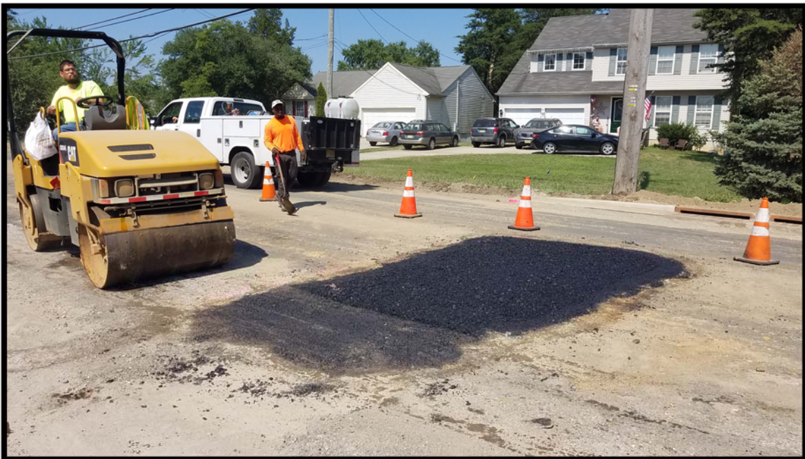
Photograph 7 – Compaction of Hot Mix Asphalt base repairs near GTMUA Pump Station.
