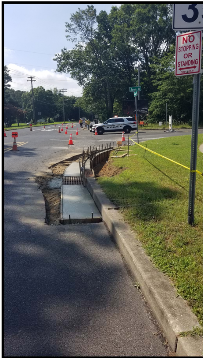
Photograph 8 – New curb and concrete gutter at the Jarvis Road and Kearsley Road intersection.
