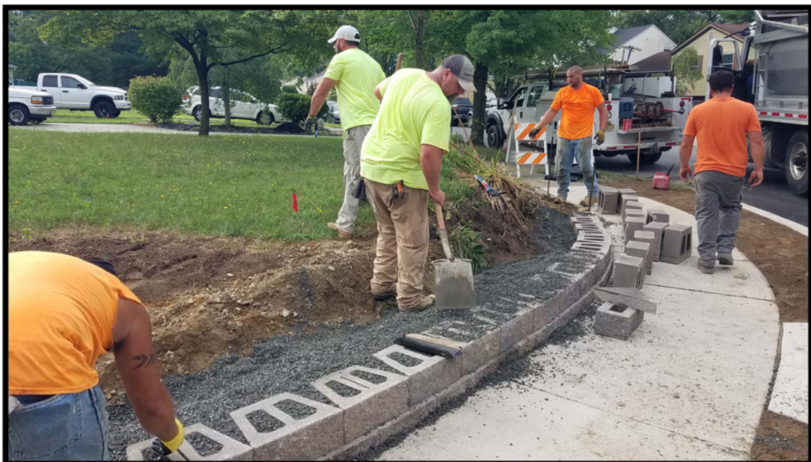
Photograph 11 – Segmental Retaining Wall being installed at Mary Ellen Lane intersection.
