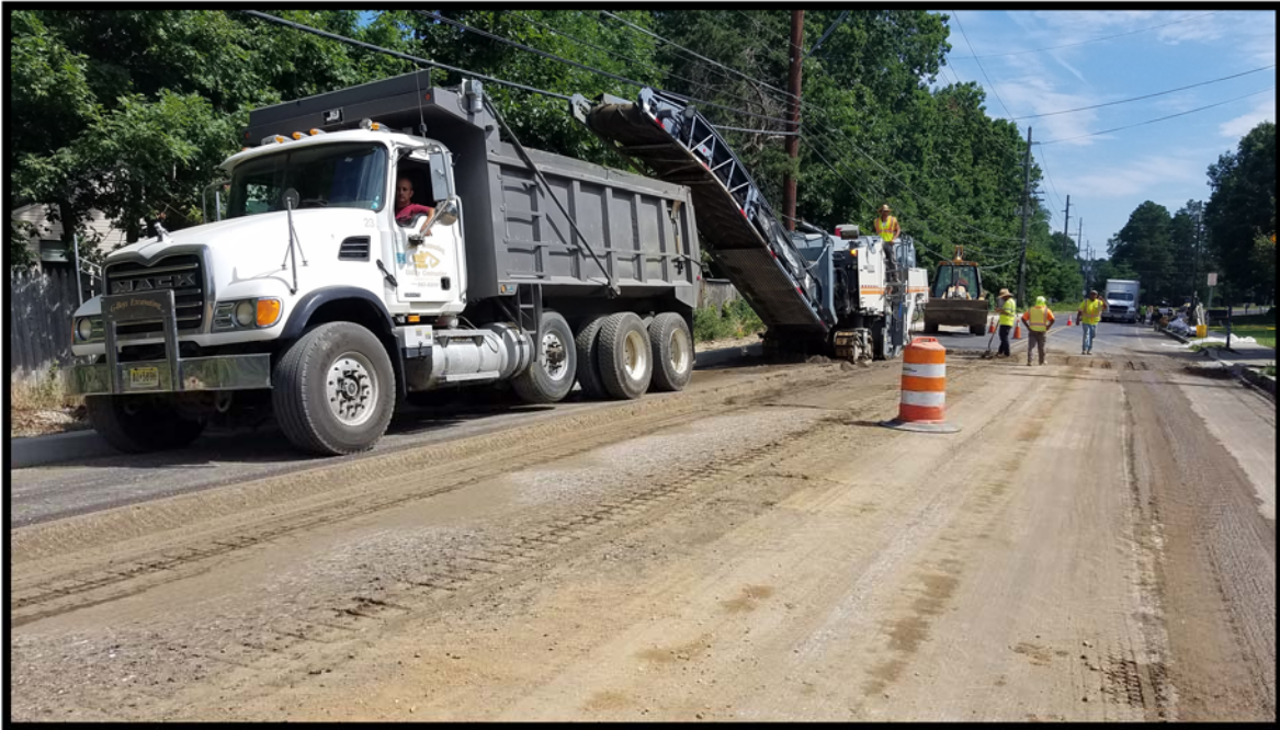
Photograph 2 – Milling of the reclaimed subbase material to subgrade elevation prior to placement of Hot Mix Asphalt Base Course.
