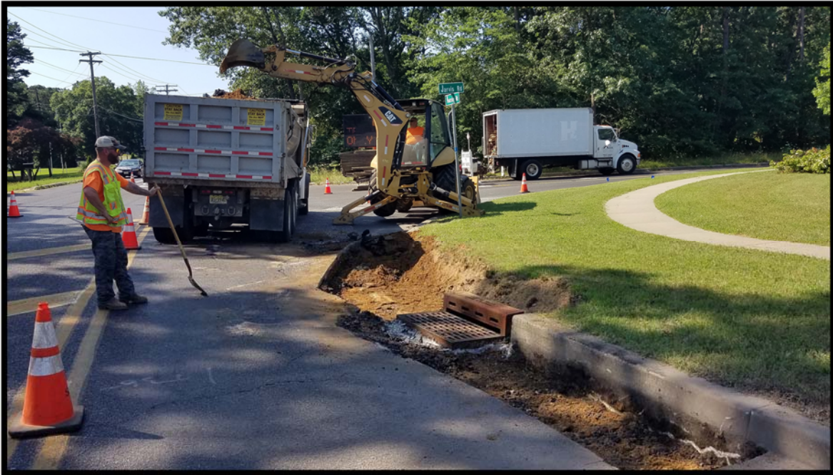
Photograph 4 – Excavation for new curb at the Jarvis Road and Kearsley Road intersection.
