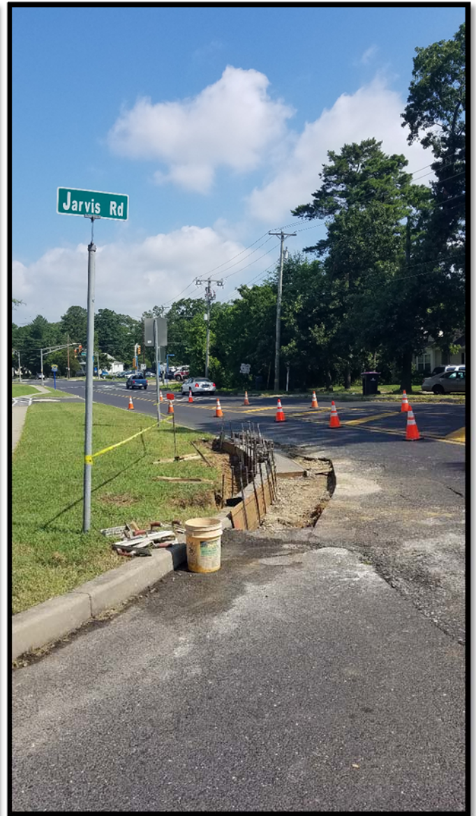
Photograph 9 – New curb and concrete gutter at the Jarvis Road and Kearsley Road intersection.
