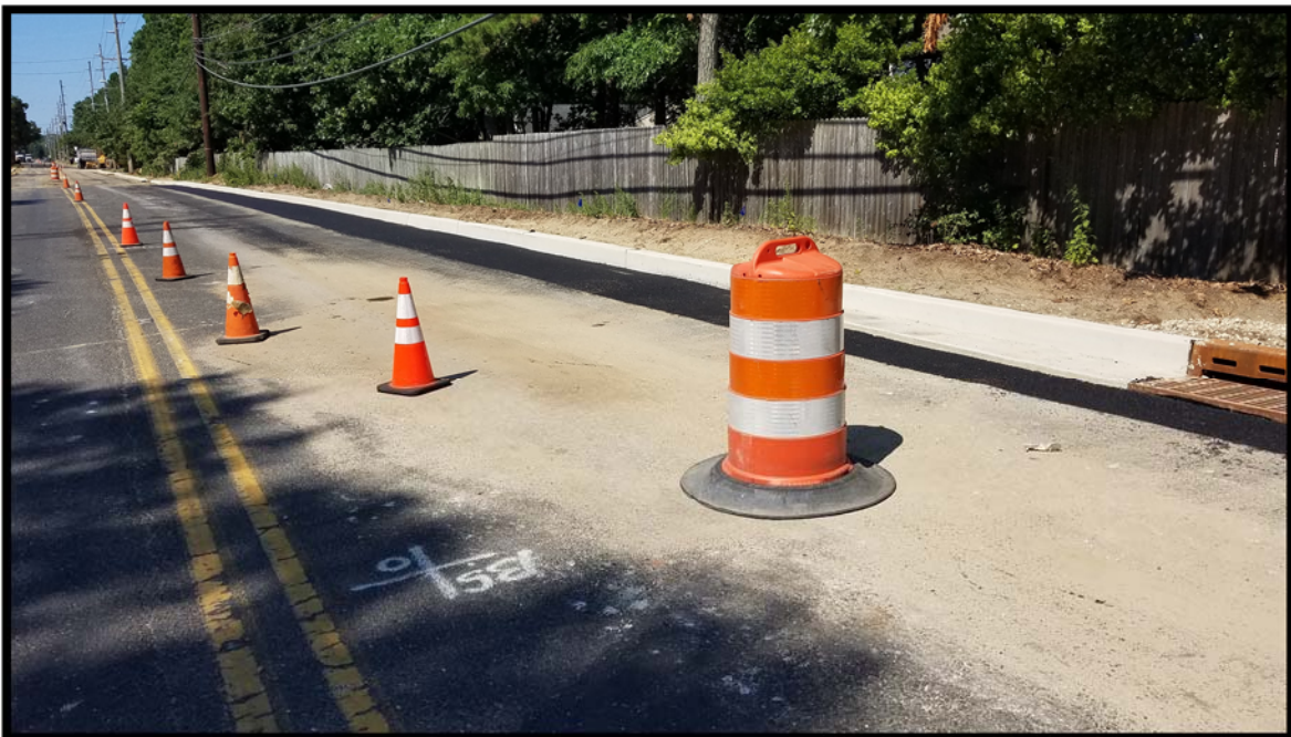
Photograph 5 – Hot Mix Asphalt pavement restoration adjacent to concrete curb and gutter within milling limits of project.
