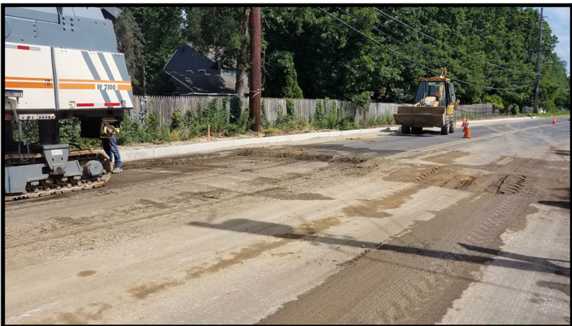
Photograph 3 – Milling of the reclaimed subbase material to subgrade elevation prior to placement of Hot Mix Asphalt Base Course. Note transition at limits of reclamation area.
