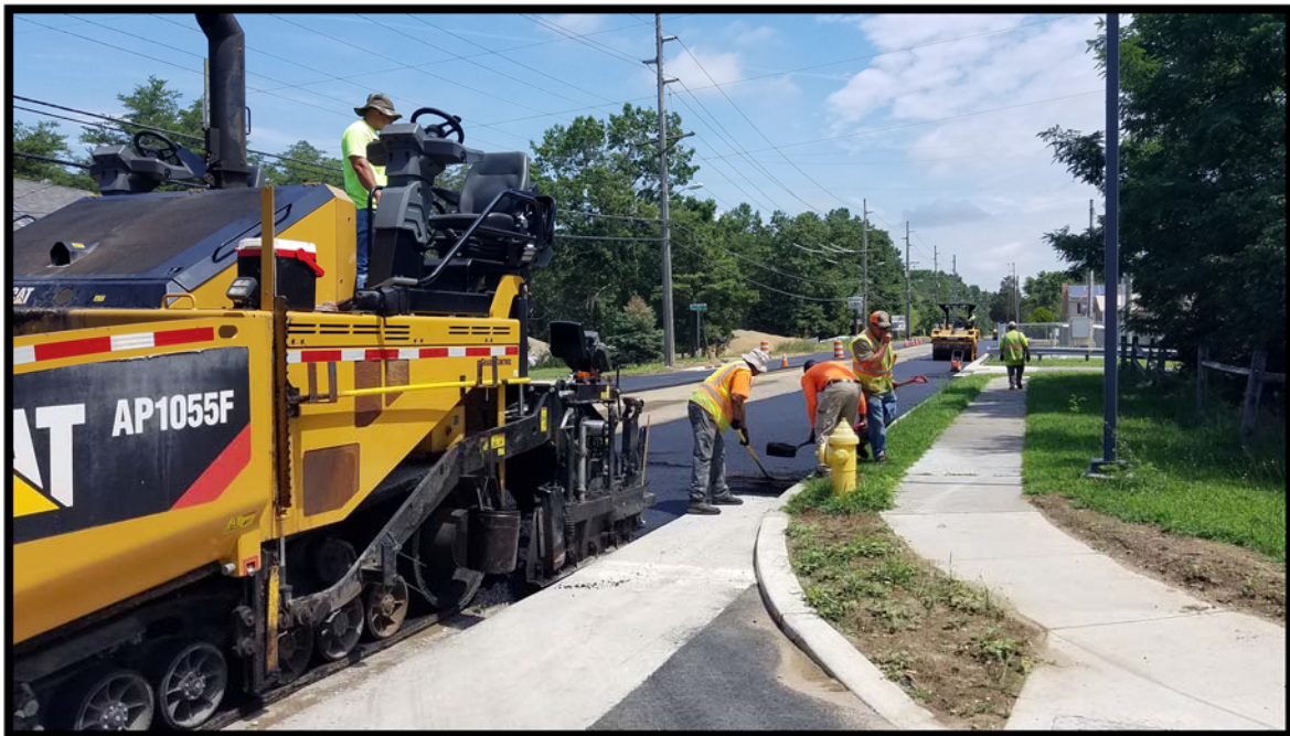
Photograph 10 – Hot Mix Asphalt Base Paving being installed on Jarvis Road.
