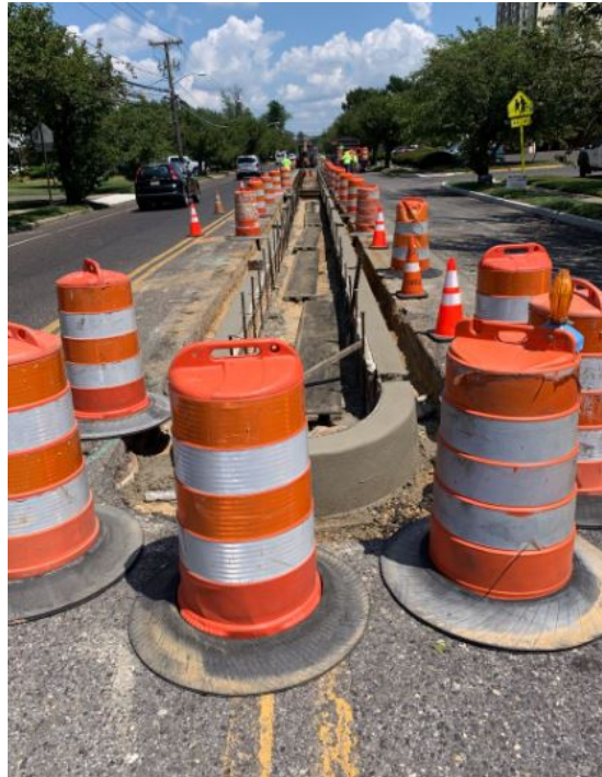
Figure 1: Concrete center island curb placed
