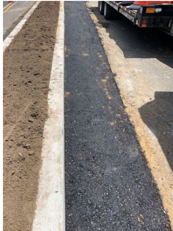
Figure 5: Pavement restoration by concrete center island
