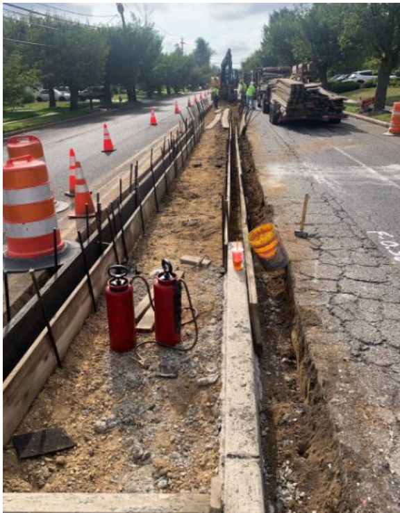
Figure 2: Concrete restraint curb forms
