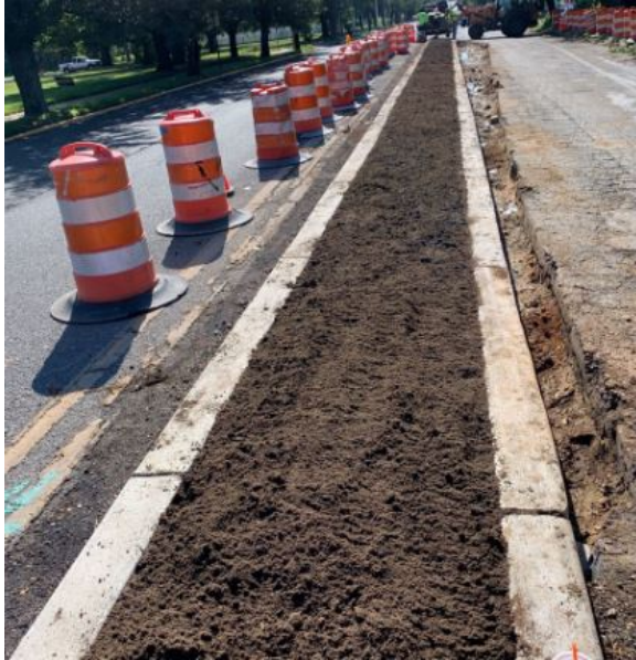
Figure 4: Topsoil placed within center island
