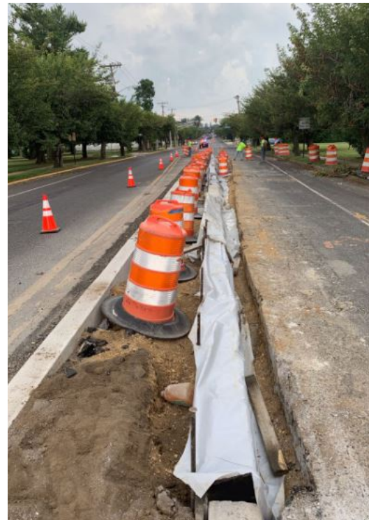
Figure 3: Concrete island curb placed and protected
