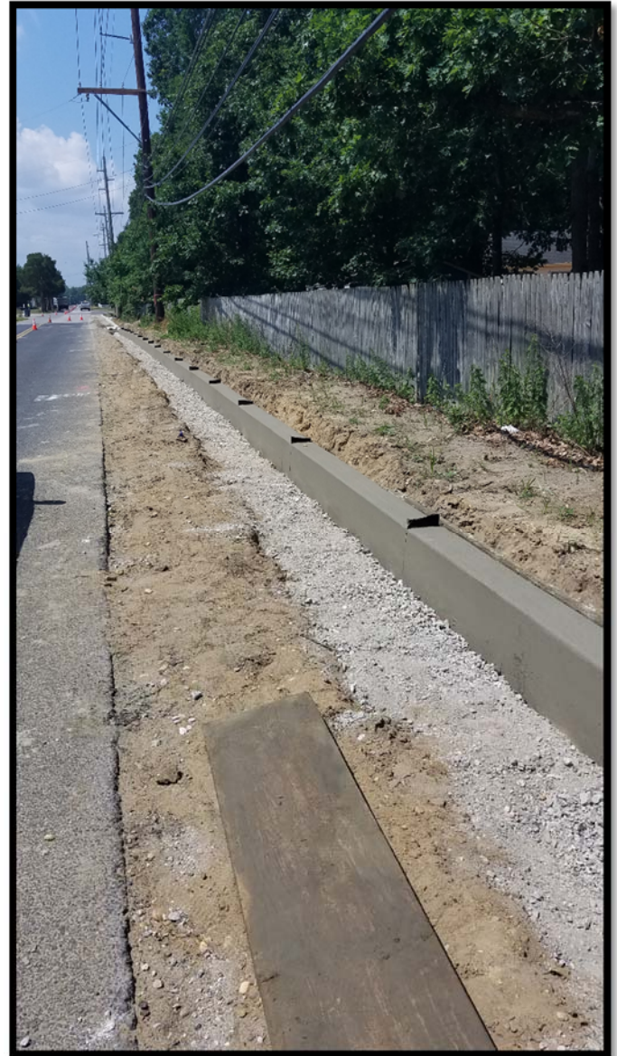
Photograph 3 – Newly poured concrete for the vertical curb between stations 132+70L and 134+40L.
