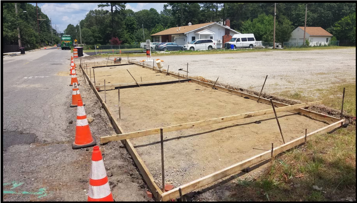
Photograph 6 – Forms placed and subgrade preparation in progress for driveway concrete pour.
