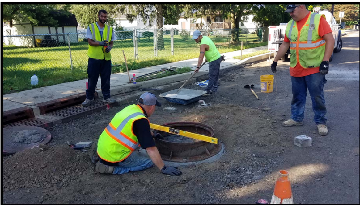
Photograph 5 – Manhole casting being reset to proper grade and pitch.
