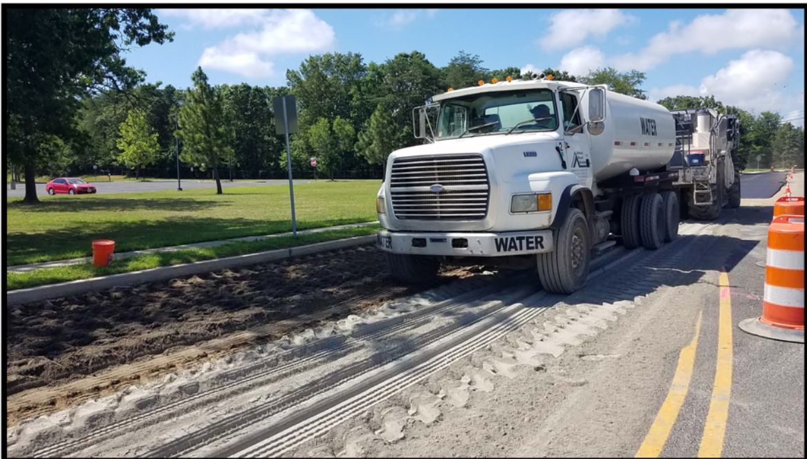
Photograph 7 – Full depth reclamation with cement admixture progressing on the right side of Jarvis Road from station 115+00 to 122+00.
