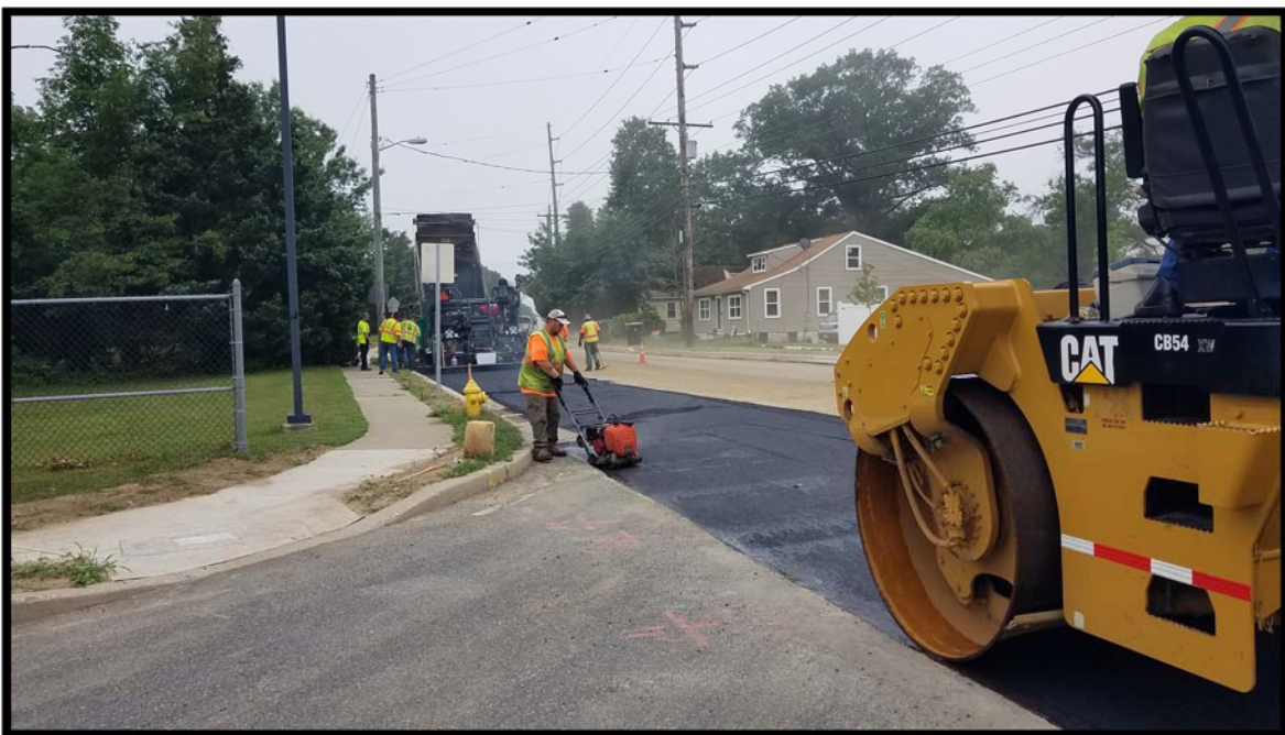
Photograph 9 – Hot Mix Asphalt Base Course being installed between stations 91+47 and 115+00 over the reclaimed subbase installed the previous week and fine graded this week.
