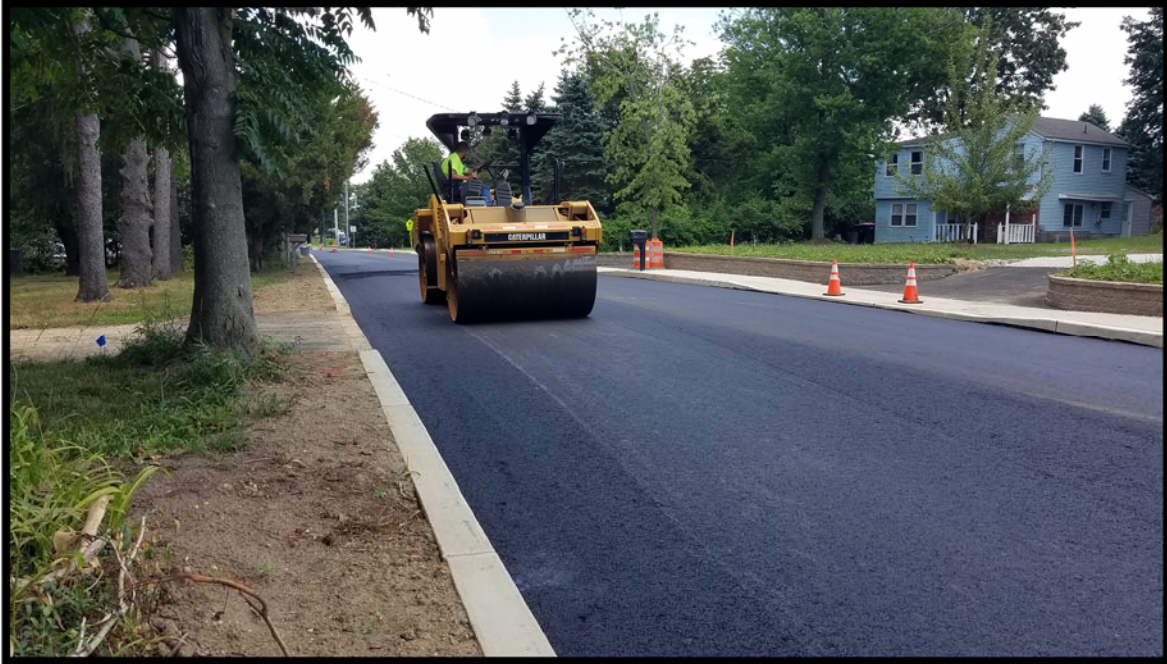
Photograph 10 – Hot Mix Asphalt Base Course being compacted with vibratory roller between stations 91+47 and 115+00.
