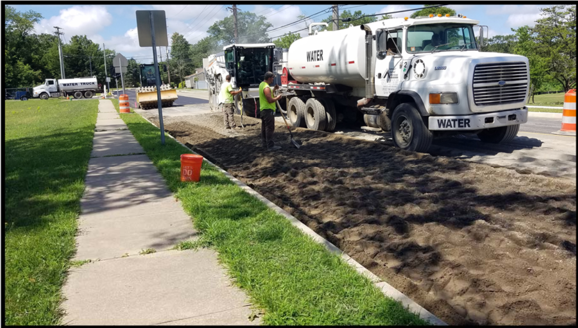
Photograph 8 – Second pass of full depth reclamation with cement admixture progressing on the right side of Jarvis Road from station 115+00 to 122+00.
