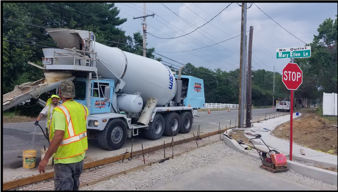
Photograph 4 – Reinforced concrete swale formed out at Mary Ellen Lane and prepared for concrete pour.
