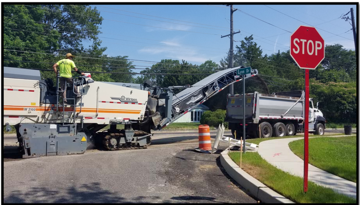
Photograph 1 – Milling of the reclaimed subbase material to subgrade elevation prior to placement of Hot Mix Asphalt Base Course.
