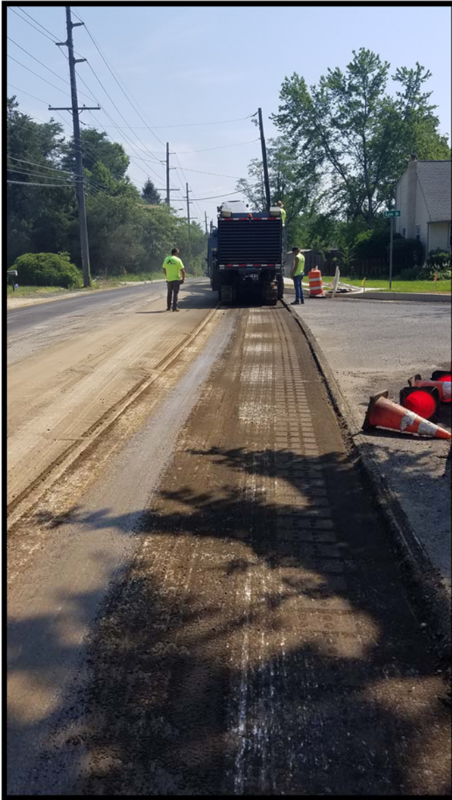
Photograph 2 – Milling of the reclaimed subbase material to subgrade elevation prior to placement of Hot Mix Asphalt Base Course.
