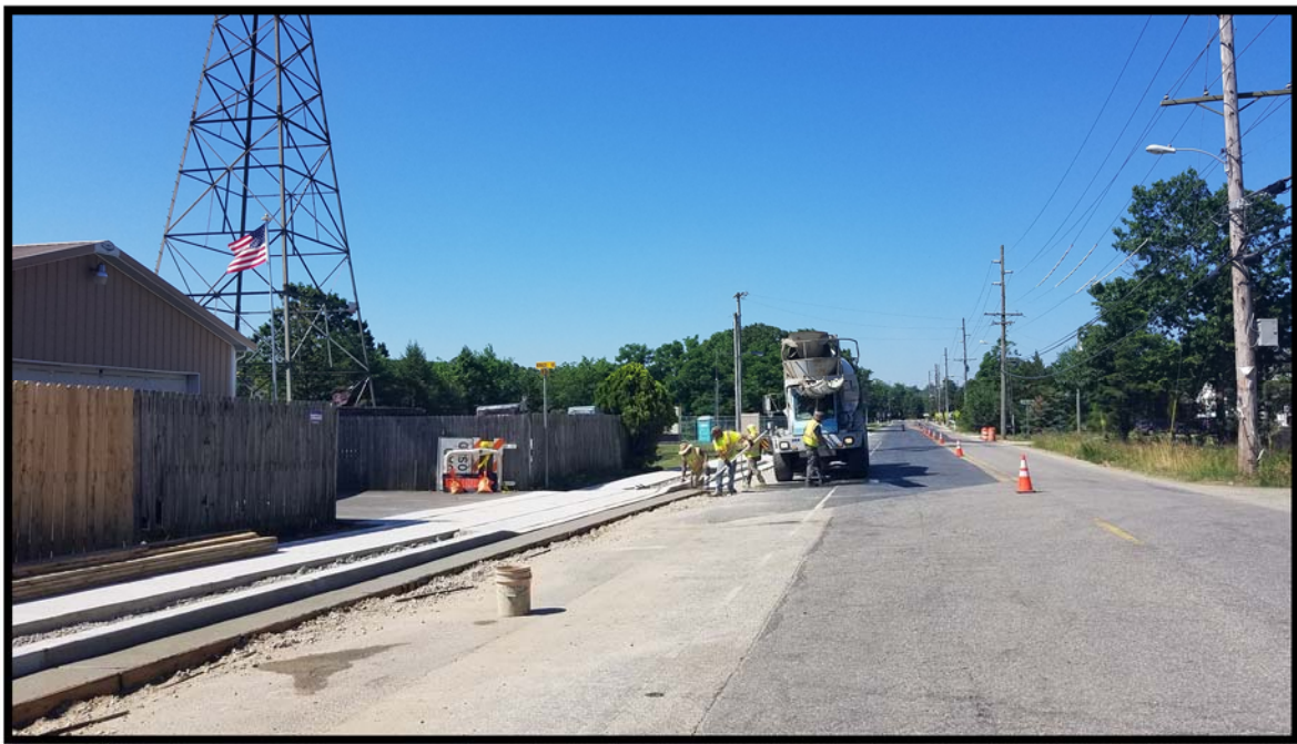
Photograph 1 – Concrete gutter being installed between stations 122+90R and 124+25R.
