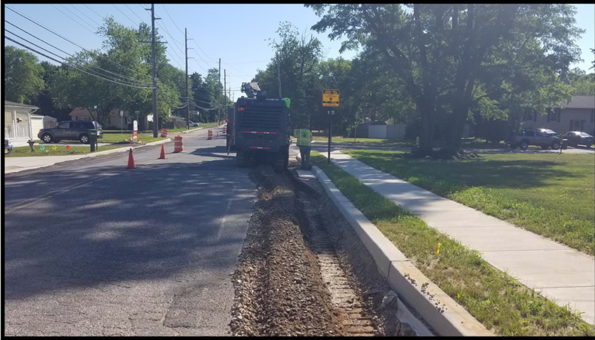
Photograph 2 – Preparing gutterline for full depth reclamation of the roadway.
