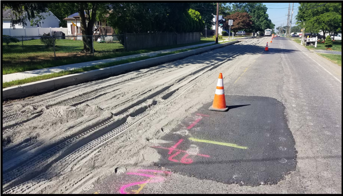
Photograph 4 – Full depth reclamation admixture of cement placed prior to being mixed with the reclaimer/stabilizer.
