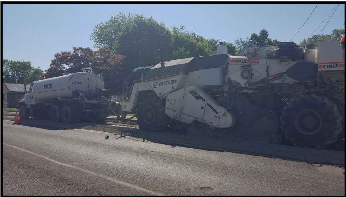
Photograph 5 – Water truck and reclaimer/stabilizer in use along northbound lanes of Jarvis Road.
