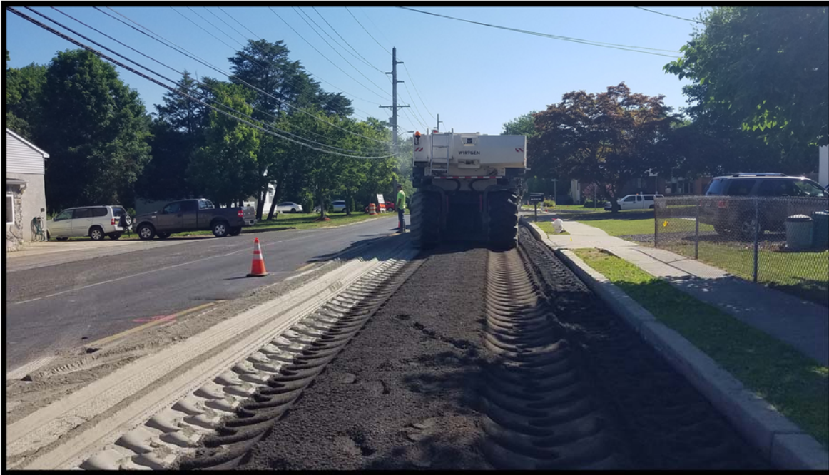
Photograph 6 – Reclaimed mixture of existing, pulverized roadway base, water and cement.
