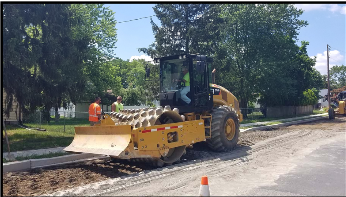
Photograph 7 – Sheep's foot roller compacting reclaimed mixture of existing, pulverized roadway base, water and cement.
