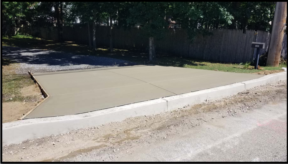
Photograph 10 – Concrete apron installed at 1465 Jarvis Road.
