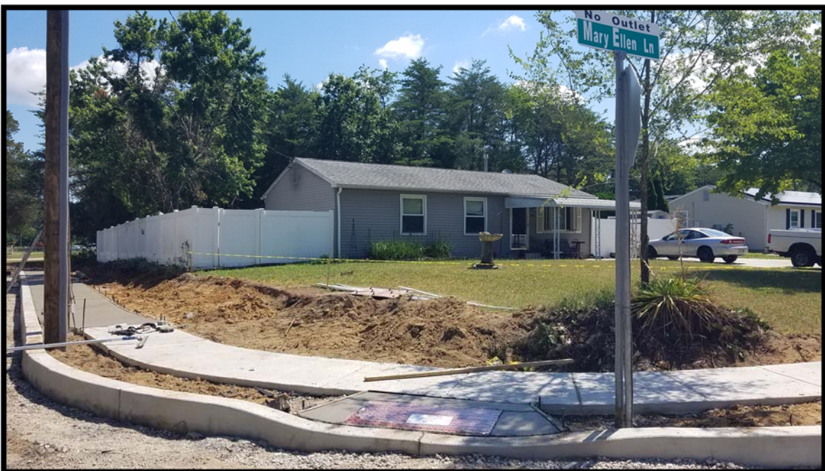
Photograph 9 – Curb, sidewalk and handicapped accessible ramp installed at Jarvis Road and Mary Ellen Lane.
