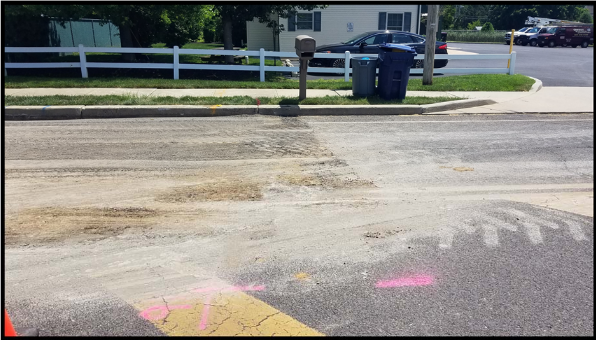
Photograph 8 – Reclaimed roadway base compacted and rolled at transition from mill & overlay section to full depth reclamation section of the project.
