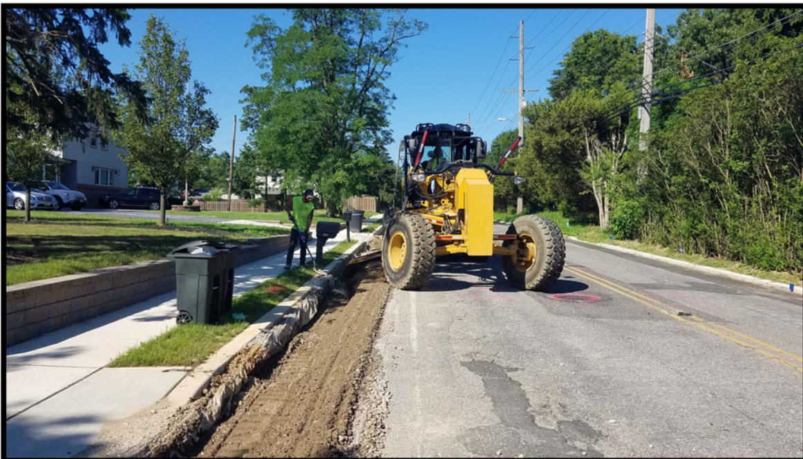
Photograph 3 – Preparing gutterline for full depth reclamation of the roadway.
