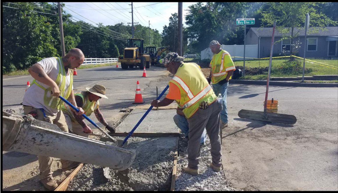
Photograph 10 – Concrete swale being installed at southern half of Mary Ellen Lane.
