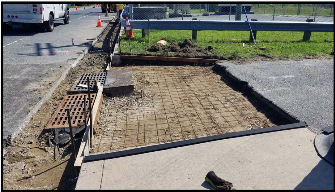
Photograph 1 – Driveway Apron at GTMUA Pump Station prepared for concrete pour.
