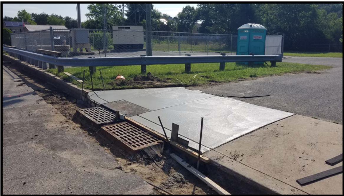
Photograph 7 – Concrete pour completed for driveway apron at GTMUA Pump Station.
