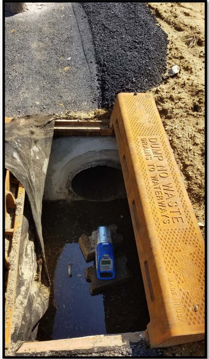
Photograph 3 – Laser level being utilized for pipe alignment of 18" RCP.
