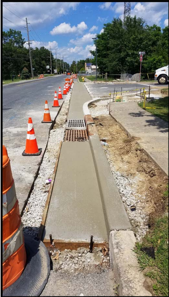
Photograph 4 – Concrete gutter and concrete swale installed at north entrance to Union Valley Elementary School.
