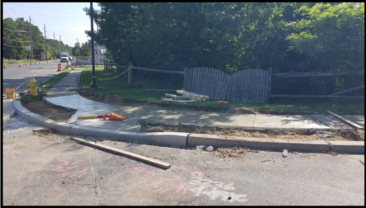
Photograph 6 – Handicapped Accessible Ramp installed at the north side of the north entrance to Union Valley Elementary School.
