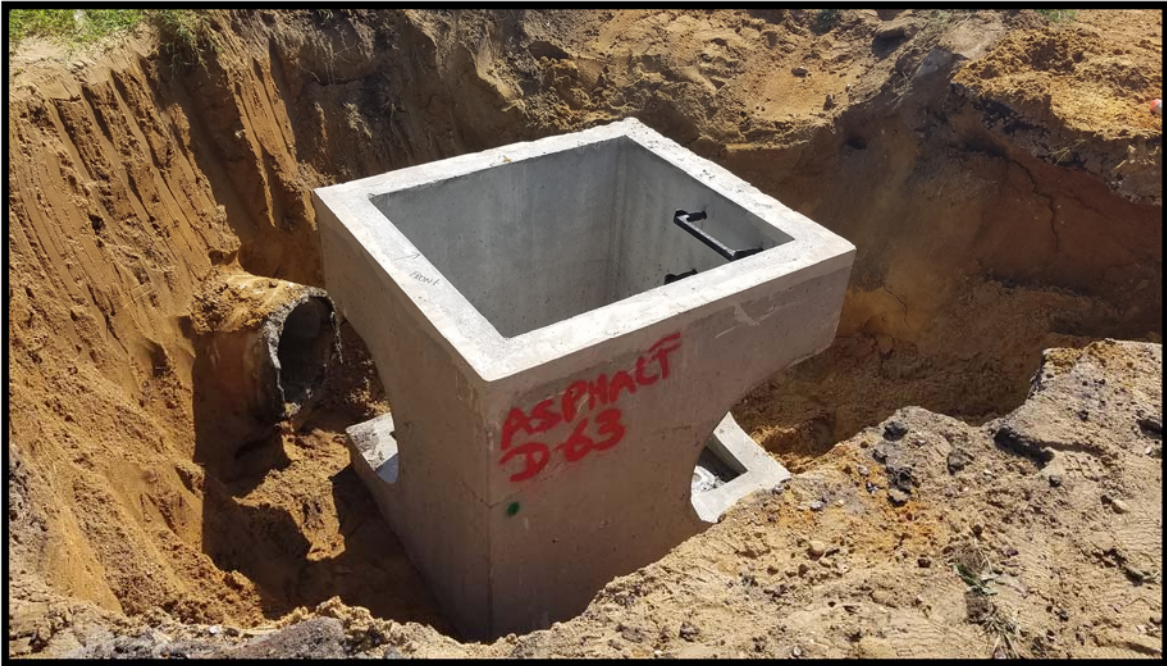
Photograph 8 – Inlet D-63 being installed near station 137+80L.
