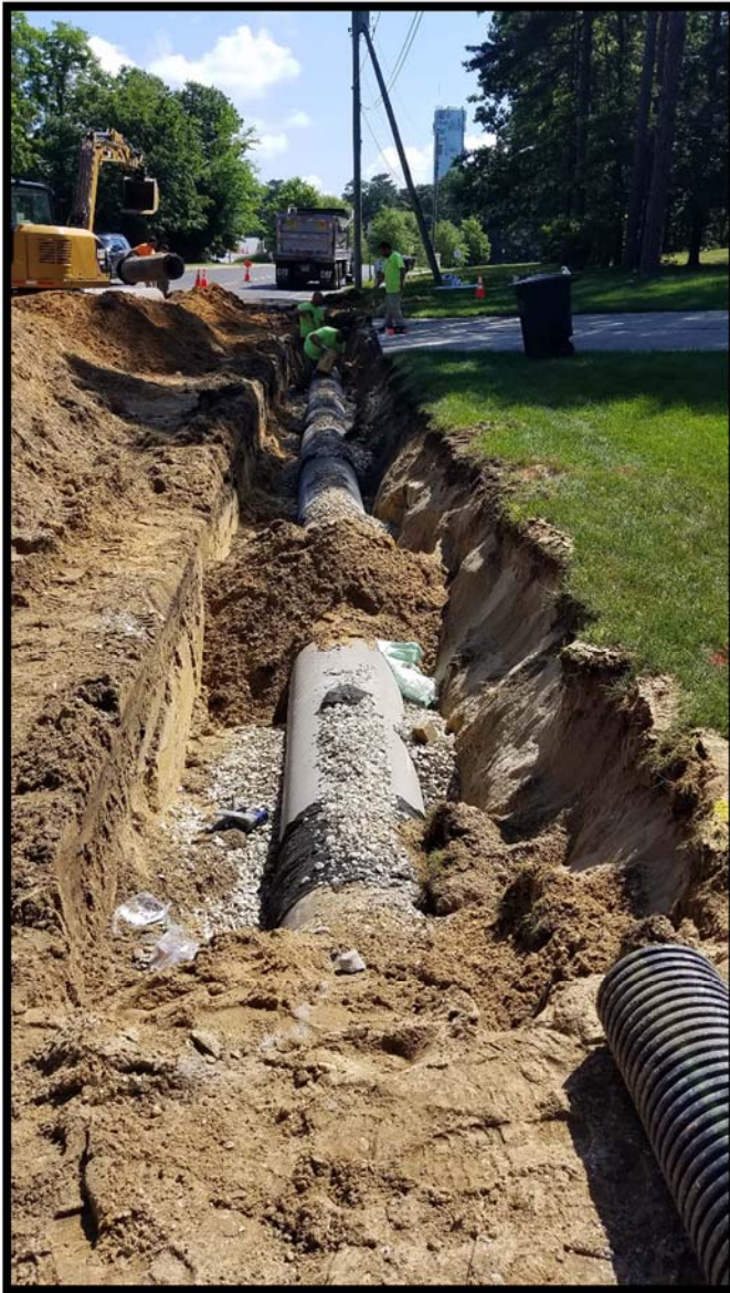
Photograph 2 - 18" RCP being installed near inlet D-64
