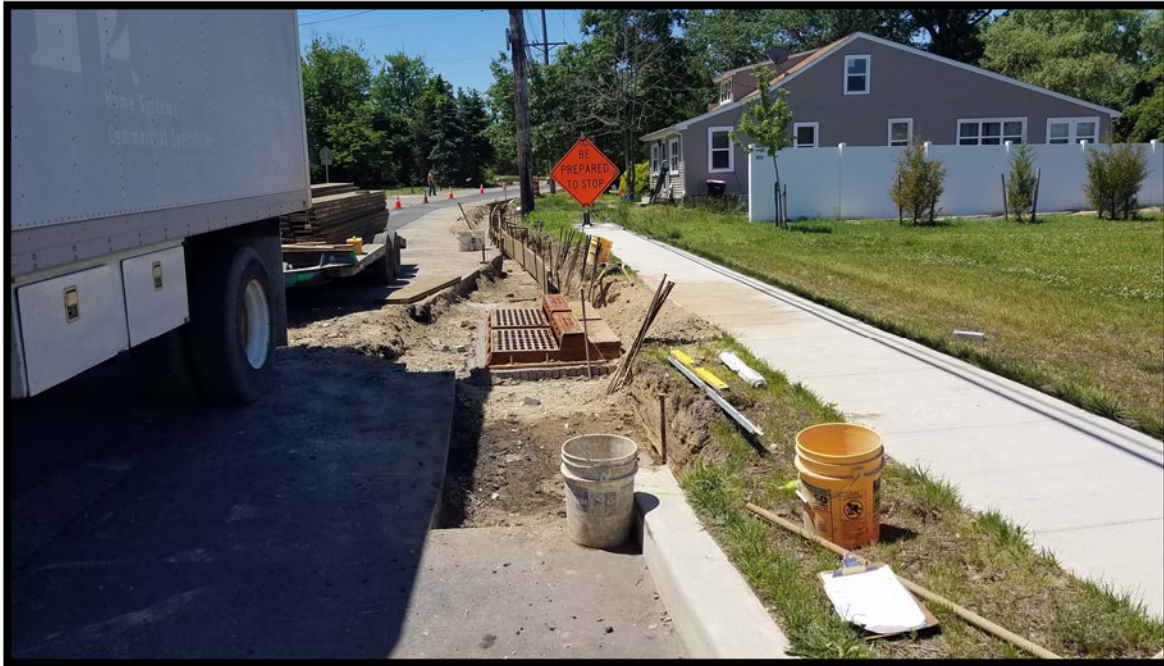
Photograph 2 – Preparing for installation of curb and gutter adjacent to inlet D-42 near station 112+90L.
