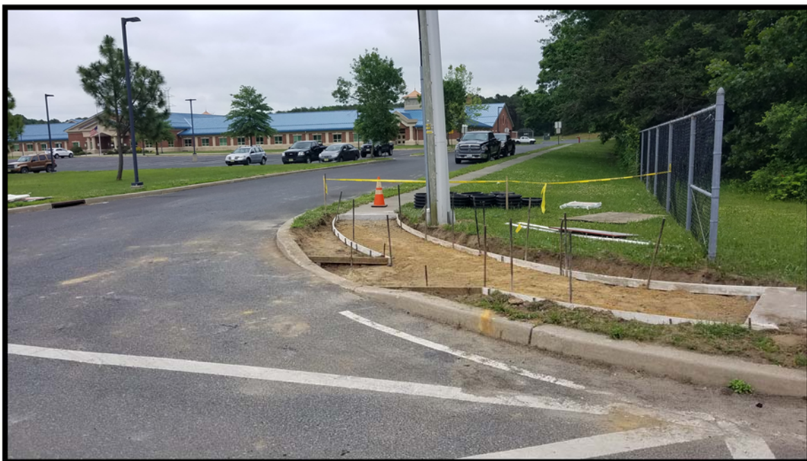
Photograph 3 – Forms and subgrade prepared for sidewalk and handicapped accessible ramp installation adjacent to Union Valley Elementary School near station 113+10R.
