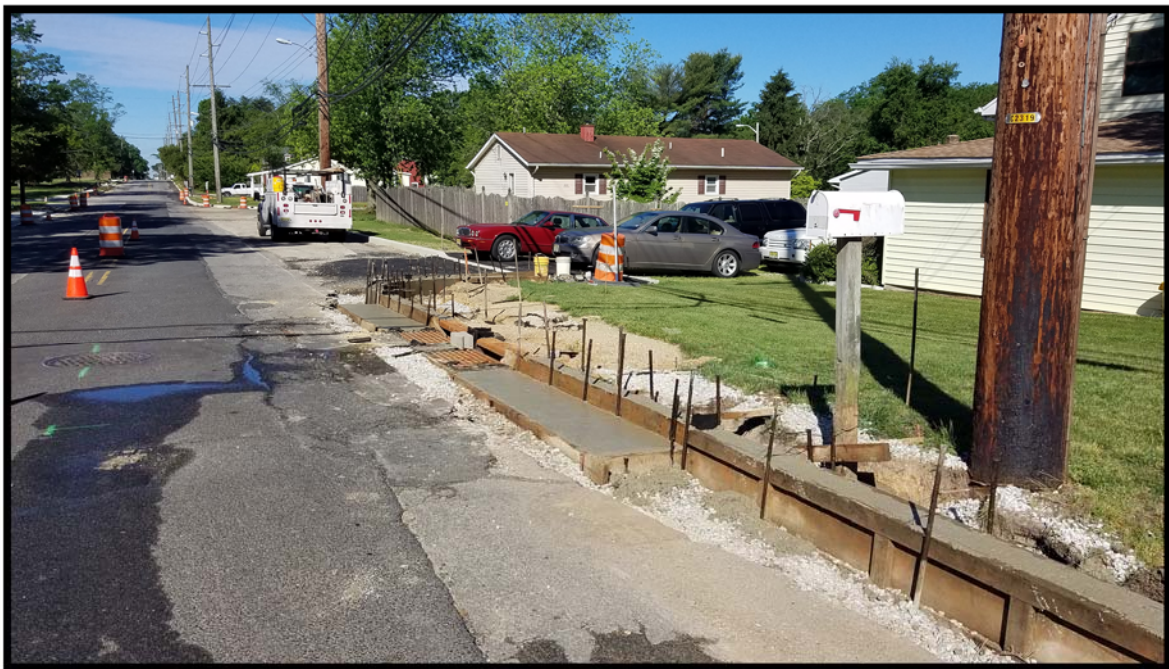
Photograph 1 – Concrete vertical curb and monolithic gutter installed at inlet D-41 near station 106+80L.
