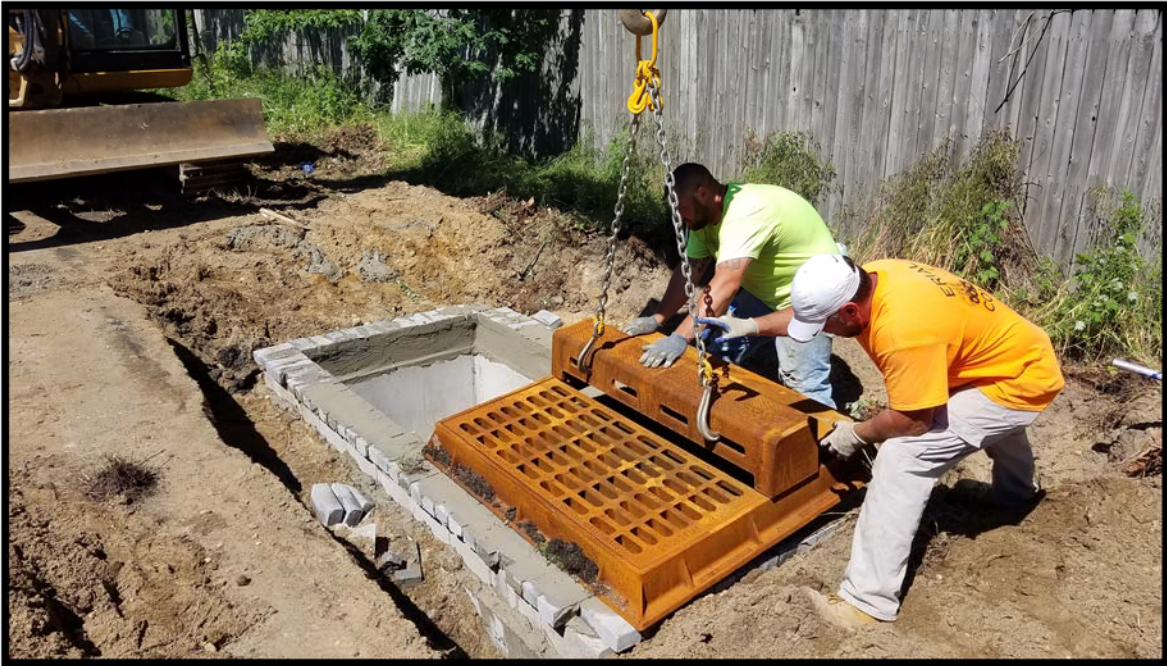
Photograph 6 – Castings for double 'B' inlet D58 being set in place.
