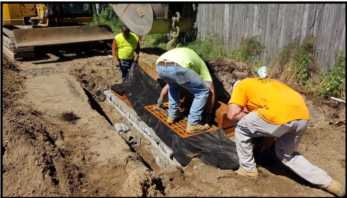
Photograph 7 – Castings for double 'B' inlet D58 set in place with inlet filter fabric being installed for soil erosion protection.
