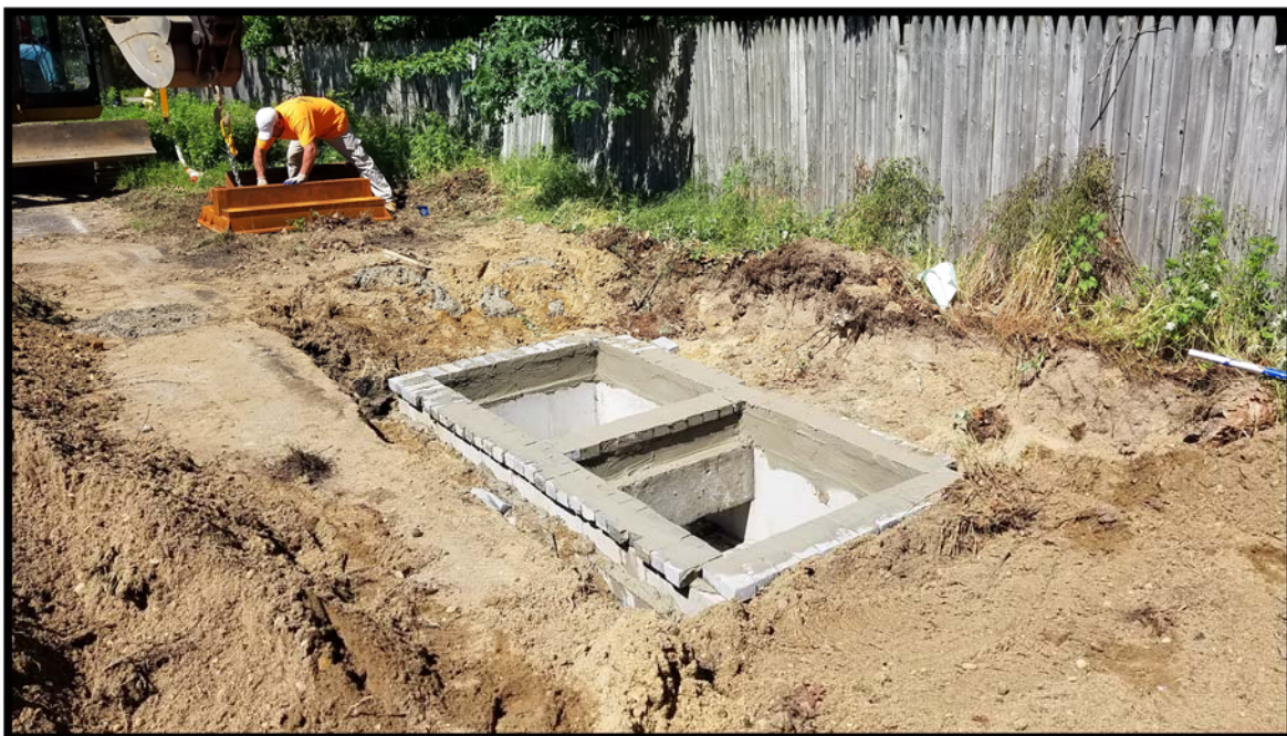
Photograph 5 – Precast double 'B' inlet D58 set in place and mortar and solid brick spacer blocks installed.
