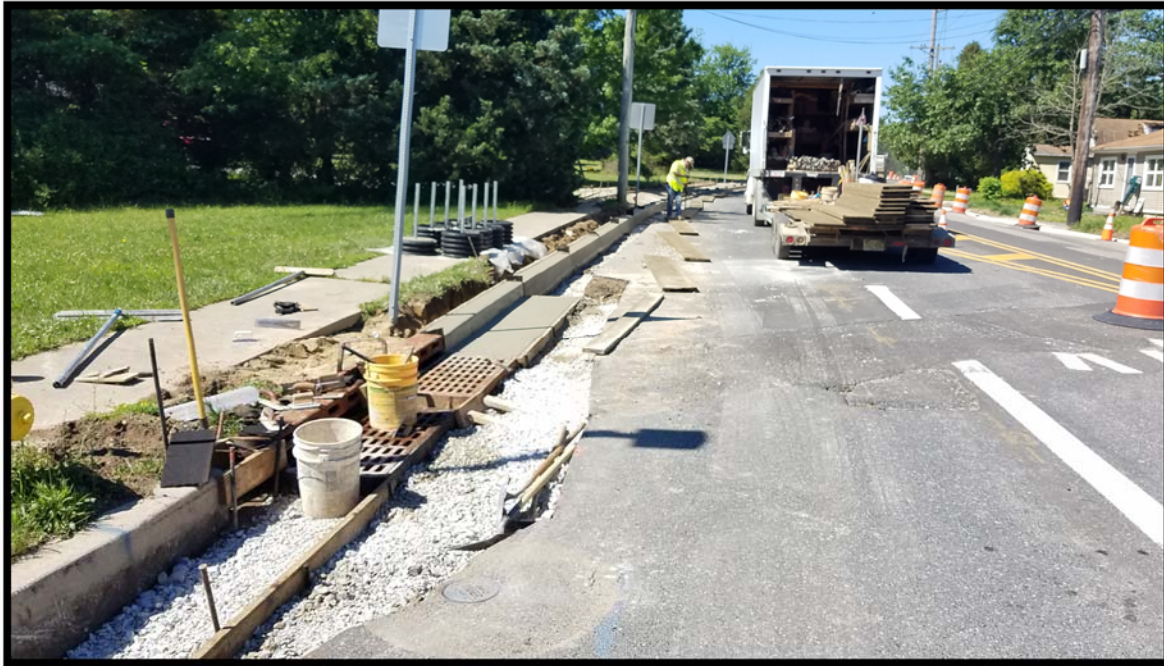
Photograph 4 – Curb and monolithic gutter installed adjacent to inlet D-43 near station 113+00R. Preparing for concrete gutter pour adjacent to existing curb that is slated to remain.
