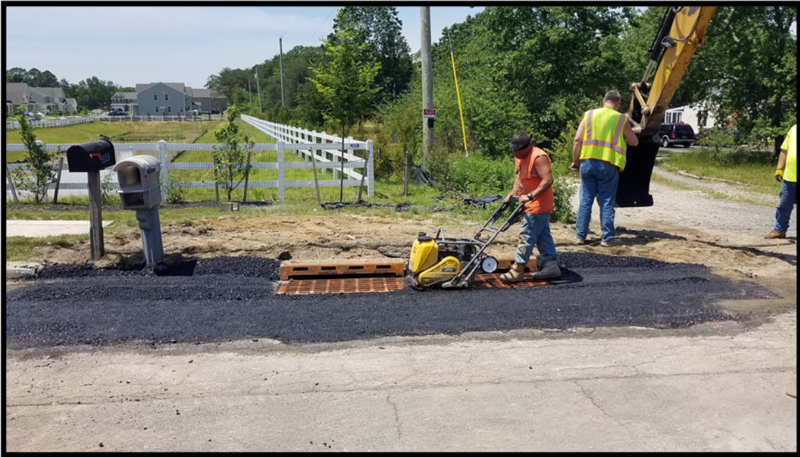
Photograph 10 – Asphalt restoration being installed at Double B inlet D-48 near station 117+25L.
