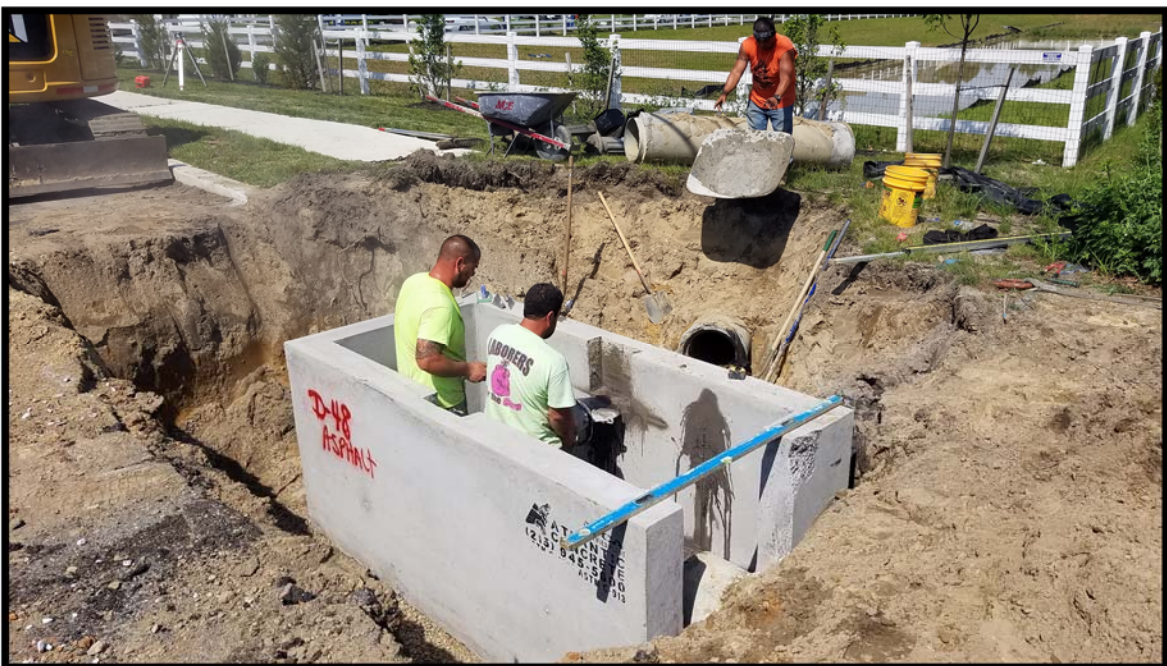
Photograph 9 – Double B inlet D-48 being set near station 117+25L.
