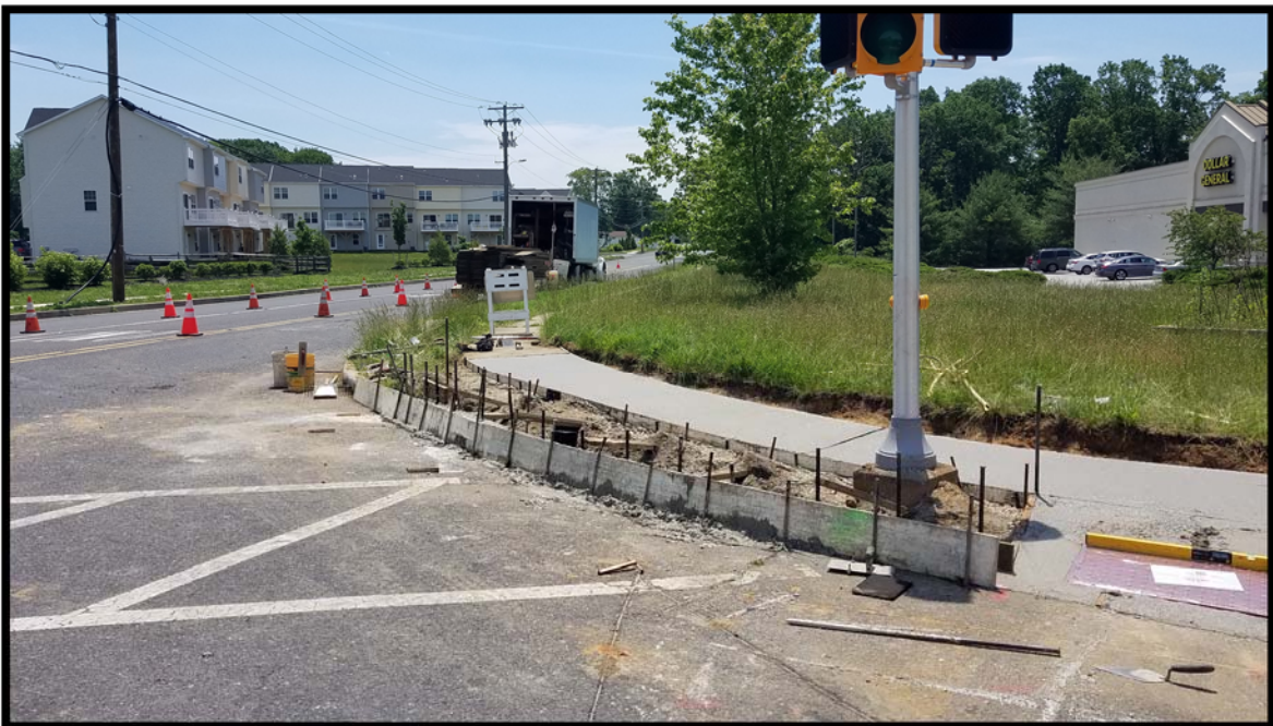
Photograph 11 – Curb, sidewalk and handicapped accessible ramp being installed at southeast corner of Erial-Williamstown Road intersection.
