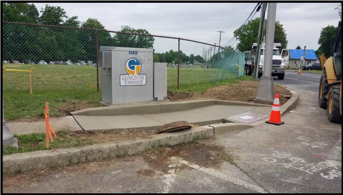
Photograph 4 – Curb, handicapped accessible ramp and header curb installed at the northwest corner of the Erial-Williamstown Road intersection.
