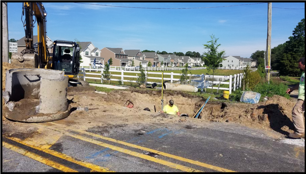
Photograph 8 – Existing manhole removed for installation of double B inlet D-48 near station 117+25L.
