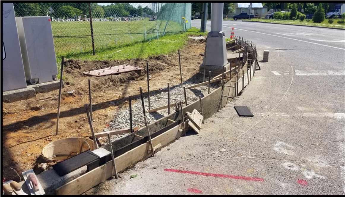
Photograph 2 – Forms installed for installation of curb and handicapped ramp depression at the northwest corner of the Erial-Williamstown Road intersection.
