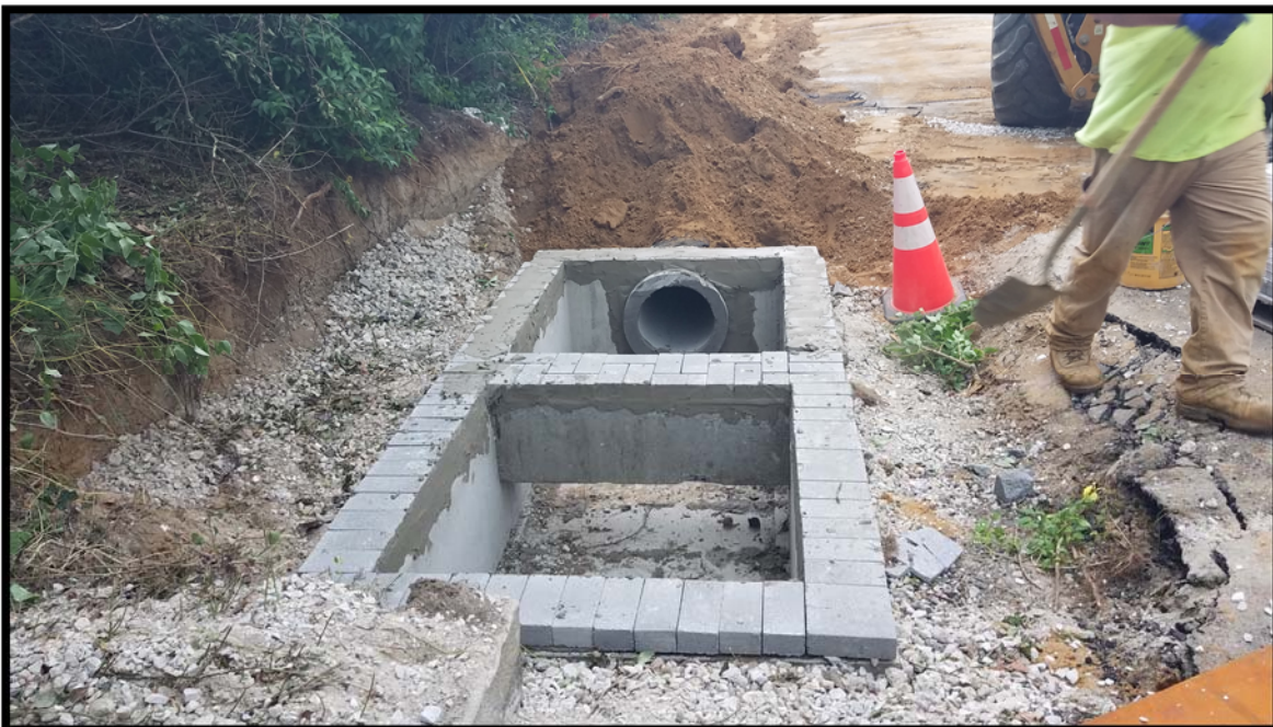
Photograph 7 – Inlet D57 installed near station 125+75R with 15" RCP and mortar and brick spacer blocks installed
