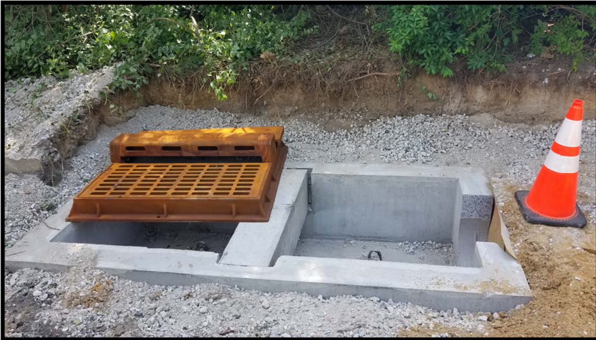
Photograph 6 – Inlet D57 installed near station 125+75R .
