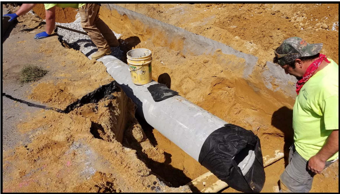
Photograph 5 – 15" Reinforced Concrete Pipe being installed in the vicinity of station 123+50 heading north towards inlet D57.
