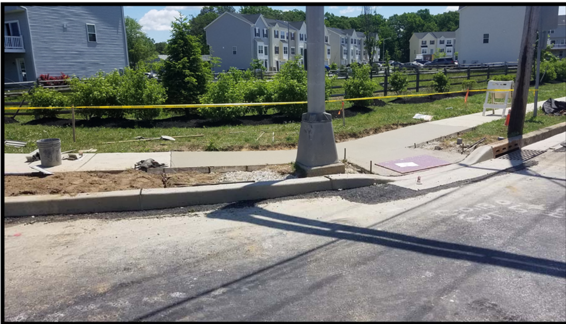
Photograph 3 – Sidewalk and handicapped accessible ramp installed at the northeast corner of the Erial-Williamstown Road intersection.
