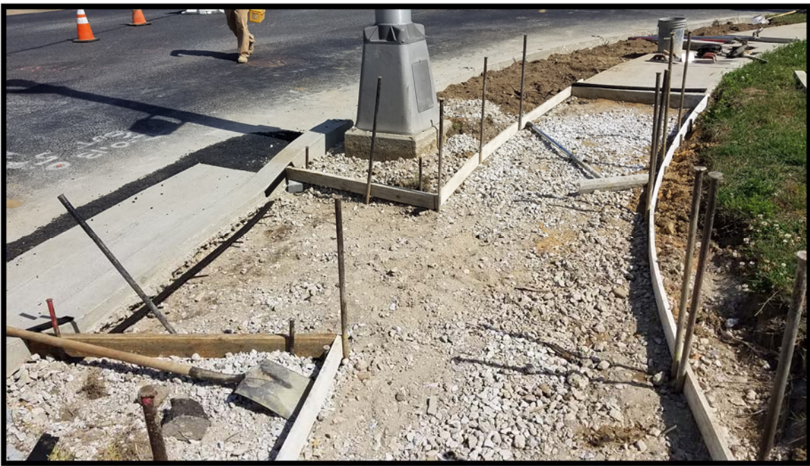
Photograph 1 – Forms installed for installation of sidewalk and handicapped accessible ramp at the northeast corner of the Erial-Williamstown Road intersection.
