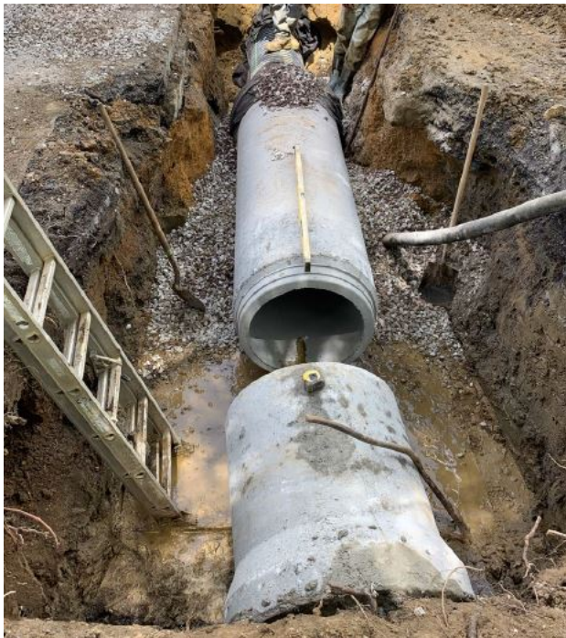
Figure 2: RCP installation
