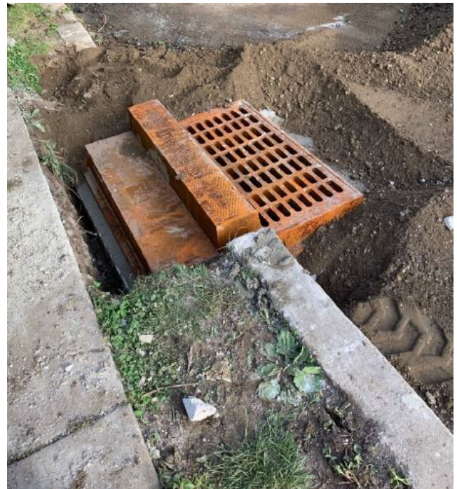
Figure 3: Type B inlet installed
