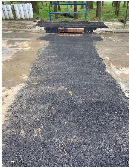
Figure 1: Stormsewer crossing roadway restoration
