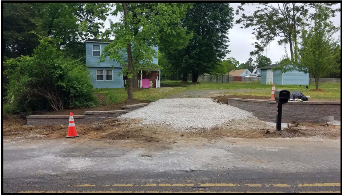
Photograph 6 – Minor field adjustment to extend Segmental Retaining Wall at north side of driveway return near station 109+50 to accommodate driveway grades and proposed sidewalk at driveway apron.
