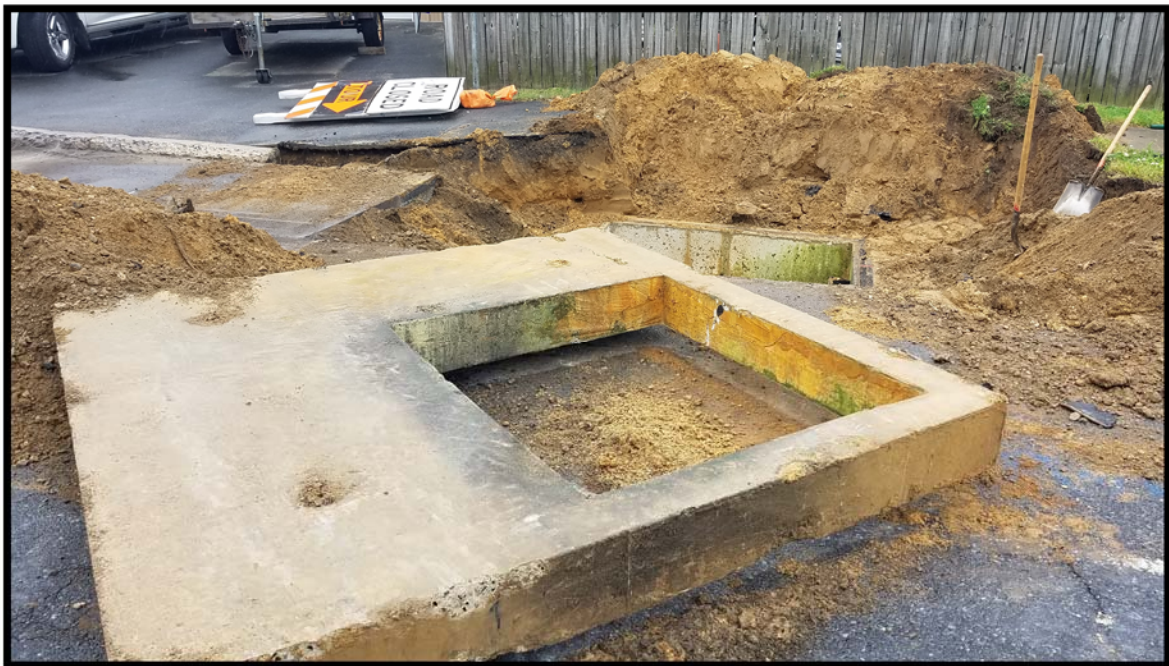
Photograph 7 – Existing inlet D-56 disassembled prior to retrofitting to “E” inlet.
