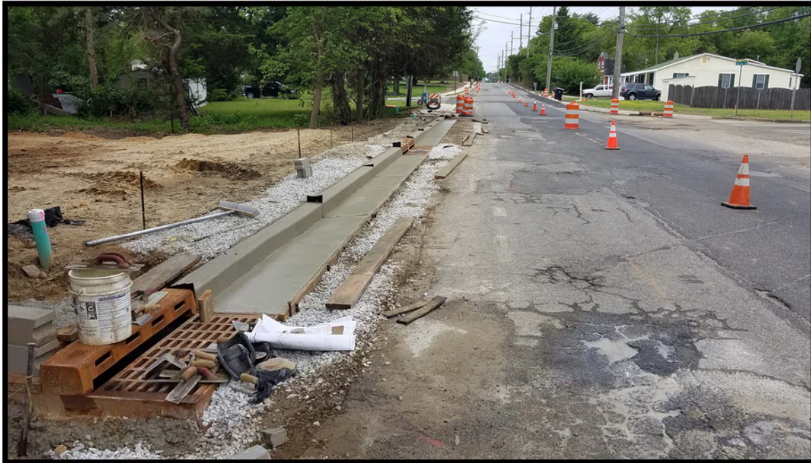
Photograph 2 – Concrete monolithic curb/gutter installed from Station 104+50R to 105+50R.
