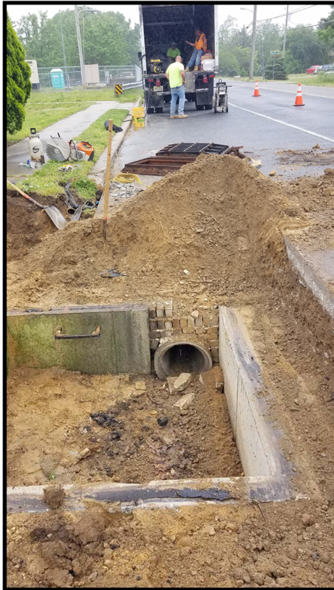
Photograph 8 - Existing inlet D-56 before modification to "E" Inlet.
