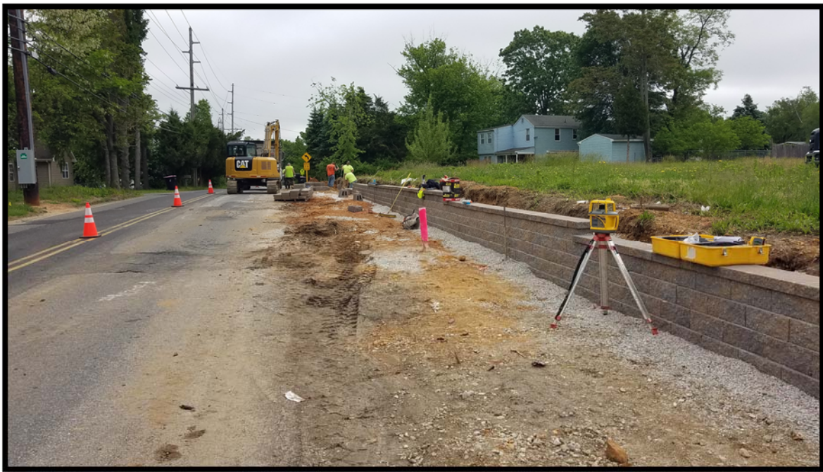
Photograph 1 – Segmental Retaining Wall being installed at widened roadway approaching station 109+50.
