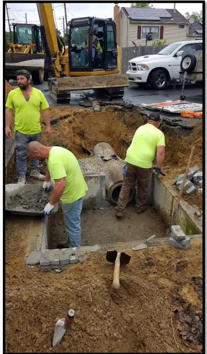
Photograph 9 – Additional Reinforced Concrete Pipe being installed at inlet D-56 before modification to "E" Inlet.
