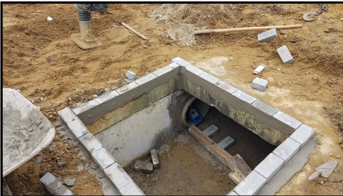
Photograph 11 – Top Slab of inlet D-56 installed and brick and mortar leveling course installed prior to setting of new casting. Note: Inlet work still ongoing and casting to be installed next week.
