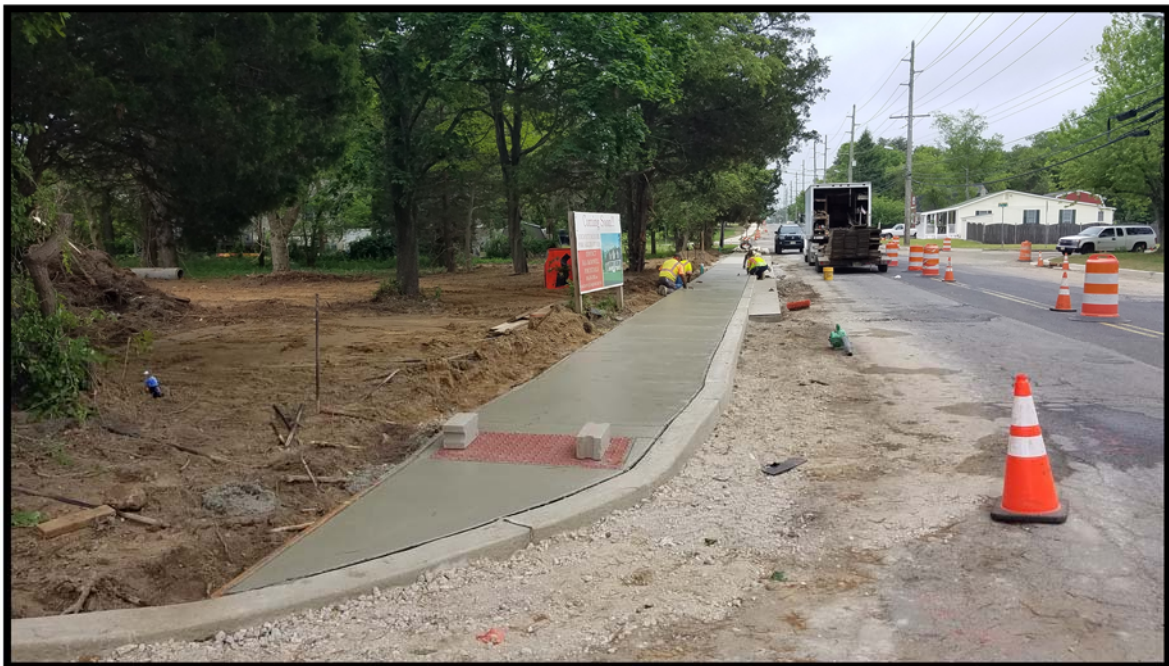
Photograph 5 – Concrete sidewalk and curb ramp R23 installed near station 106+50R
