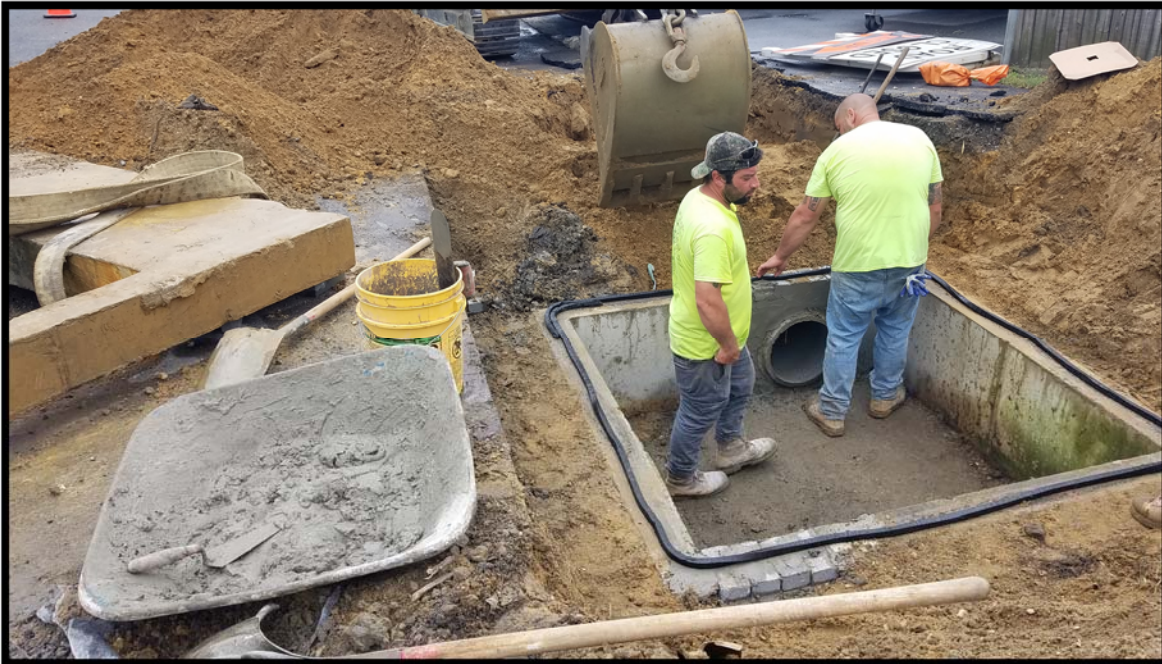
Photograph 10 – Butyl Tape installed on inlet D-56 before installing reinforced concrete top slab.
