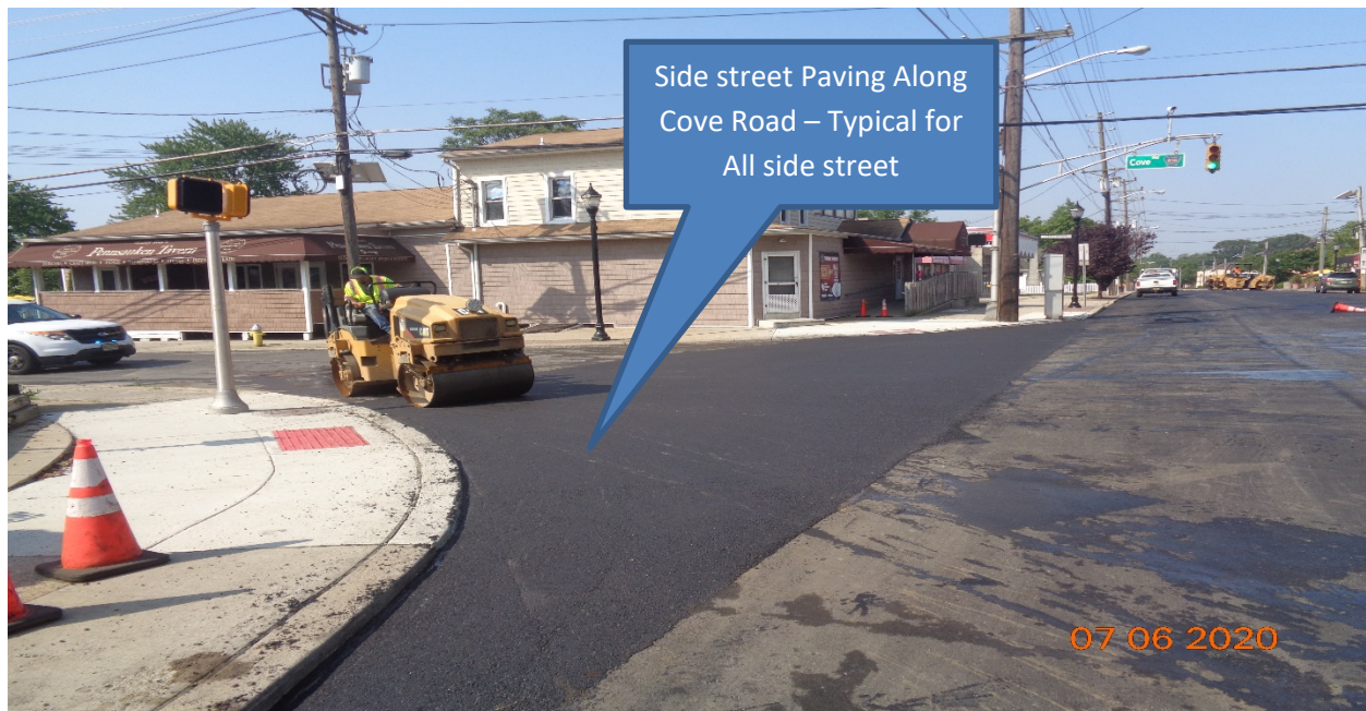
Figure 2: Hot Mix Asphalt 9.5M Surface course was place at all side street along Westfield Avenue from Lexington Avenue – Sherman Avenue, LT, and RT.
