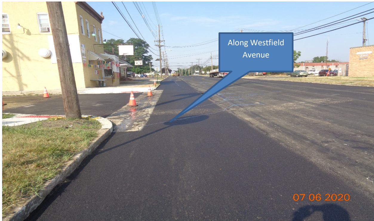
Figure 1: Hot Mix Asphalt 9.5 M surface Course was placed along Westfield Avenue from Sherman Avenue STA 109+50 – Tinsman Avenue 64+00
