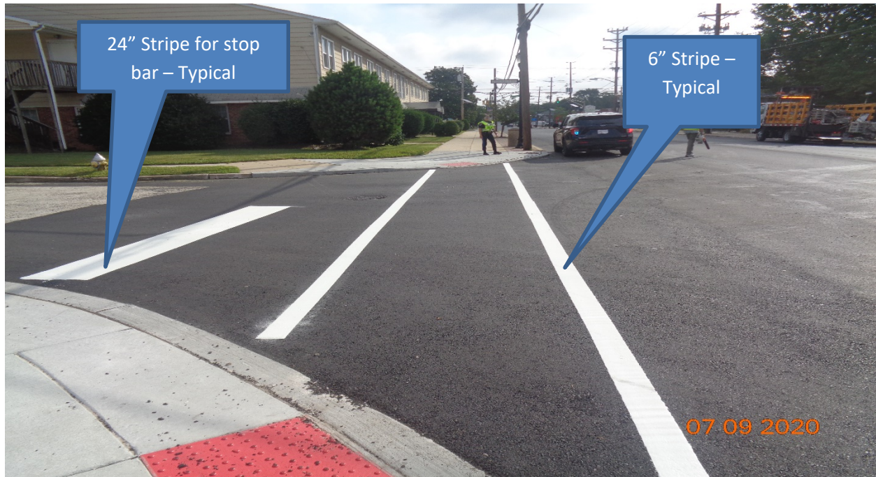
Figure 11: Thermoplastic striping along side streets from Lexington Avenue to Sherman Avenue, RT, and LT
