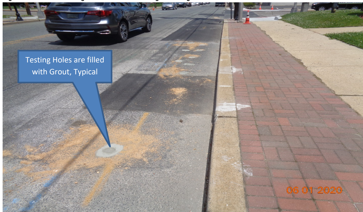
Figure 2: Gas Leak testing holes were filled with grout along Westfield Avenue at Merchantville Avenue.
