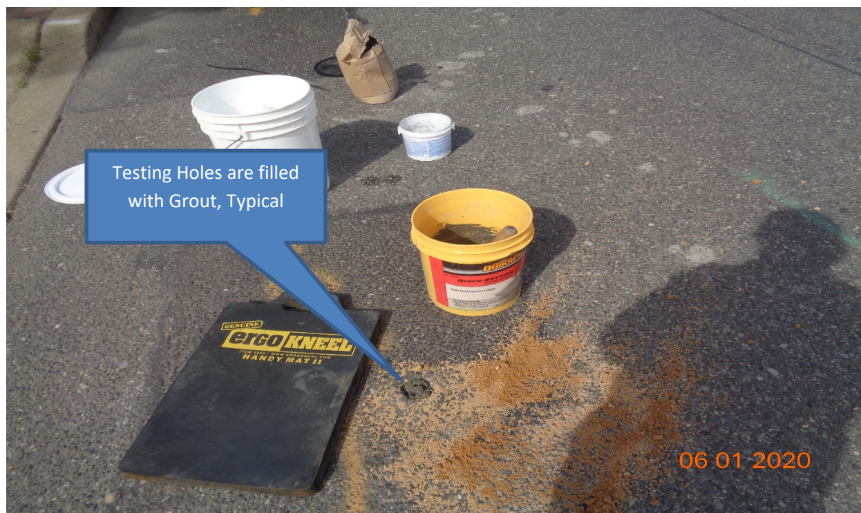
Figure 1: Gas Leak testing holes were filled with grout along Westfield Avenue at Merchantville Avenue.
