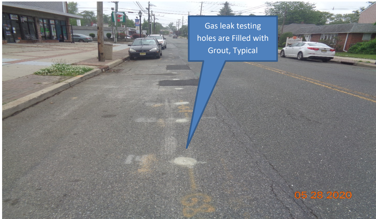
Figure 1: Gas Leak testing holes were filled with grout along Westfield Avenue at Hillcrest Avenue.
