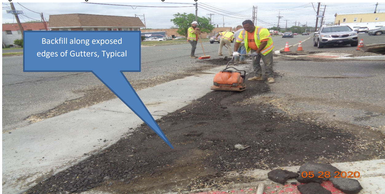
Figure 2: Exposed edges of concrete gutters were filled with DGA Along Westfield Avenue, RT, at Sherman Avenue, Bethel Avenue, and Clement Avenue, Typical
