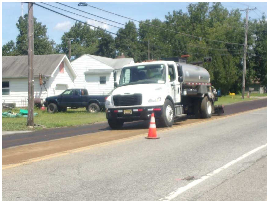
Figure 5 Full depth reclamation of the Left side of Pennington Ave. Sta. 15+00 to 27+80.
