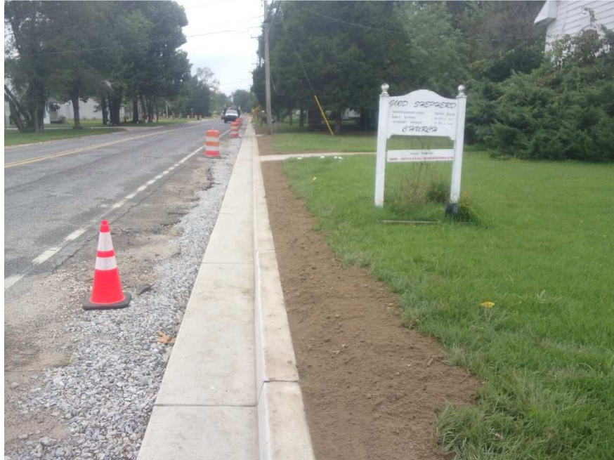
Figure 4 Typical turf repair behind curb and gutters along Pennington Avenue.
