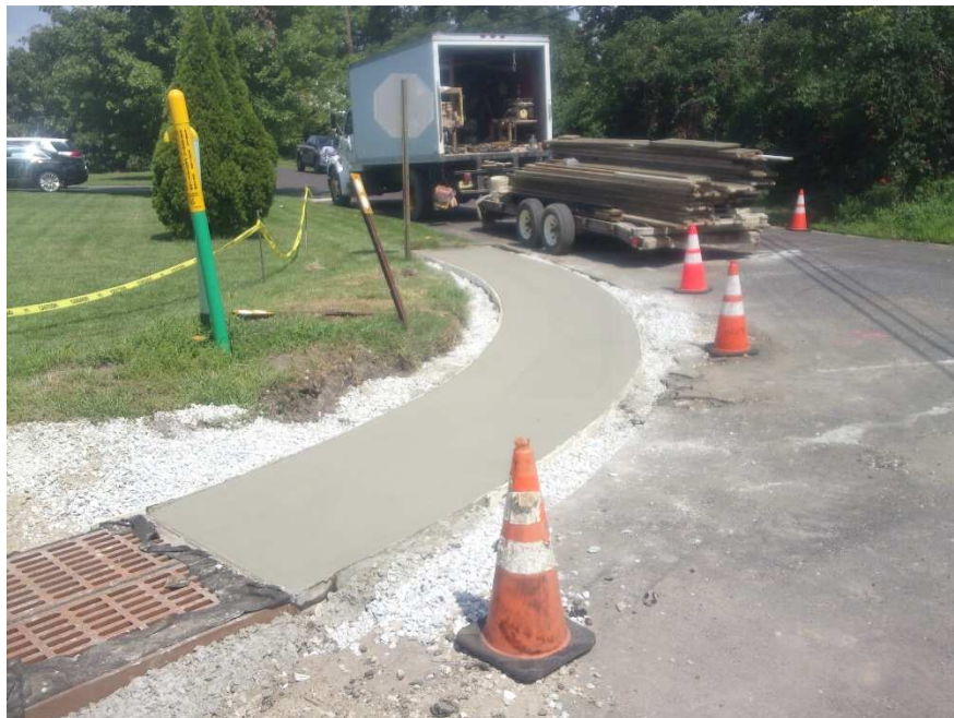
Figure 4 Concrete gutter install Northwest corner of Atlantic and Pennington Ave.
