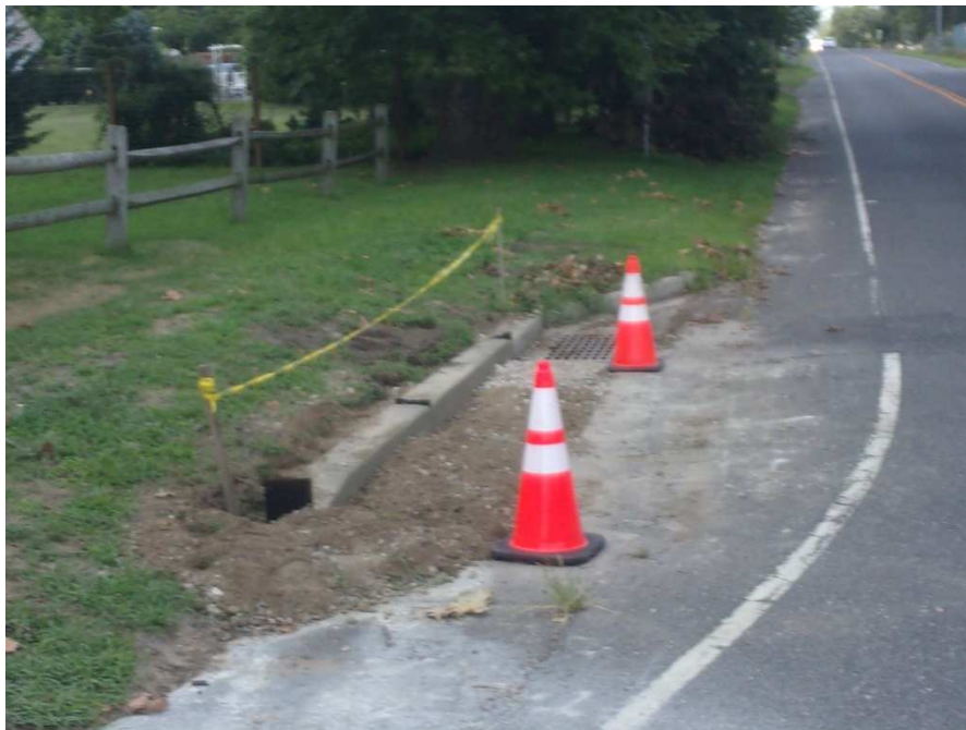
Figure 3 Installed concrete curb "A" inlet South bound side Old White Horse Pike.
