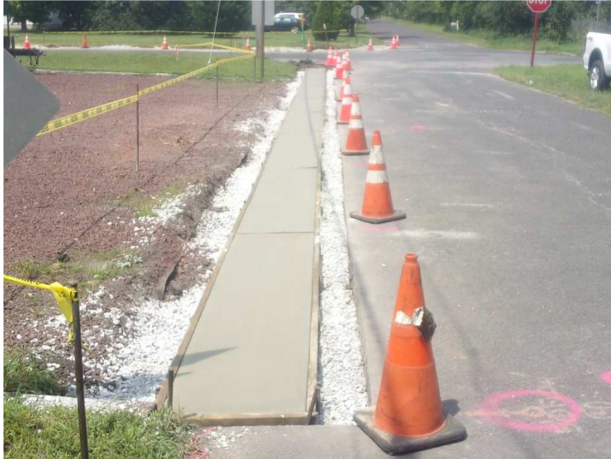
Figure 5 Concrete Gutter installed along West side of Atlantic Ave.
