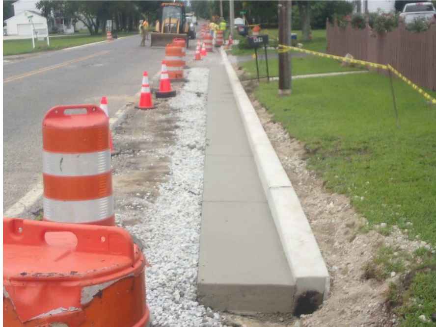
Figure 7 Concrete Gutter and Monolithic Curb and gutter installed Sta. 21+73 to 23+00 left Pennington Ave.
