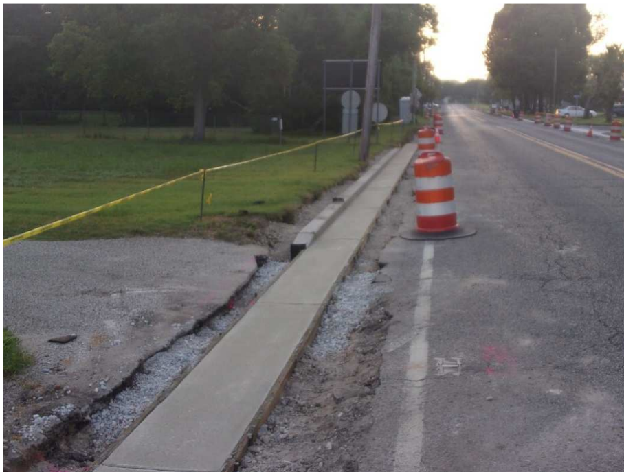
Figure 5 Concrete Gutter and Monolithic Curb and gutter installed Sta. 14+00 to 15+43 left Pennington Ave.
