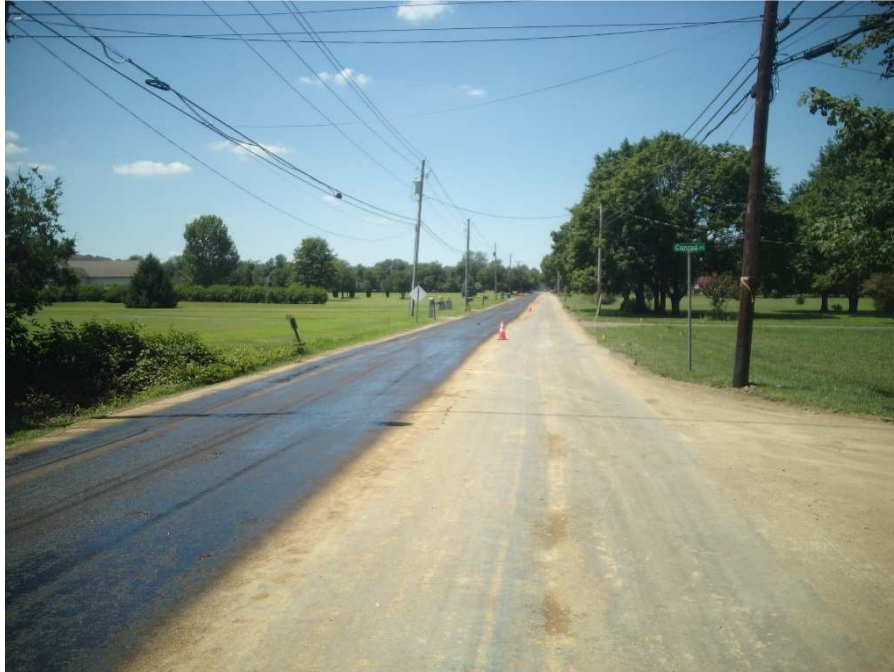
Figure 4 Full Depth Reclamation (FDR) along Chew Road
