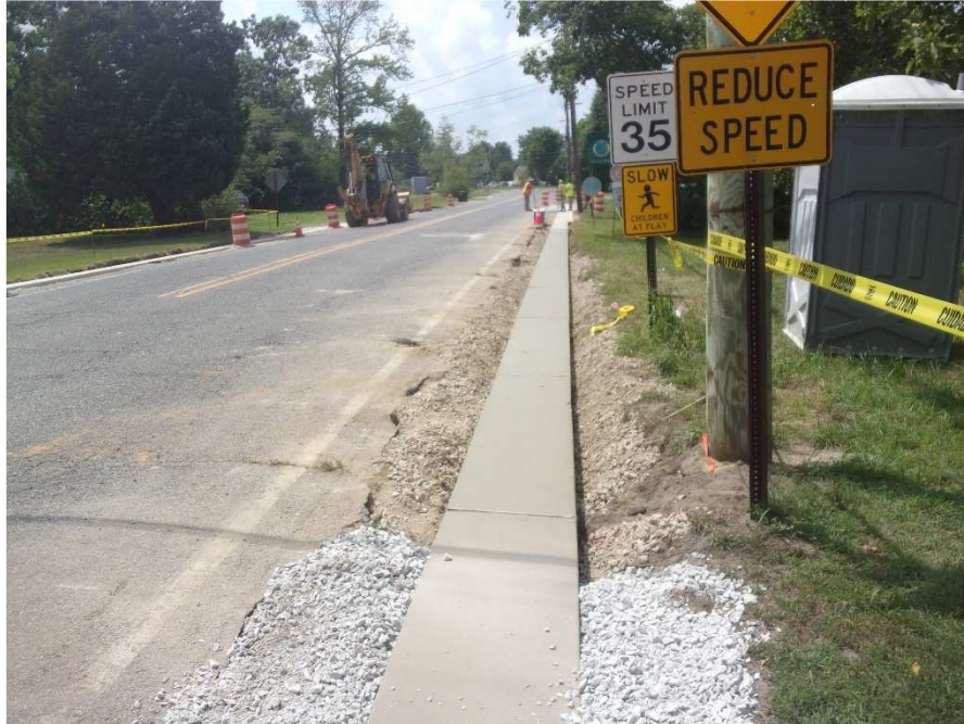
Figure 6 Concrete Gutter installed on Pennington Ave. Sta 15+47 to 16+95 left
