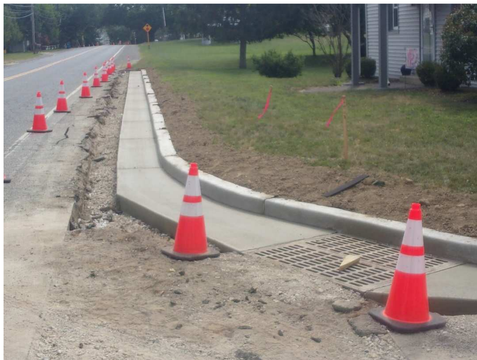
Figure 1 Concrete gutter installed Pennington Ave. right Station 23+00 to Oak St.
