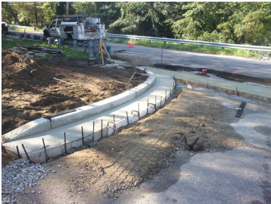
Figure 5 Concrete Gutter and Curb installed Northeast Corner Condo Ave. and Chew Rd.
