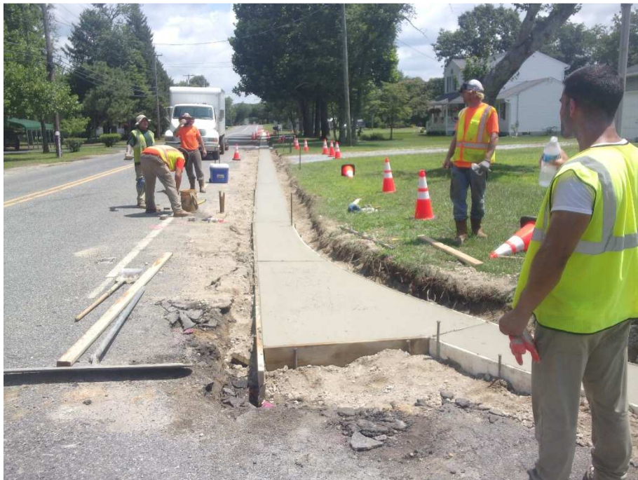
Figure 9 Concrete gutter installed Station 18+50 to Maple Ave. right side of Pennington Ave
