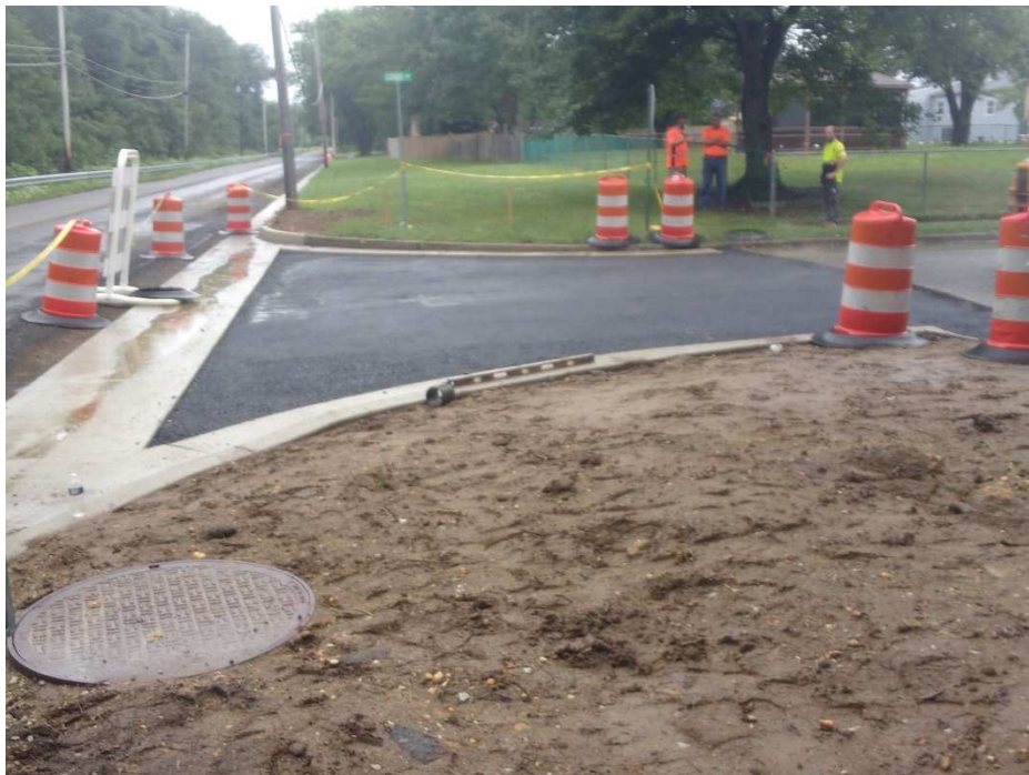
Figure 11 Base pave Condo Ave. behind gutter
