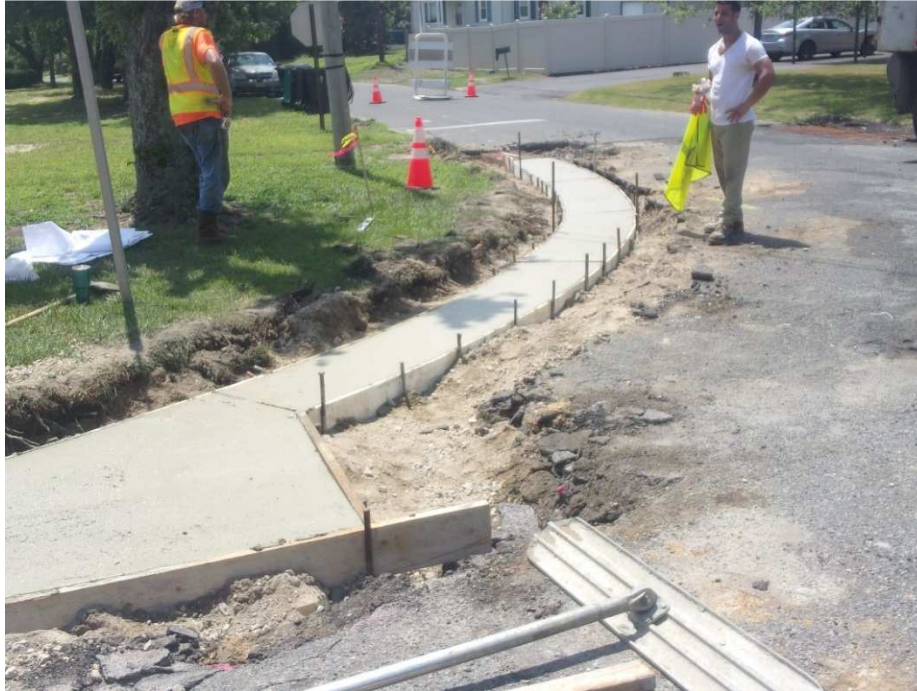
Figure 10 Concrete gutter installed Station Eastern corner of Maple Ave
