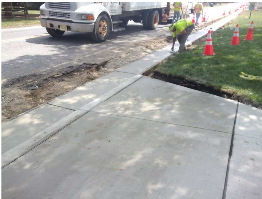
Figure 7 Concrete Gutter installed on Pennington Ave. sta 19+60 to 18+45
