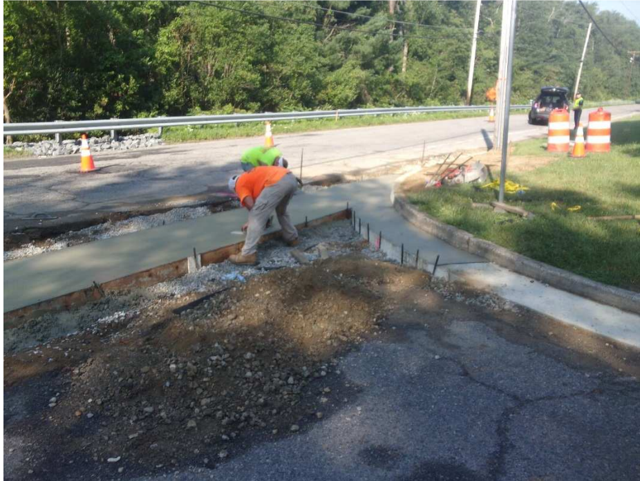
Figure 6 Concrete Gutter and Curb installed Northwest Corner Condo Ave. and Chew Rd.
