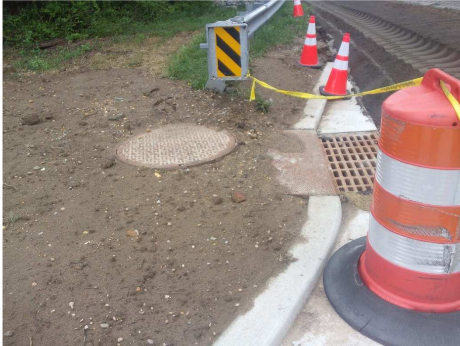
Figure 8 Set Square framed Manhole Casting Corner of Condo Ave. and Chew Road
