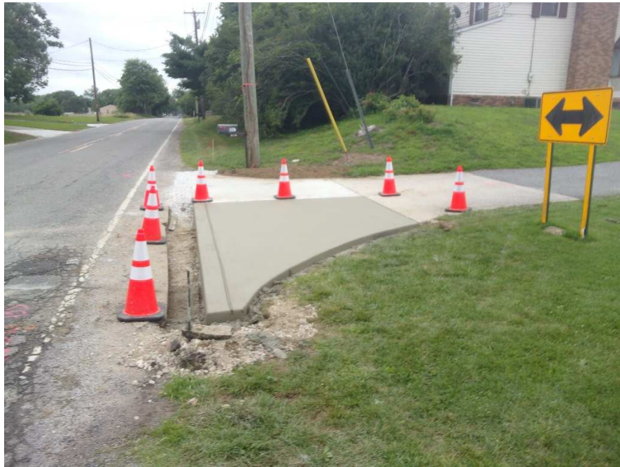
Figure 8 Second half of driveway apron installed at 1067 Chew Road
