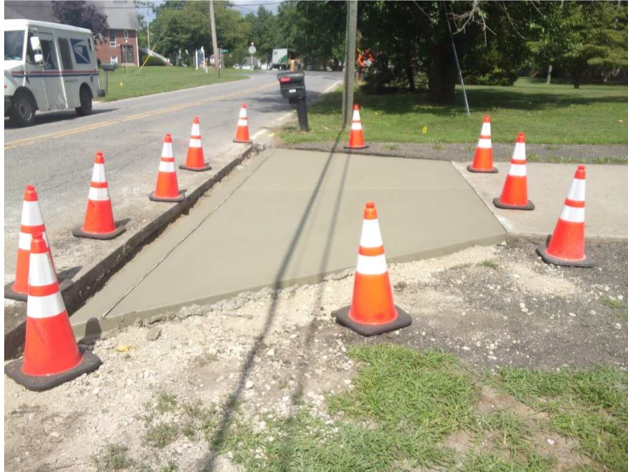
Figure 4 Driveway apron installed 1006 Chew Road
