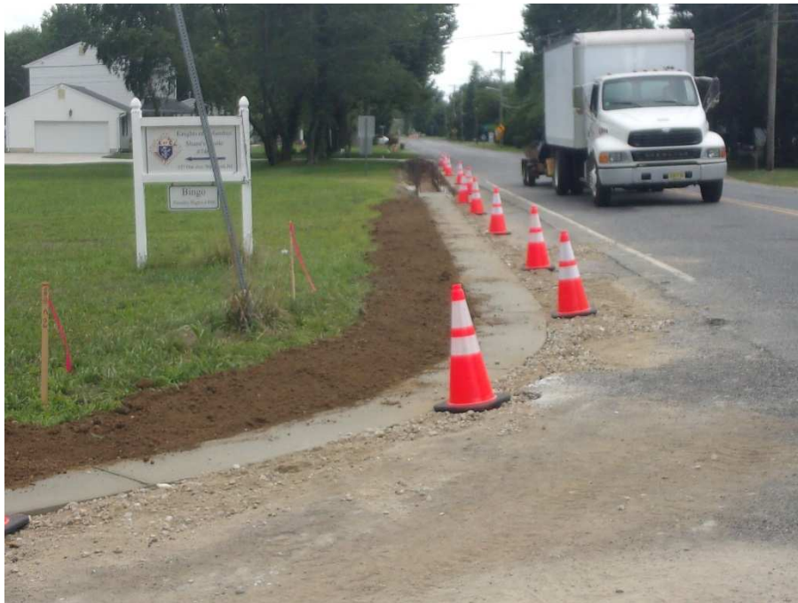
Figure 9 Concrete gutter installed Station 19+50 to Oak St. right side of Pennington Ave
