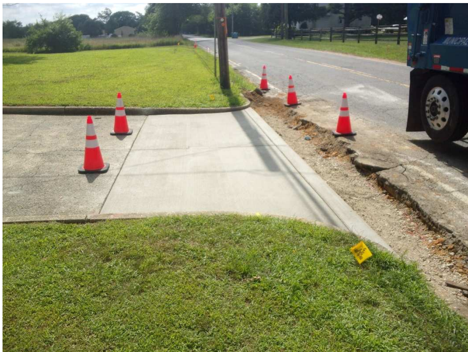
Figure 5 Driveway apron installed 1064 Chew Road Sta. 45+50
