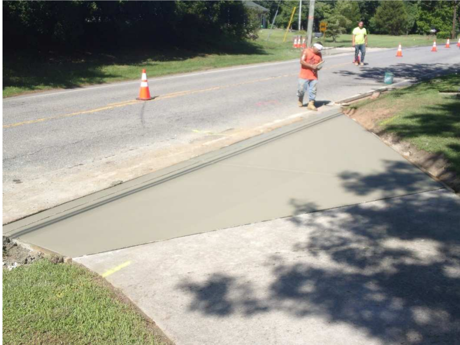
Figure 2 Driveway apron installed 1064 Chew Road Sta.44+75
