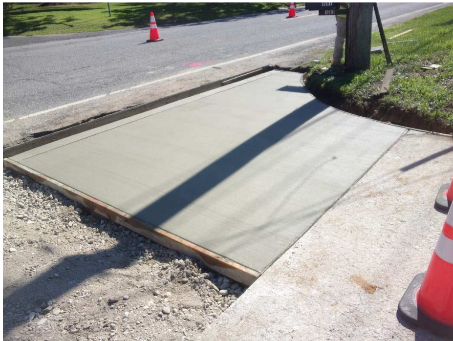
Figure 3 Driveway apron half installed to allow access 1067 Chew Road
