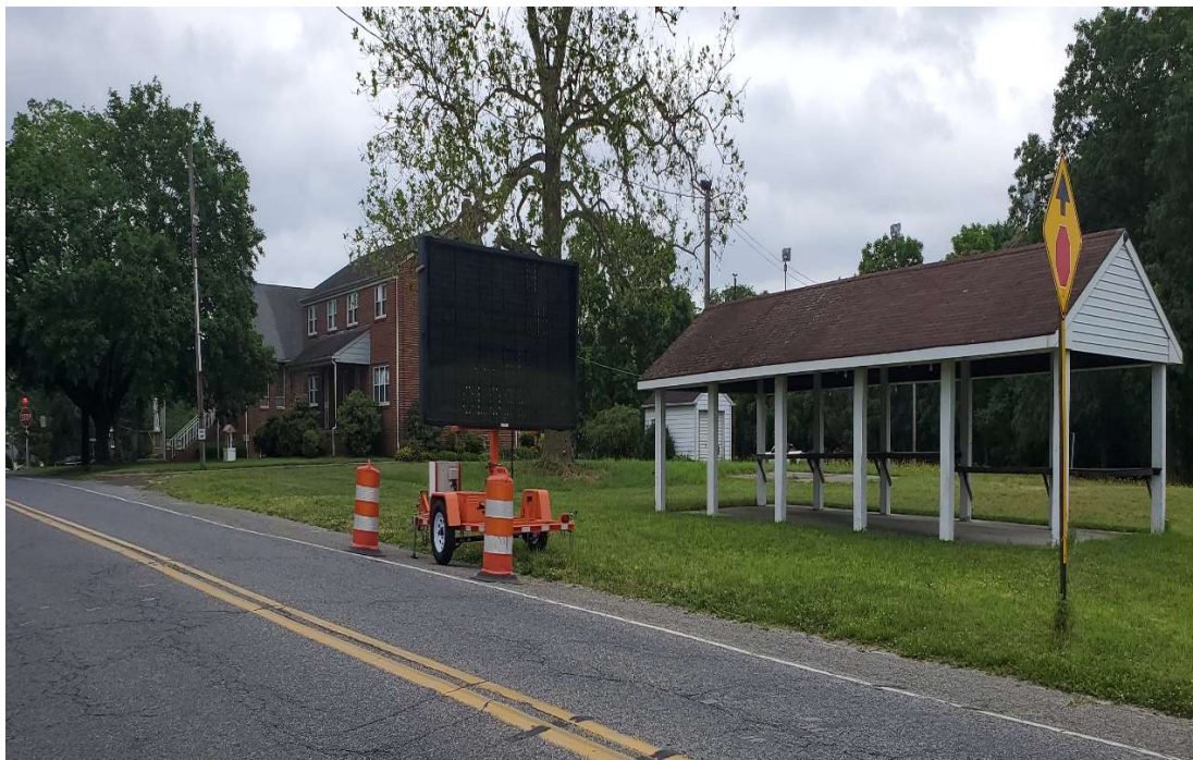
Figure 1 VMS installed at each end of the project warning motorist of Project Start
