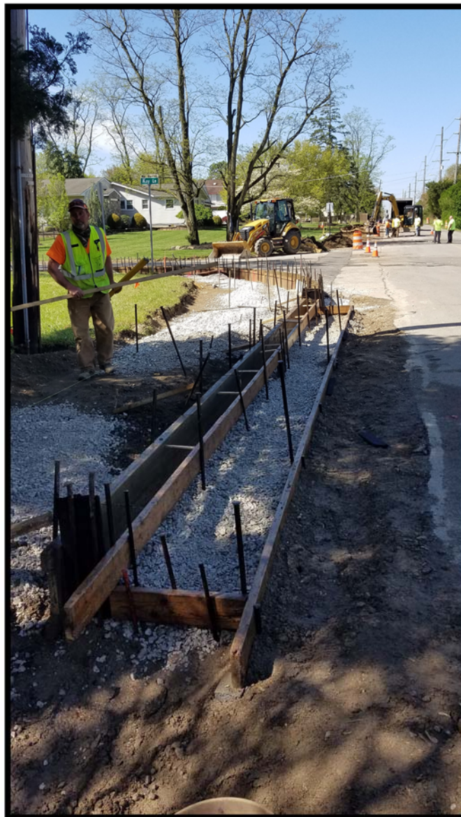
Photograph 1 – Monolithic curb and gutter formed out on Jarvis Road near Kay Lane.
