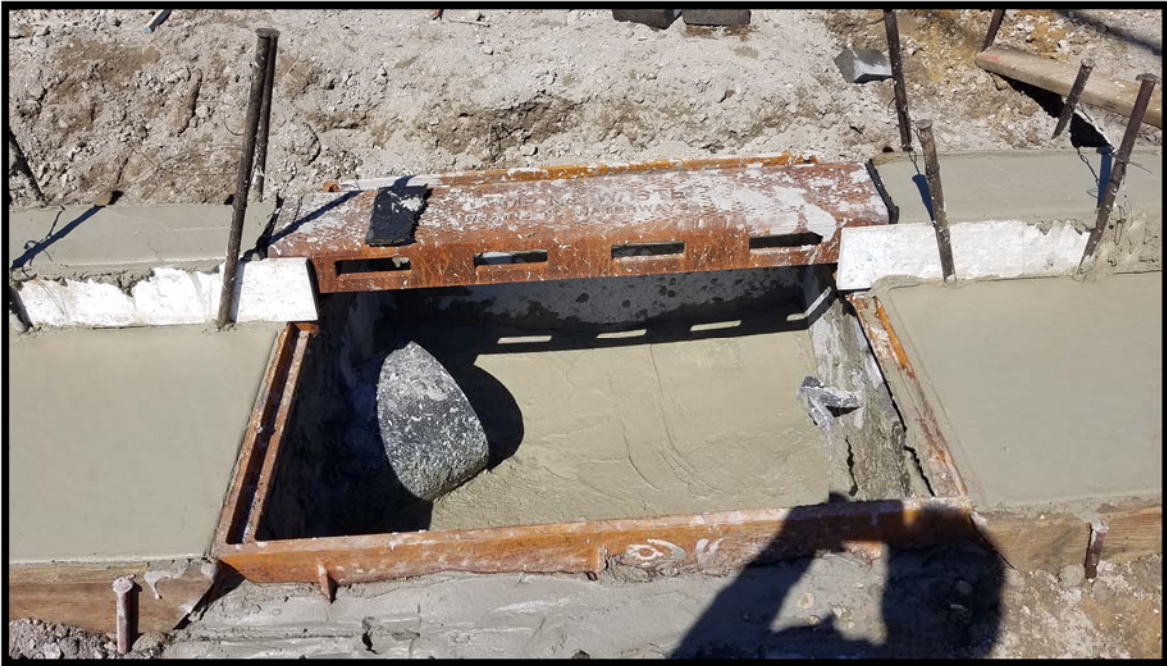
Photograph 8 – Concrete bench and concrete curb and gutter poured at 'B' Inlet installed at the New Brooklyn Road intersection per approved RFI #5-Revised.
