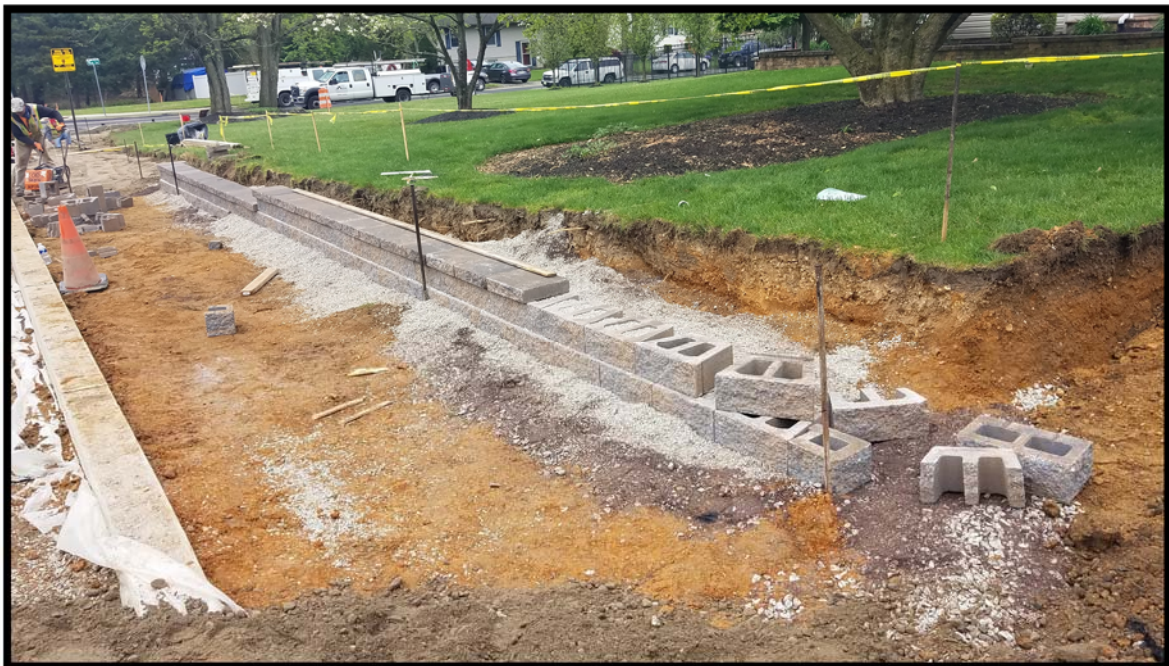
Photograph 7 – Segmental retaining wall being installed near Lynn Drive.
