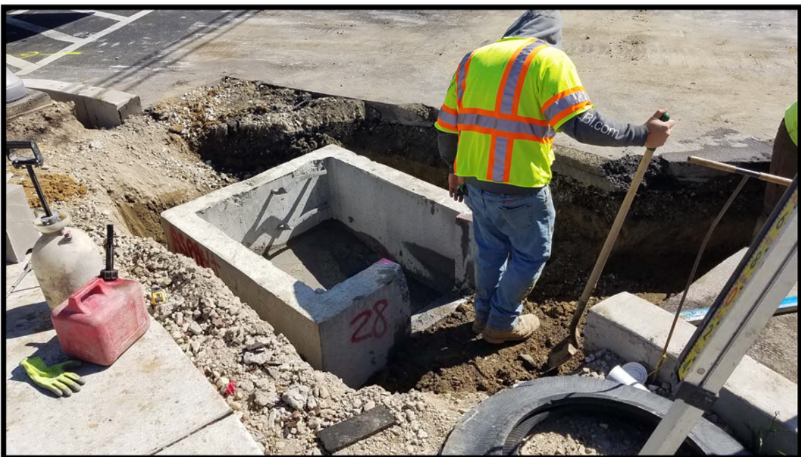
Photograph 3 – Inlet being set at the New Brooklyn Road intersection per approved RFI #5-Revised.
