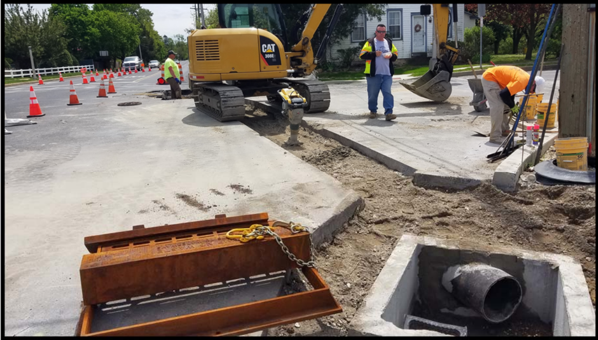
Photograph 4 – Inlet and 14" Ductile Iron Pipe being installed at the New Brooklyn Road intersection per approved RFI #5-Revised.
