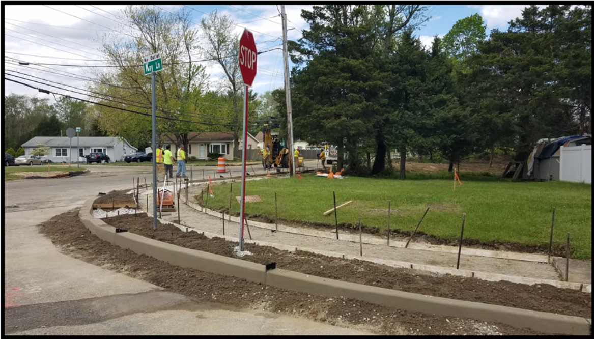
Photograph 2 – Curb forms stripped and trench backfilled with Dense Graded Aggregate, forms set and subgrade being prepared for sidewalk installation near Kay Lane.
