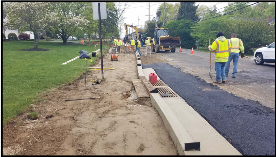
Photograph 6 – Inlet D-33 at Station 103+00 near Lynn Drive offset to avoid utility conflict. Preparation underway for sidewalk and segmental retaining wall installation.
