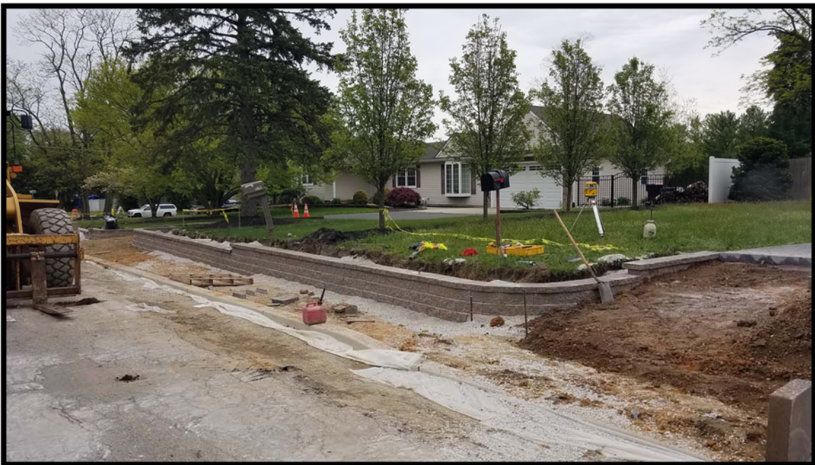
Photograph 9 – Segmental retaining wall being installed near Station 101+50R.
