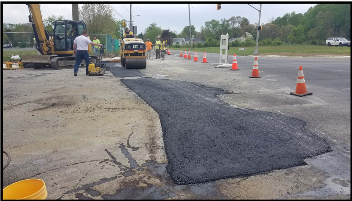
Photograph 5 – Road restoration for Inlet and 14" Ductile Iron Pipe installed at the New Brooklyn Road intersection per approved RFI #5-Revised.
