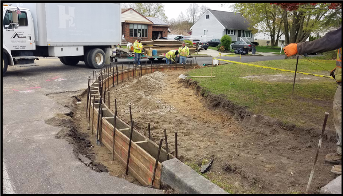
Photograph 2 - Concrete curb forms installed at the intersection of Jarvis Road and Sherri Lane.
