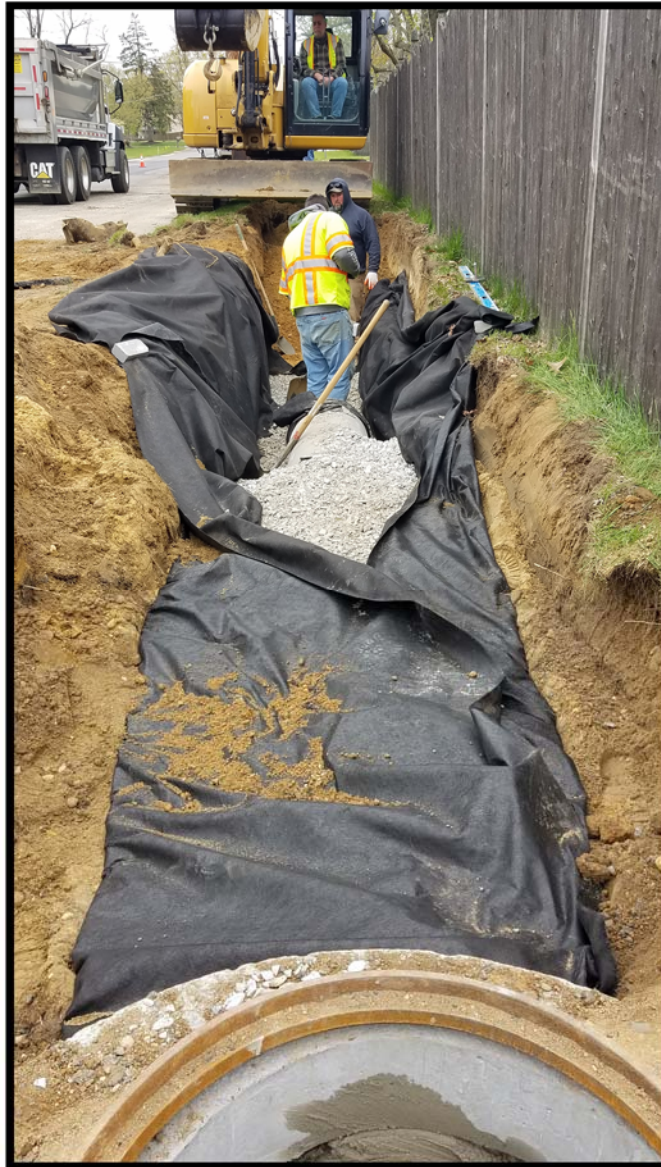
Photograph 1 – Perforated Reinforced Concrete Pipe and Stone Trench Drain being installed between Manholes D40 & D38.
