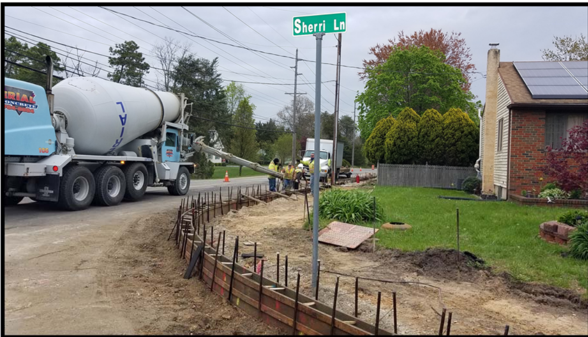
Photograph 5 – Concrete pour for curb at Sherri Lane.
