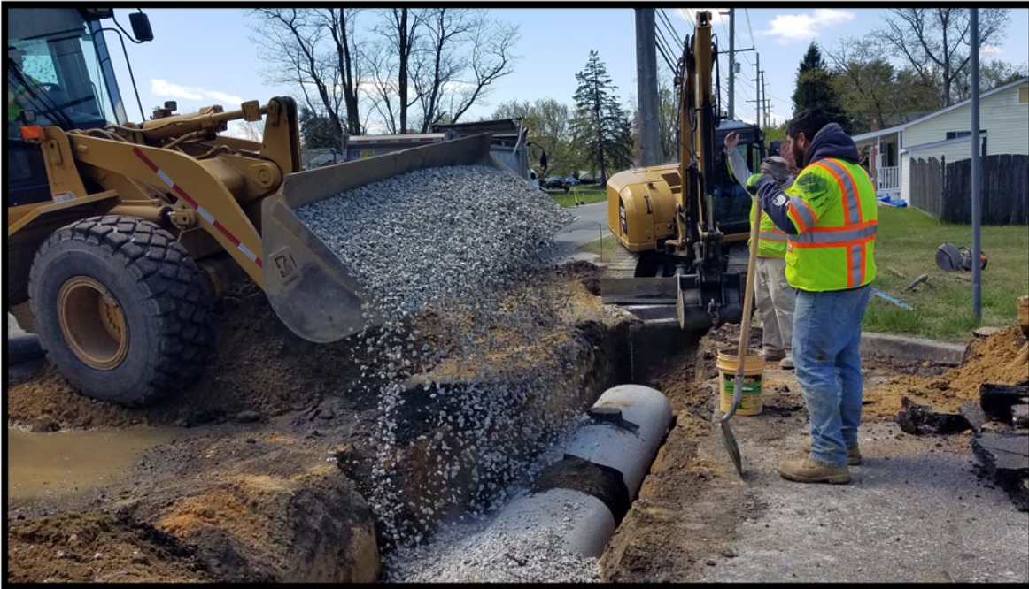
Photograph 4 – Horizontal Elliptical Reinforced Concrete Pipe being installed at Jarvis Court.
