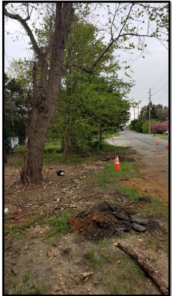
Photograph 7 – Tree and roots at station 105+06R in conflict with Double 'B' inlet D36 and corresponding piping.
