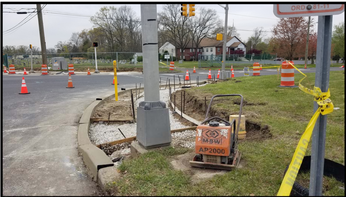
Photograph 3 – Curb poured and sidewalk forms and bedding prepared for concrete pour at the Jarvis Road and New Brooklyn-Erial Road intersection.
