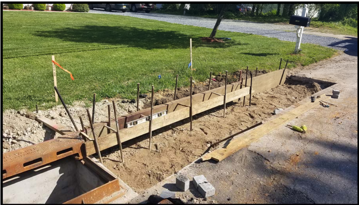
Photograph 5 – Curb forms being installed adjacent to Double “B” Inlet.
