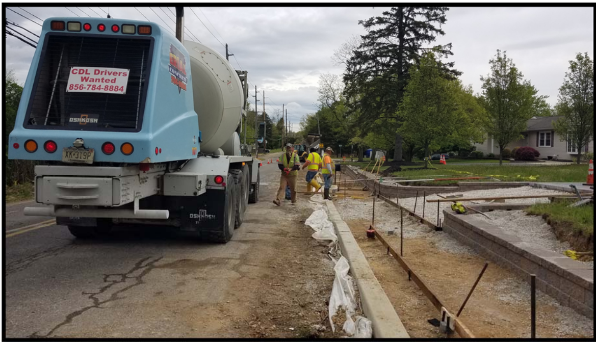
Photograph 1 – Preparing for concrete pour for sidewalk and driveway apron adjacent to completed Segmental Retaining Wall.
