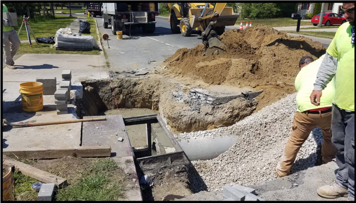
Photograph 8 – Modified “B” Inlet D-54 being converted to Double Modified “B” Inlet.
