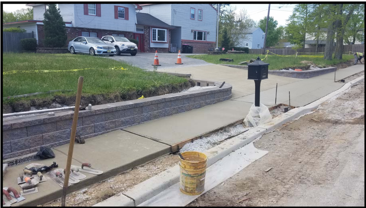
Photograph 3 – Completed curb, sidewalk and driveway apron adjacent to Segmental Retaining Wall.
