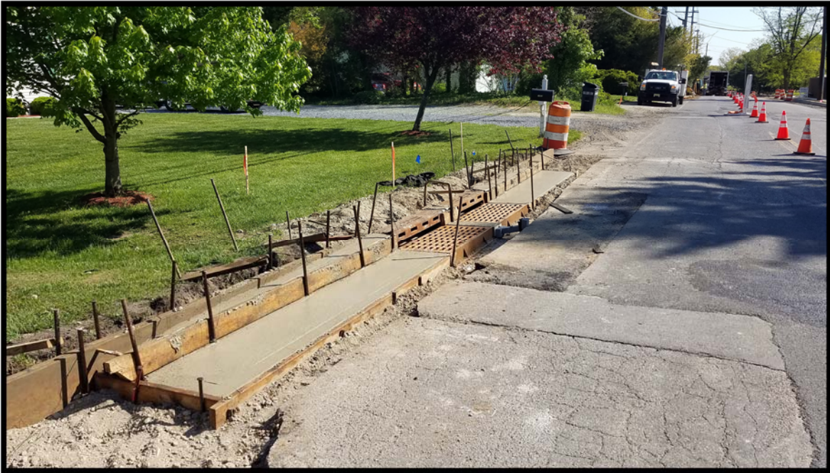
Photograph 6 – Monolithic Concrete Curb and Gutter installed adjacent to Double “B” Inlet.
