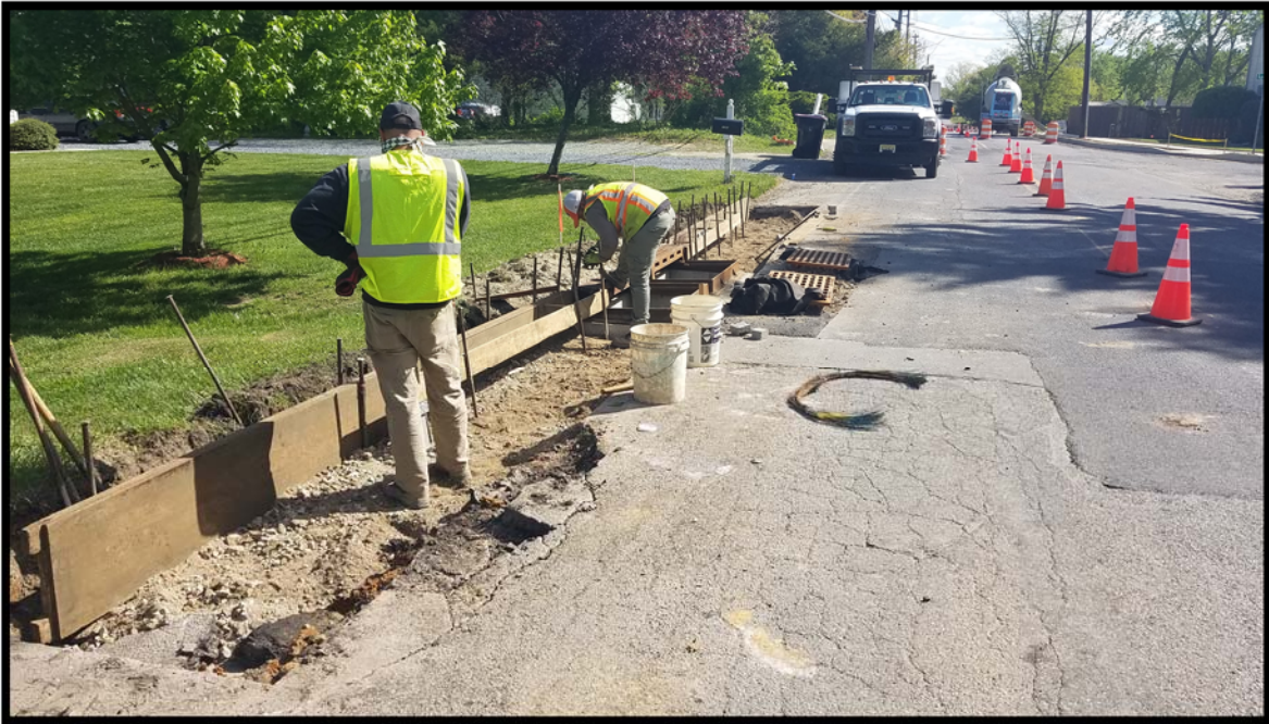
Photograph 4 – Curb forms being installed adjacent to Double “B” Inlet.
