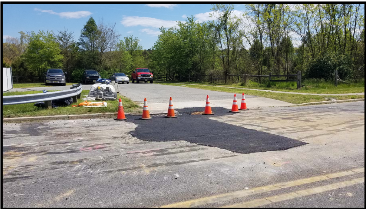
Photograph 9 – Asphalt restoration and temporary driveway restoration adjacent to Inlet D-54.
