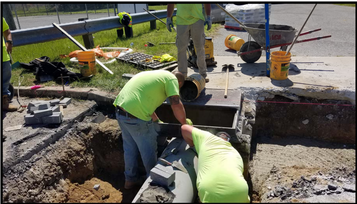
Photograph 7 – Modified “B” Inlet D-54 being converted to Double Modified “B” Inlet.
