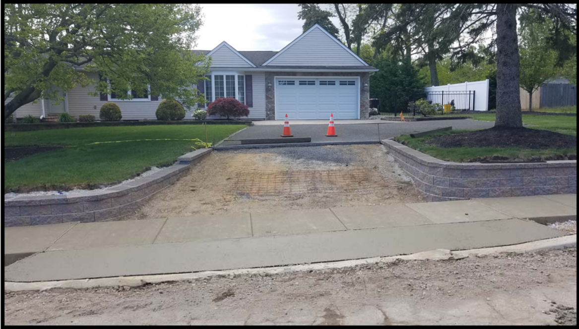
Photograph 2 – Preparing for concrete pour for driveway apron adjacent to completed Segmental Retaining Wall.
