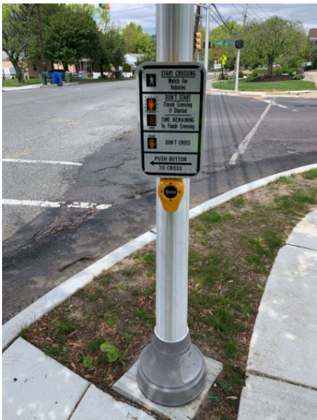
Figure 2: Push button installed
