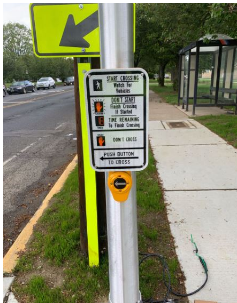
Figure 1: Push button installed
