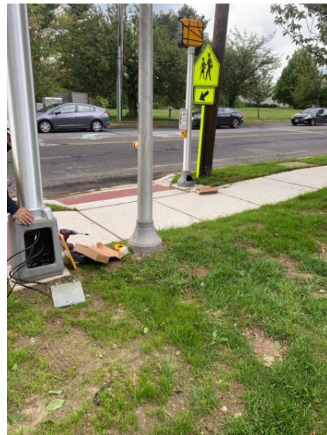
Figure 3: Preparation for installation of push button
