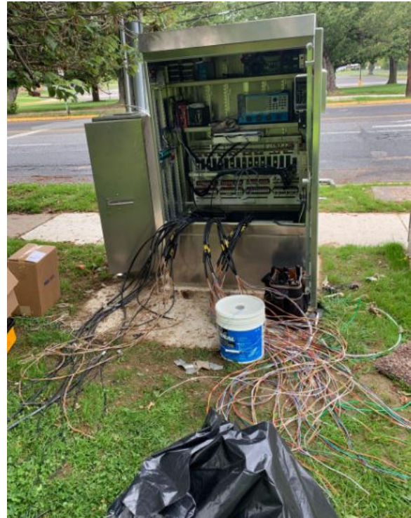
Figure 5: Securing traffic signal wires
