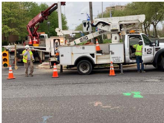
Figure 2: Diehl preparation to install traffic signal
