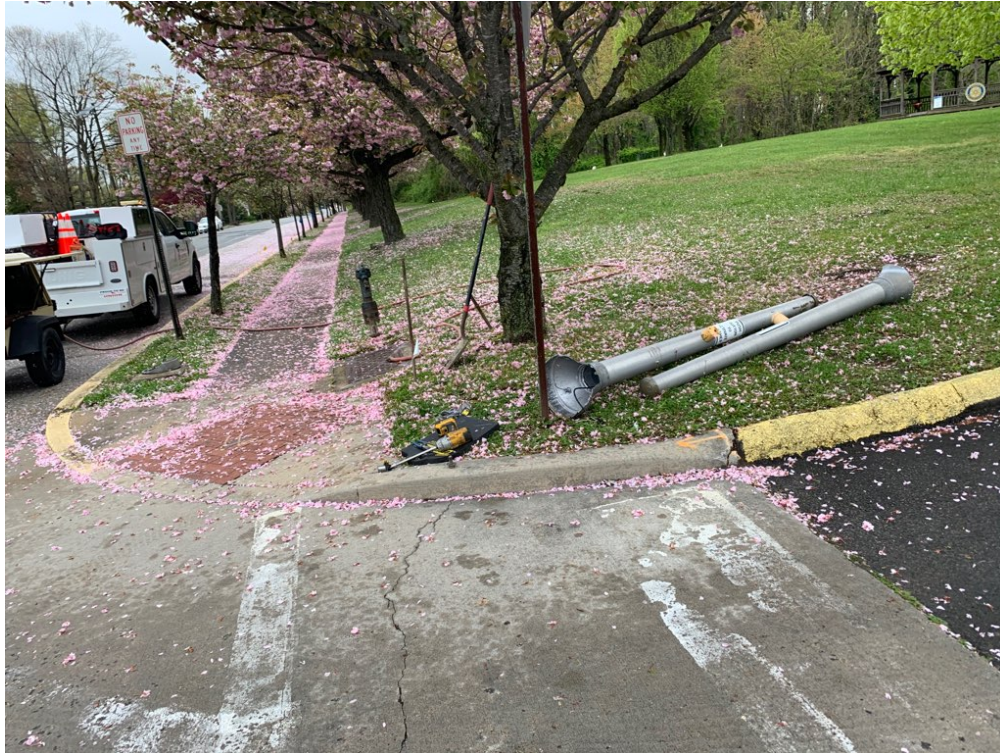
Figure 1: Pedestrian signal pole removal
