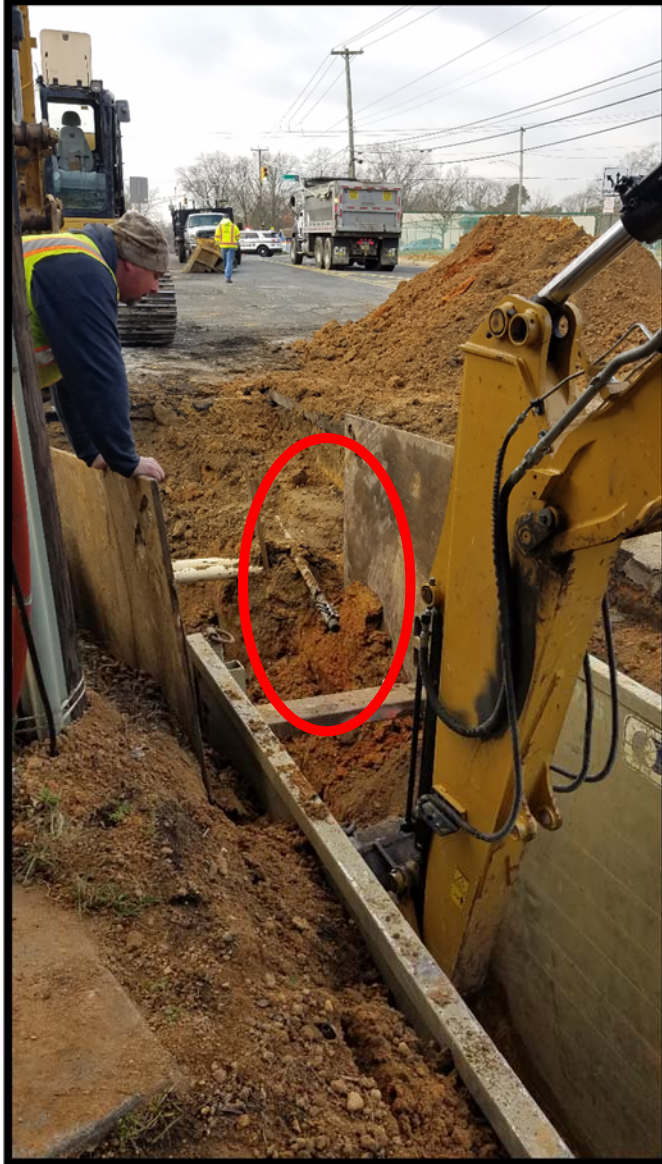
Trench box in place for installation of 18" Reinforced Concrete Pipe (RCP) between manholes D-12 and D-13 near STA 83+00. Note repair clamp installed on gas main stub by SJ Gas.
