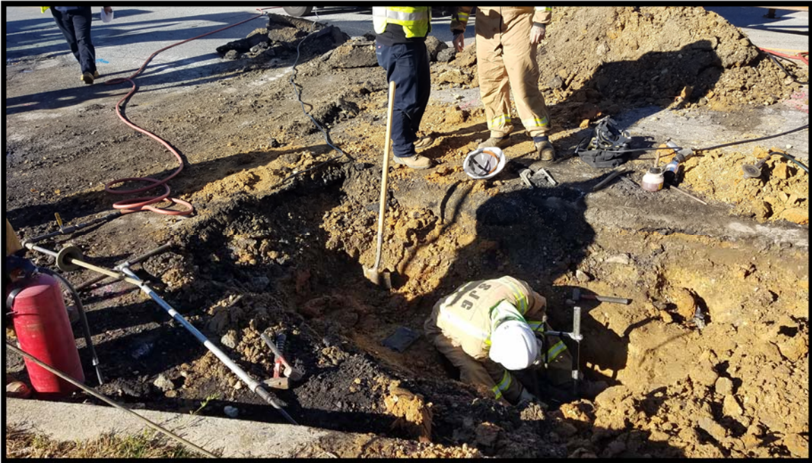
A damaged, unmarked gas main stub near STA 83+00 required repairs by South Jersey Gas representatives.
