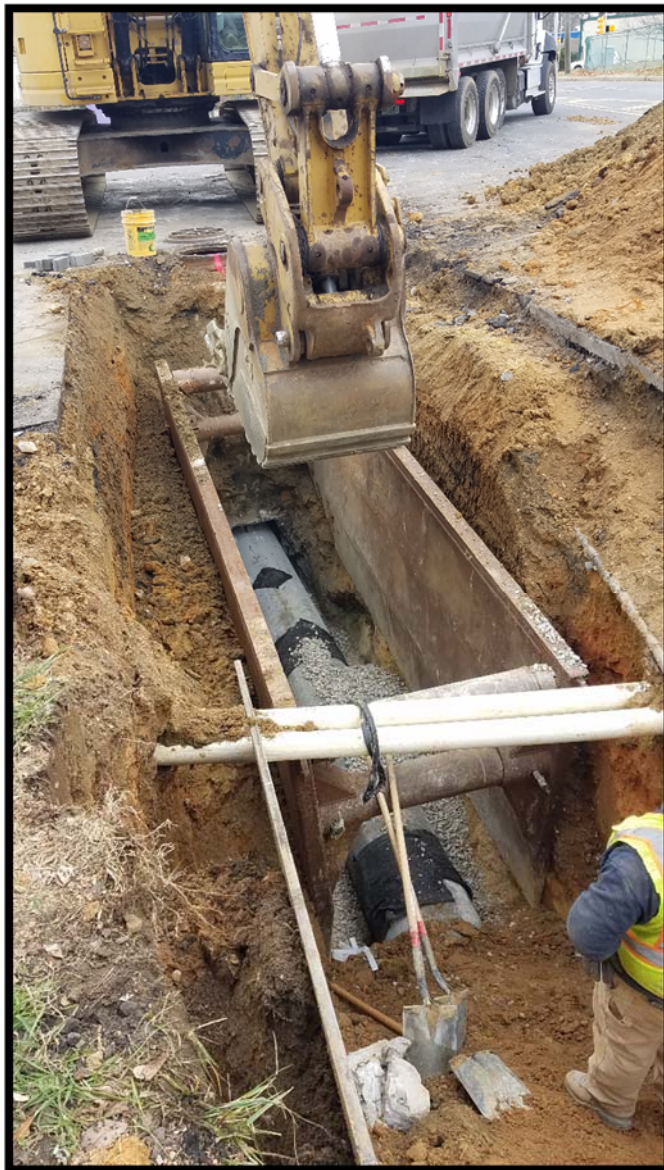
New 18" Reinforced Concrete Pipe (RCP) placed between manholes D-12 and D-13 near STA 83+00.
