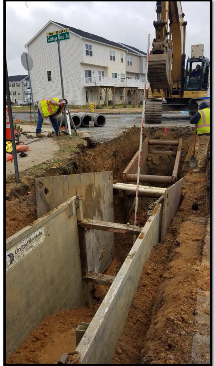
Trench boxes in place for installation of 18" Reinforced Concrete Pipe (RCP) between manholes D-12 and D-13 near STA 83+00.
