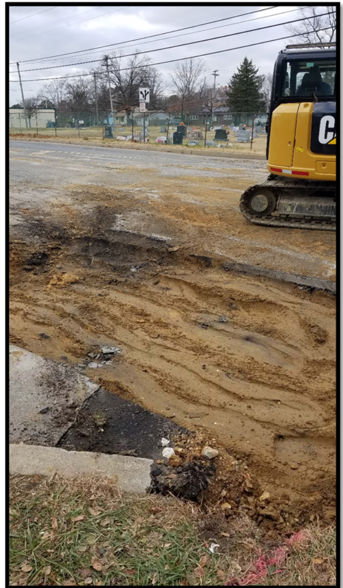
Trench between manholes D-12 and D-13 compacted after installation of 18" RCP.
