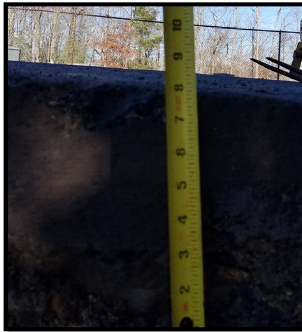
Trench between manholes D-12 and D-13 being boxed out for installation of Hot Mix Asphalt Trench Restoration.
