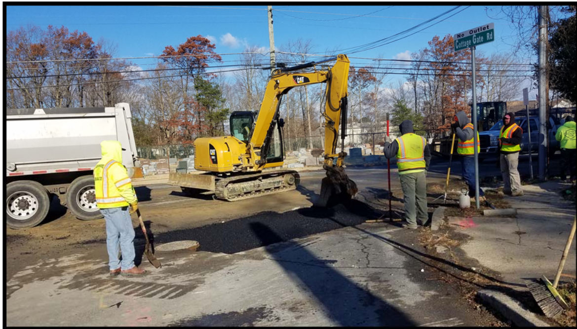
Trench restoration between manholes D-12 and D-13 being installed after installation of 18" RCP and compaction of subbase.
