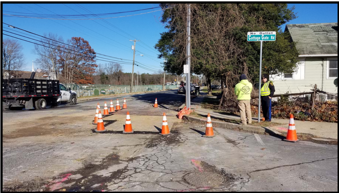
Delays caused by gas stub repair near STA 83+00 required steel plating overnight.
