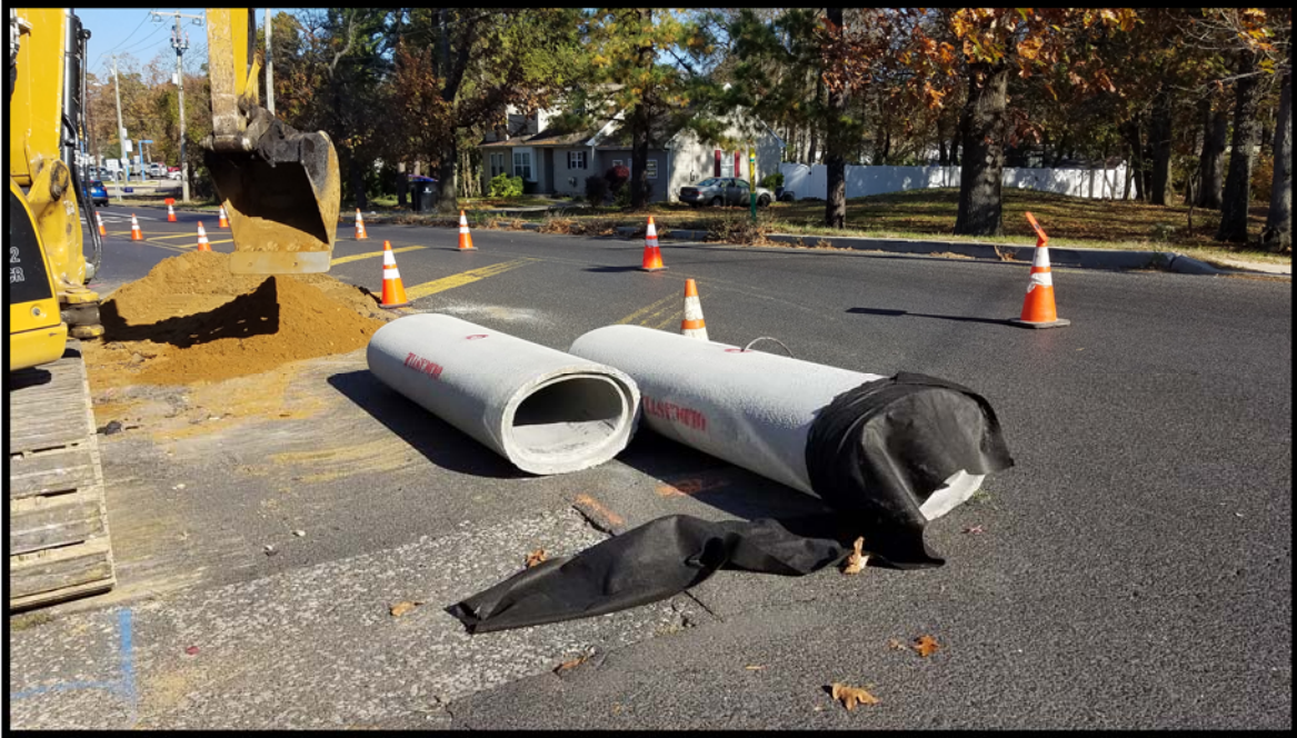
Horizontal Elliptical Reinforced Concrete Pipe (HERCP) at Kearlsey Road intersection being replaced with new HERCP.
