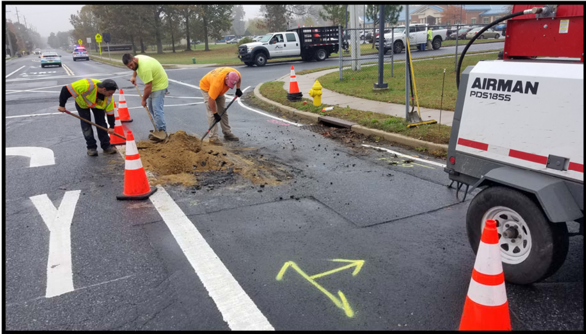
Underground utilities being located by test pits.
