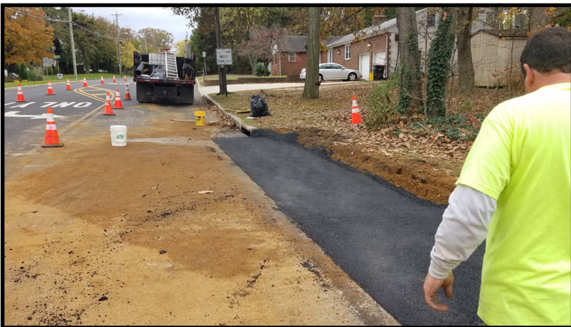
Horizontal Elliptical Reinforced Concrete Pipe (HERCP) at Kearsley Road intersection installed and trench restored with Hot Mix Asphalt.
