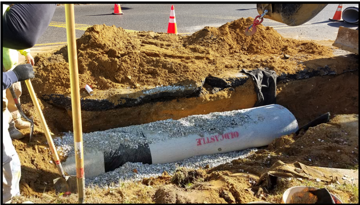
New Horizontal Elliptical Reinforced Concrete Pipe (HERCP) at Kearlsey Road intersection being installed.
