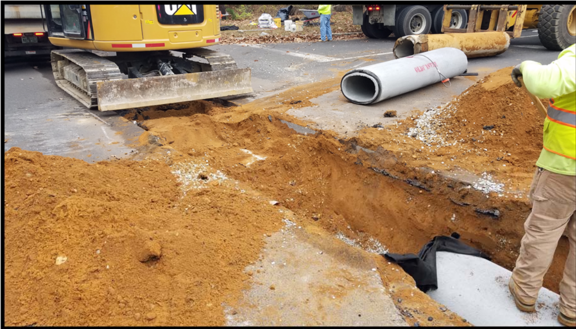
Trench for Horizontal Elliptical Reinforced Concrete Pipe (HERCP) at Kearsley Road intersection being backfilled.
