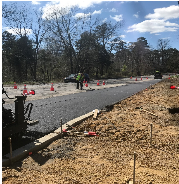
Figure 1: Crew installing Hot Mix Asphalt Base
