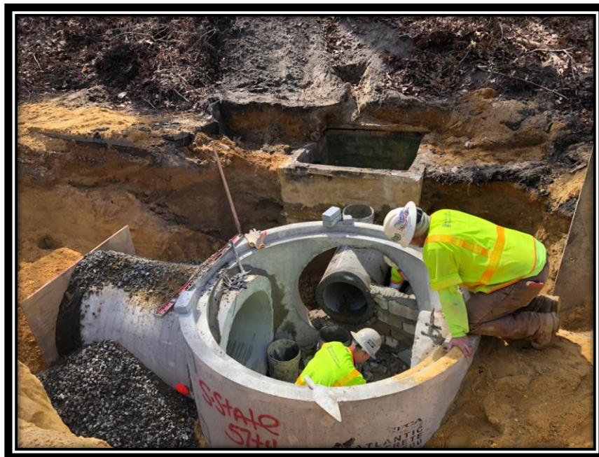
Figure: 2 – Installation of 6' diameter storm sewer manhole on Watsontown-New Freedom Road (CR 691) between Berlin-Clementon Road and Carriage Stop Drive in the Borough of Pine Hill
