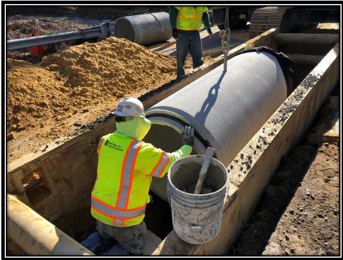
Figure: 1 – Installation of 36" RCP along the southbound lane of Watsonstown-New Freedom Road (CR 691) in the Borough of Pine Hill
