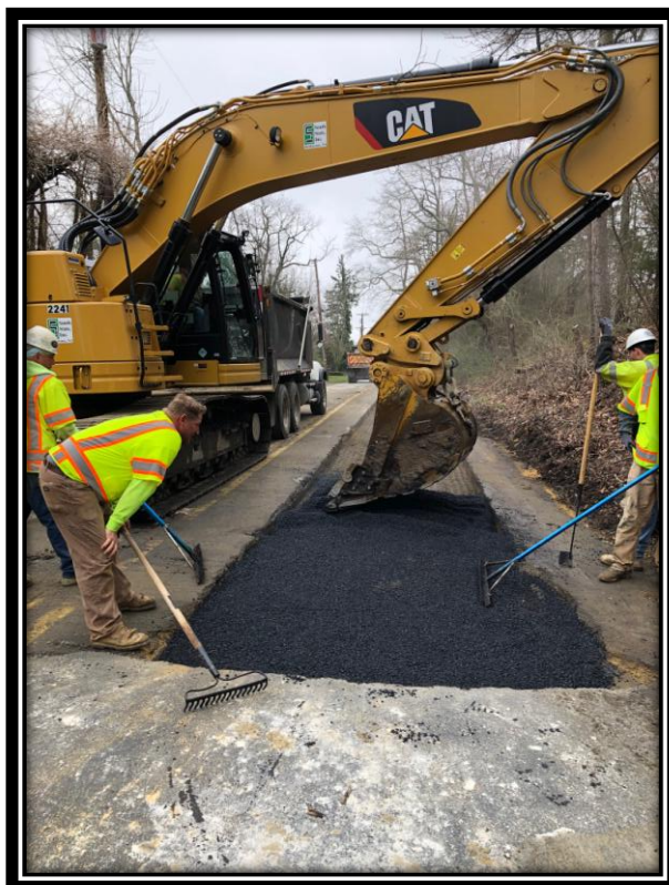
Figure: 3 – Asphalt restoration of the 36' RCP trench along the southbound lane of Watsontown-New Freedom Road (CR 691) in the Borough of Pine Hill
