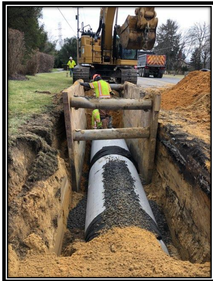
Figure: 1 – Installation of 36" RCP along the northbound lane of Watsonstown-New Freedom Road (CR 691) in the Borough of Berlin
