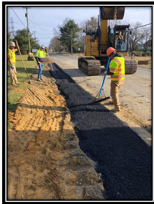
Figure: 3 – HMA restoration of the 24" RCP trench along the northbound lane of Watsontown-New Freedom Road (CR 691) in the Borough of Berlin
