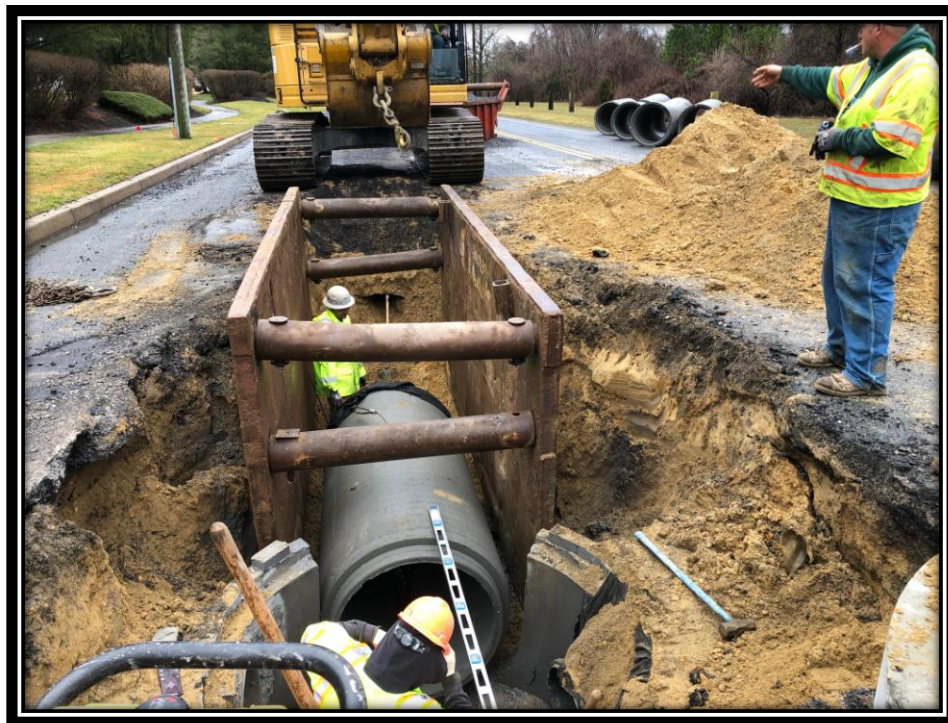
Figure: 2 – Installation of 36" RCP along the northbound lane of Watsontown-New Freedom Road (CR 691) in the Borough of Berlin
