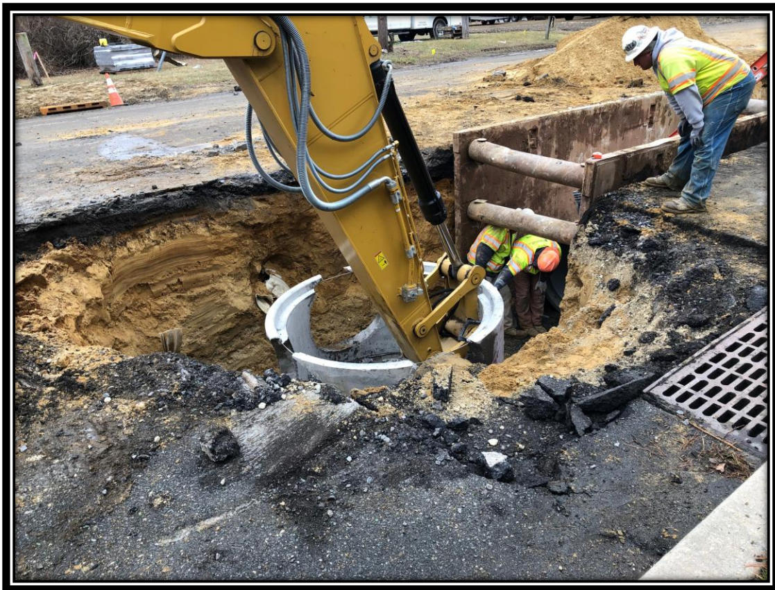
Figure: 1 – Installation of 6' diameter storm sewer manhole along the northbound lane of Watsonstown-New Freedom Road (CR 691) in the Borough of Berlin
