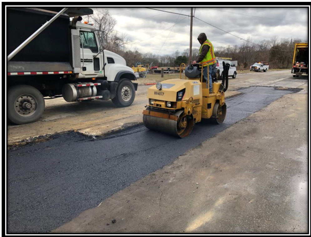
Figure: 3 – HMA restoration of the 36" RCP trench along the northbound lane of Watsontown-New Freedom Road (CR 691) in the Borough of Berlin
