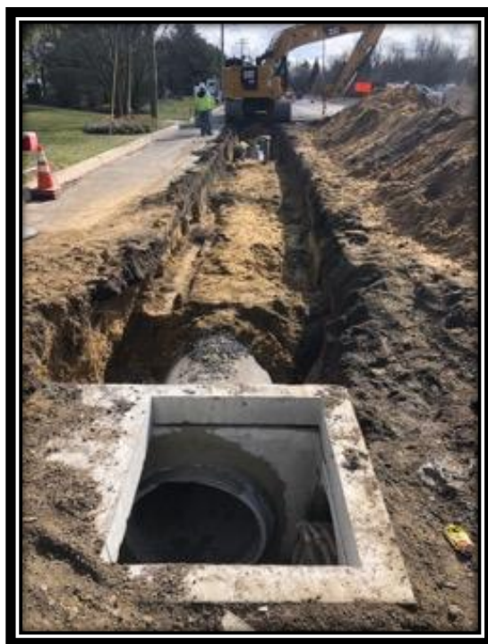
Figure: 3 – Installation of 36" RCP along the northbound lane of Watsonstown-New Freedom Road (CR 691) in the Borough of Berlin approaching Carriage Stop Drive
