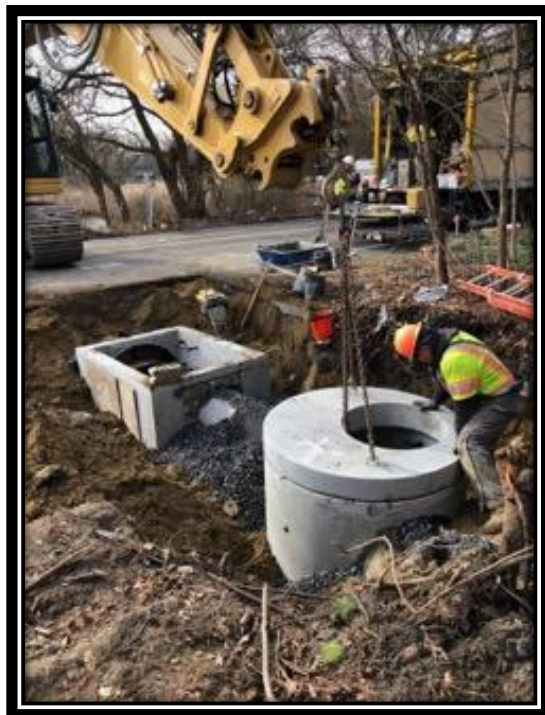
Figure: 2 – Installation of 4' diameter storm sewer manhole, type B inlet and 18" RCP along the northbound lane of Watsonstown-New Freedom Road (CR 691) in the Borough of Berlin
