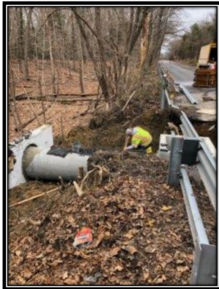
Figure: 1 – Installation of 30” concrete headwall, type B inlet and 30” RCP along the southbound lane of Watsonstown-New Freedom Road (CR 691) in the Borough of Pine Hill
