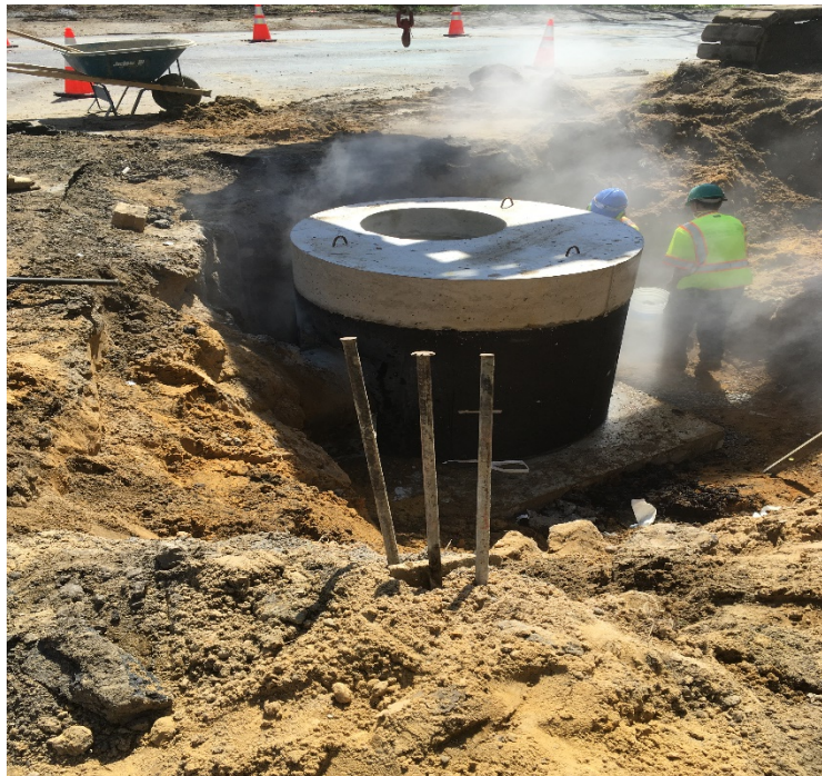
Figure 1: Crew installing Doghouse
