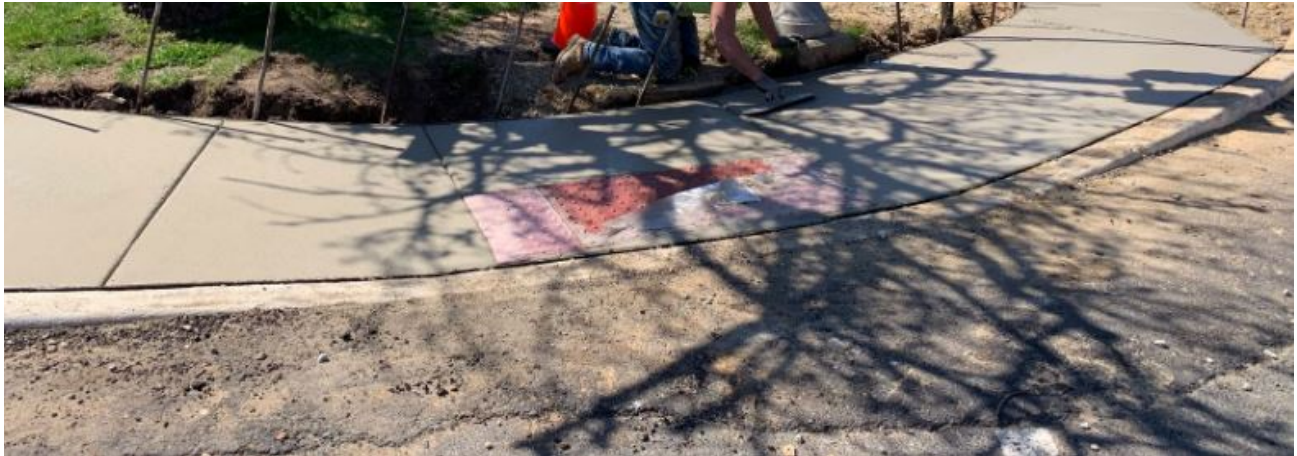
Figure 1: Concrete curb ramp placed
