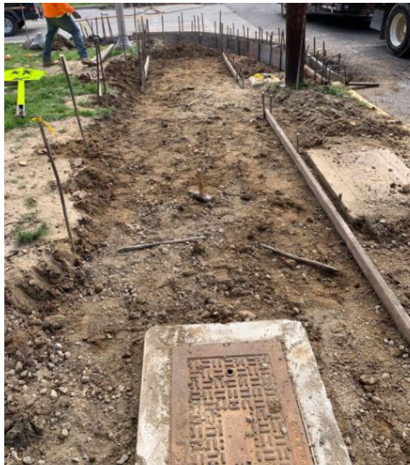
Figure 2: Forms for concrete curb and sidewalk
