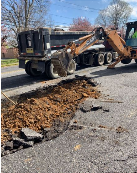
Figure 4: Excavation for proposed curb
