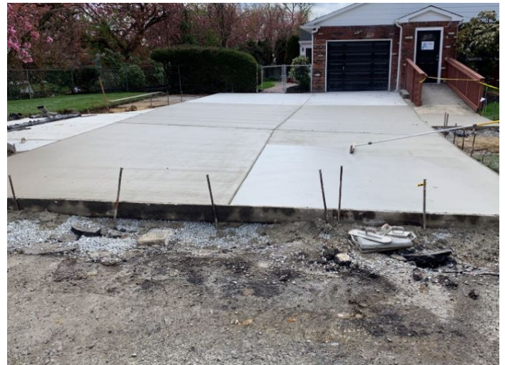
Figure 3: Concrete reinforced driveway placed
