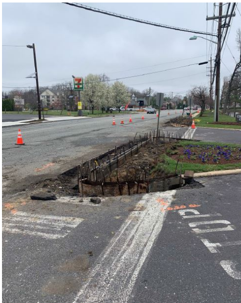
Figure 2: Concrete curb forms
