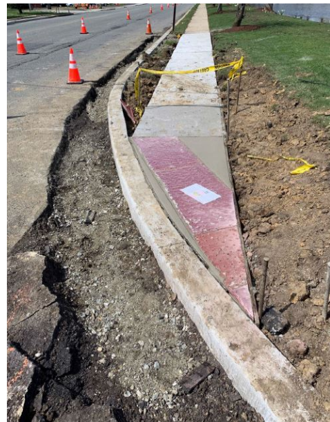
Figure 3: Concrete curb ramp placed
