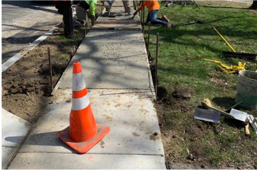
Figure 1: New concrete sidewalk
