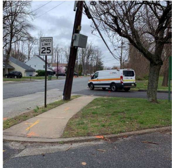
Figure 5: Utility mark out
