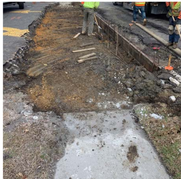
Figure 3: Removing apron
