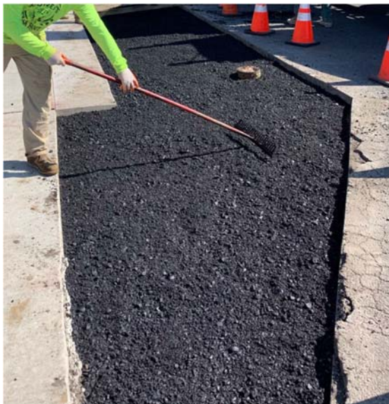
Figure 2: Asphalt repair
