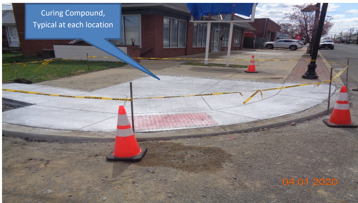
Figure 5: West Concrete curb, sidewalk and HC Ramp at Hollinshead Avenue along Westfield Avenue, RT.
