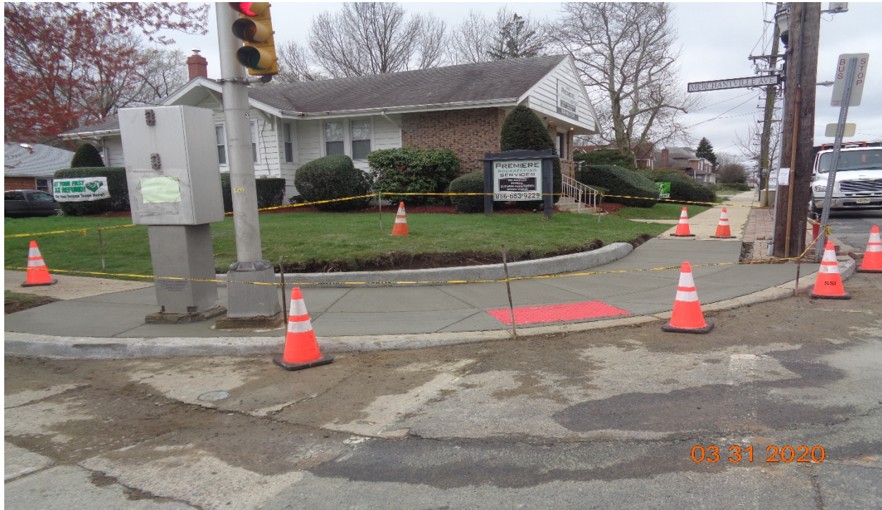
Figure 1: West Concrete curb, sidewalk and HC Ramp at Merchantville Avenue along Westfield Avenue, RT
