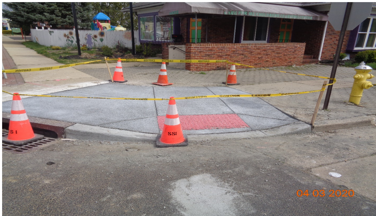
Figure 7: East Concrete curb, sidewalk and HC Ramp at Hillcrest Avenue along Westfield Avenue, RT.
