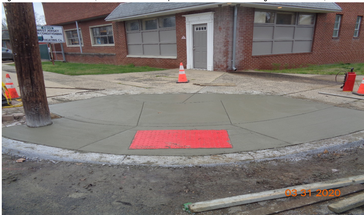
Figure 2: East Concrete curb, sidewalk and HC Ramp at Gross Avenue along Westfield Avenue, RT.
