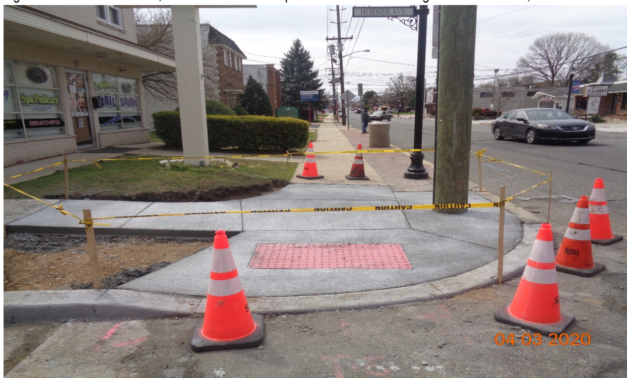
Figure 8: West Concrete curb, sidewalk and HC Ramp at Horner Avenue along Westfield Avenue, RT.
