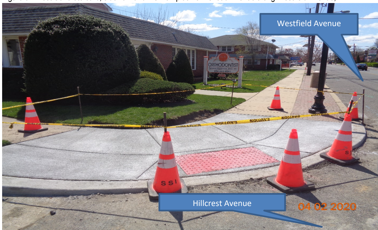
Figure 6: West Concrete curb, sidewalk and HC Ramp at Hillcrest Avenue along Westfield Avenue, RT.
