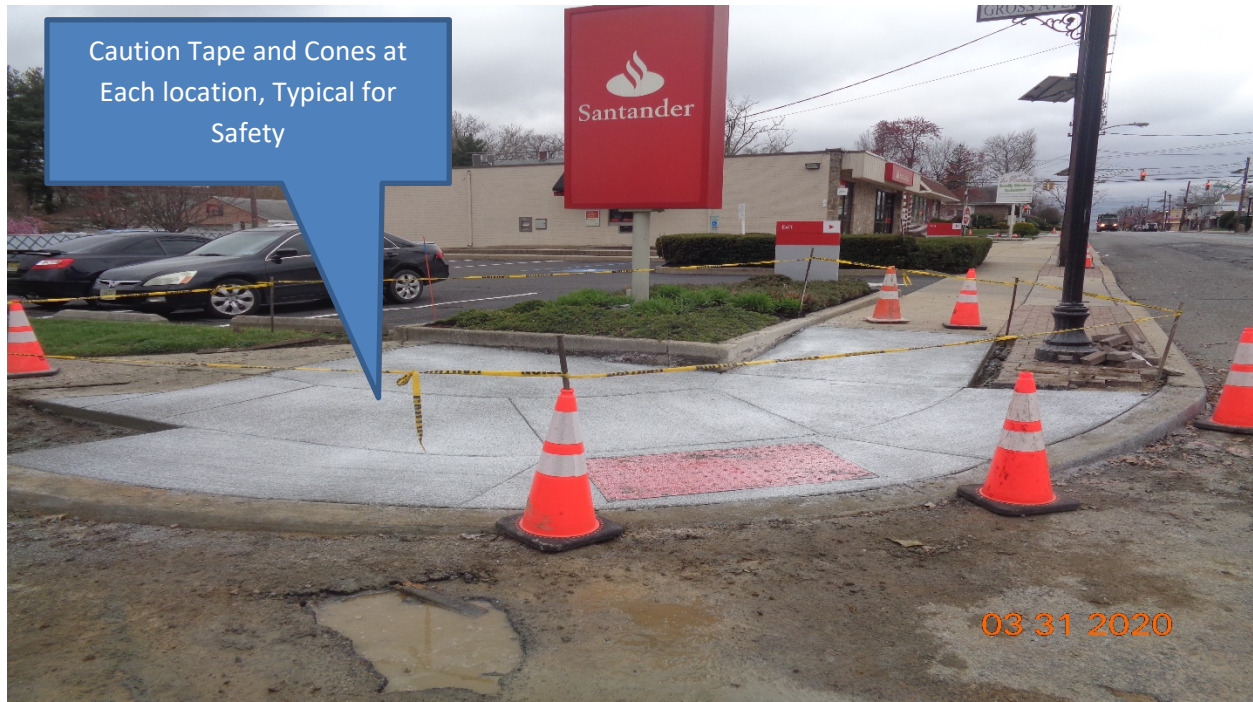
Figure 3: West Concrete curb, sidewalk and HC Ramp at Gross Avenue along Westfield Avenue, RT.
