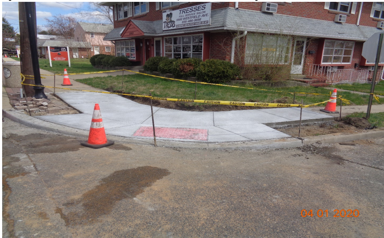
Figure 4: East Concrete curb, sidewalk and HC Ramp at Hollinshead Avenue along Westfield Avenue, RT.
