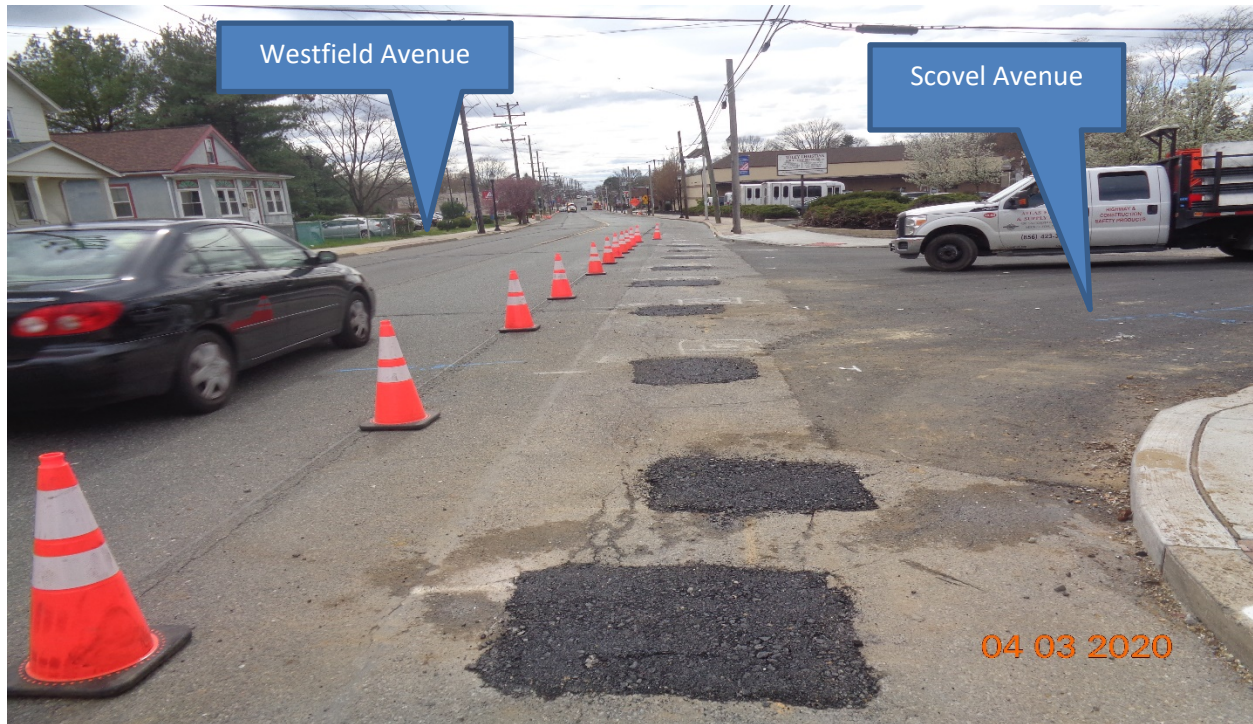
Figure13: Gas leak fixing is under progress along Westfield Avenue at Scovel Avenue
