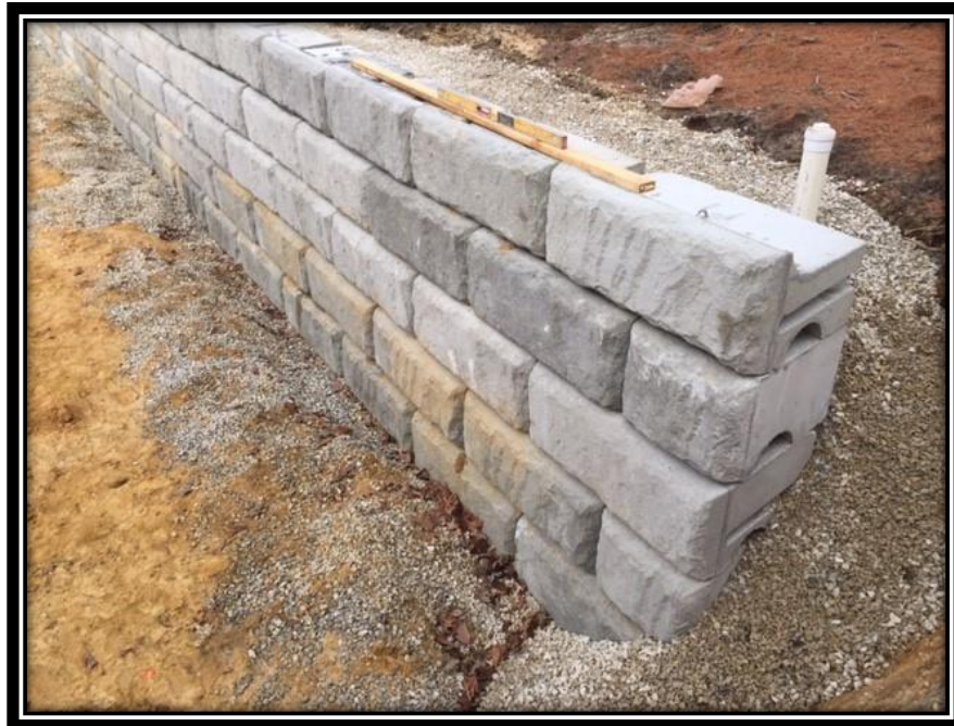
Figure 1: Contractor installing the REDI-ROCK cap block on the east retaining wall.
