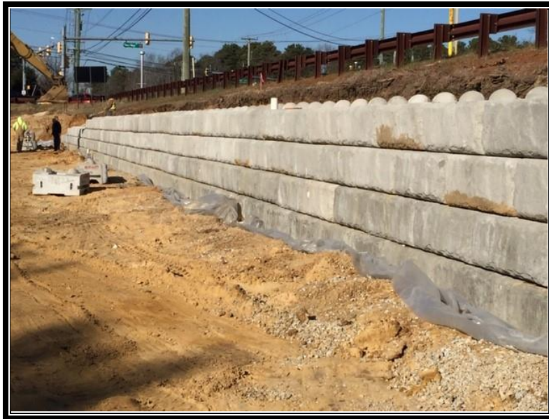
Figure 3: East retaining wall progress using REDI-ROCK..
