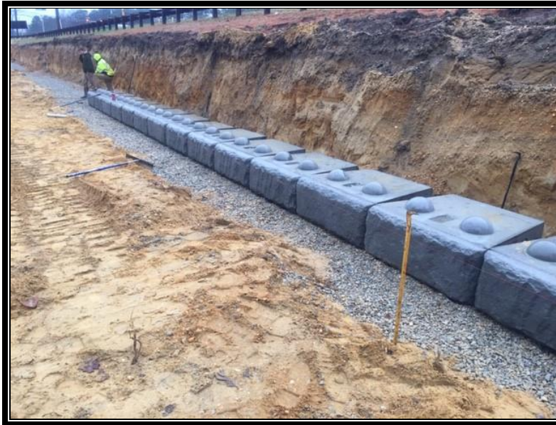
Figure 2: Crew installing the first level of REDI-ROCK retaining wall block..
