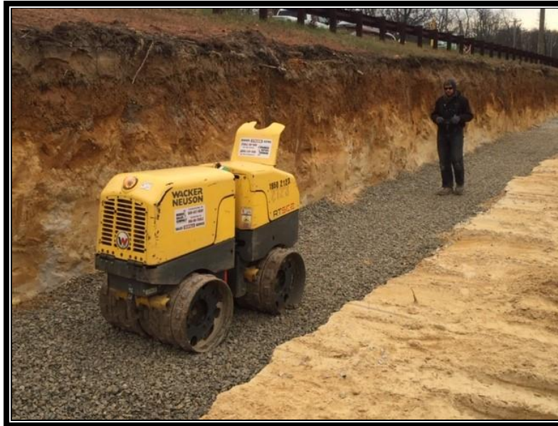
Figure 2: Crew using a walk-behind sheep's foot roller to achieve compaction.
