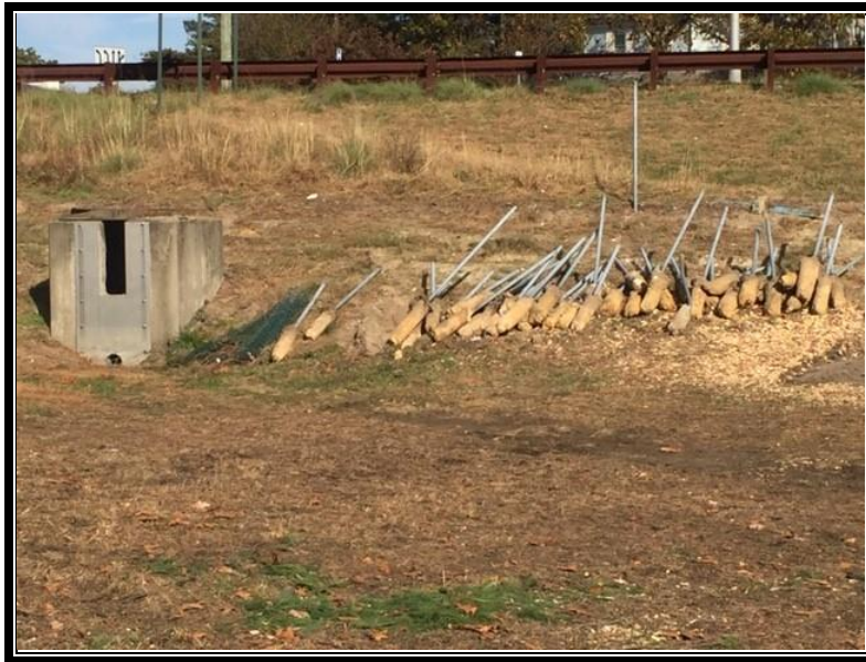
Figure 3: Crew stockpiling galvanized fence post for concrete removal.
