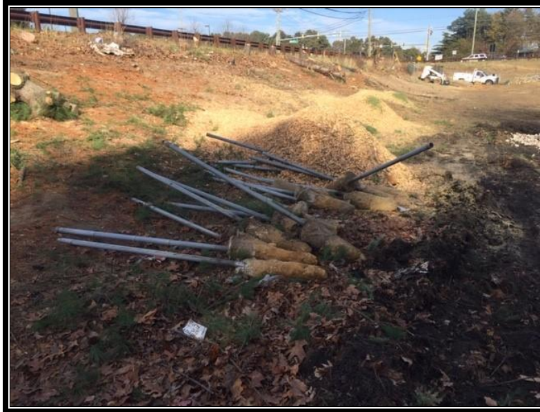
Figure 2: Crew removing the galvanized fence post from the chain-link fence.
