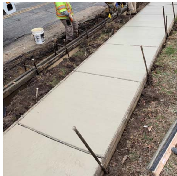
Figure 3: New concrete sidewalk and forms for vertical curb
