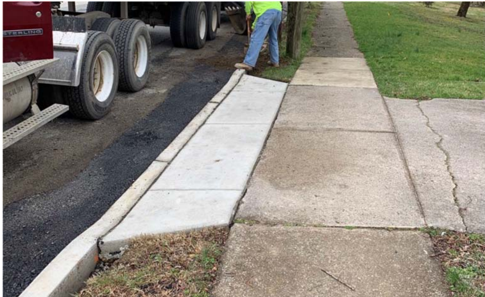
Figure 1: New Concrete driveway apron, curb and topsoil
