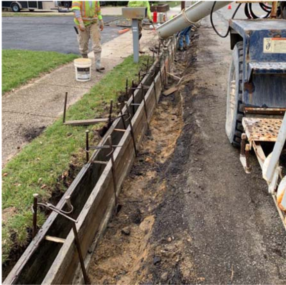
Figure 4: Pouring vertical curb
