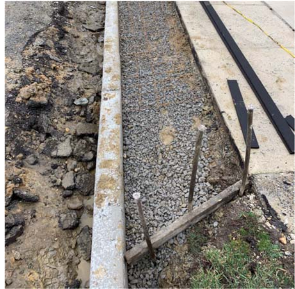
Figure 5: Forming new concrete apron
