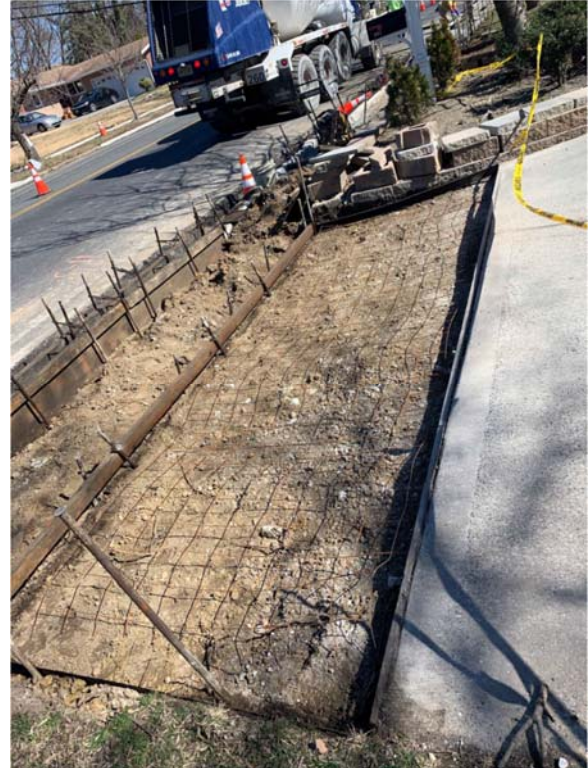
Figure 5: Driveway apron formed up
