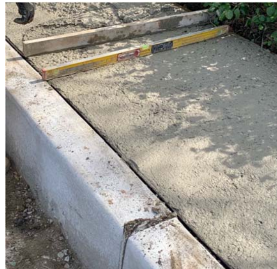
Figure 3: Checking sidewalk for correct grading with a smart level
