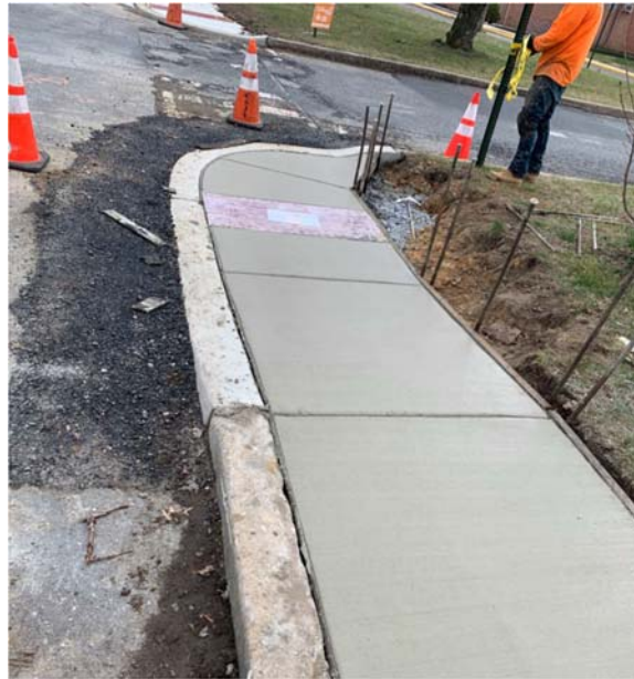
Figure 1: Concrete sidewalk placed
