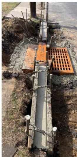
Figure 2: Concrete curb placement
