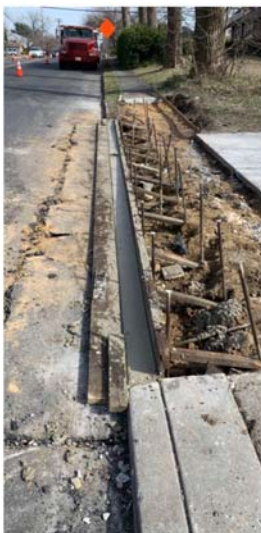
Figure 2: Concrete curb placement
