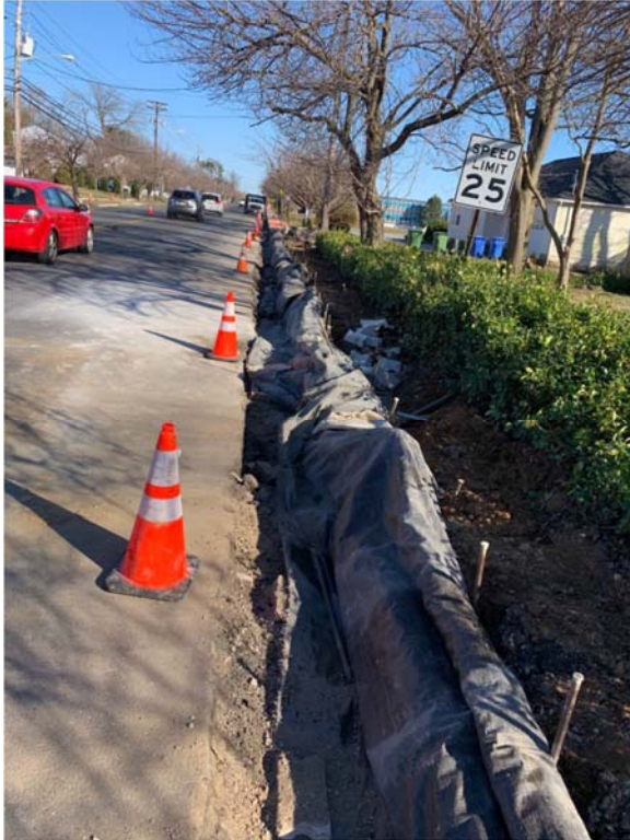
Figure 4: Concrete curb covered with blankets
