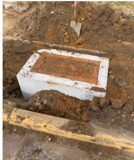
Figure 5: Junction box installed
