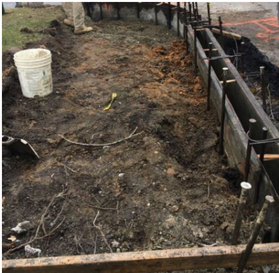
Figure 4: Sidewalk removed and curb formed up
