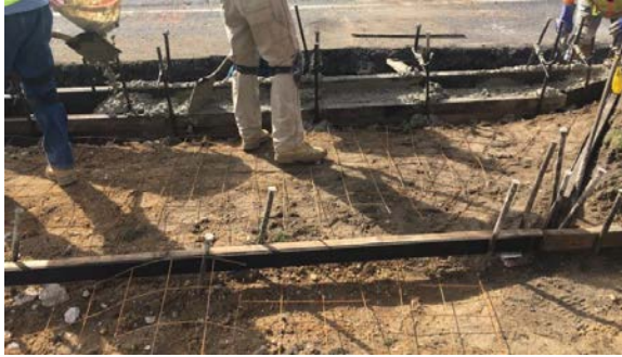
Figure 2: Concrete curb placement
