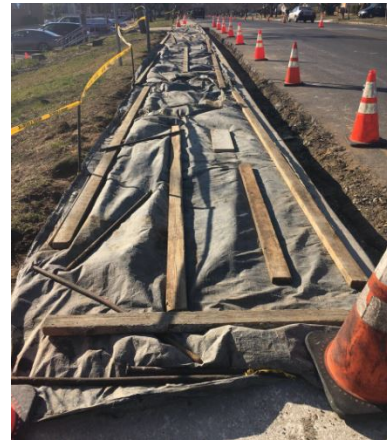
Figure 3: Concrete sidewalk covered with blankets
