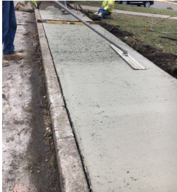
Figure 1: Concrete sidewalk placed
