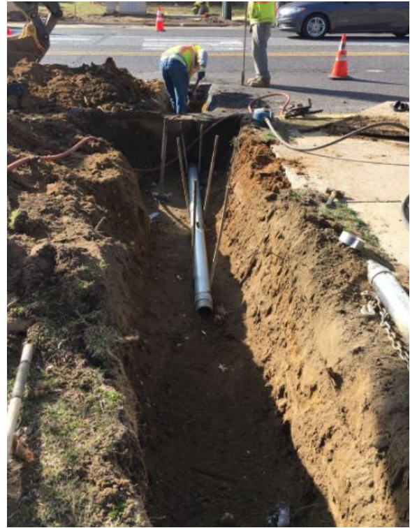
Figure 5: RMC installation
