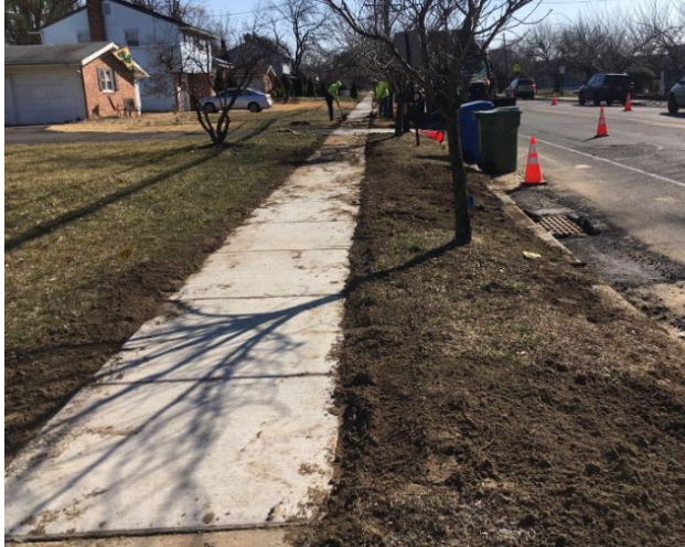
Figure 4: Topsoiling operations
