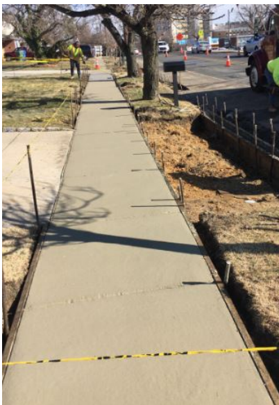
Figure 2: Concrete sidewalk placed
