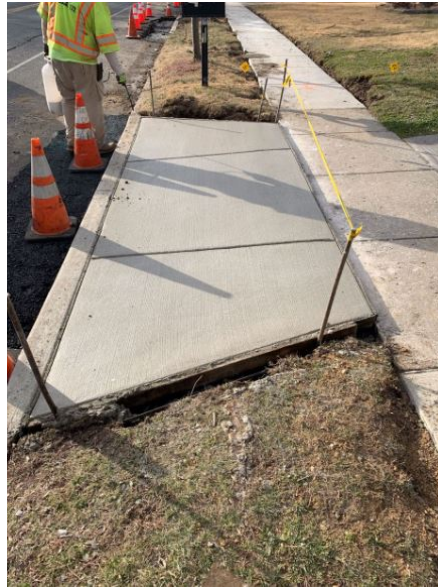
Figure 1: Concrete driveway placed
