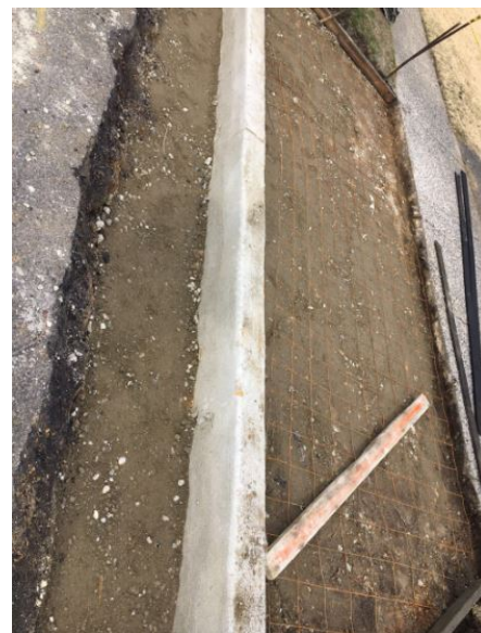
Figure 3: Concrete curb and DGA subbase
