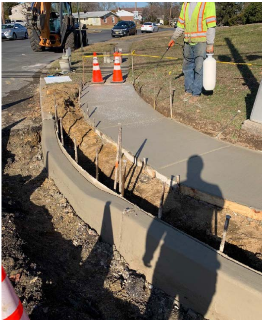
Figure 2: Concrete curing application
