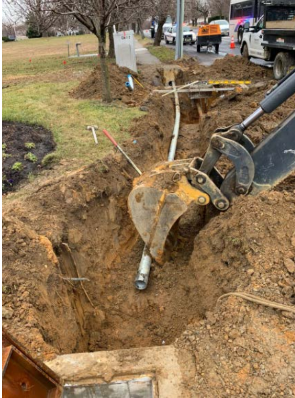
Figure 4: RMC installation
