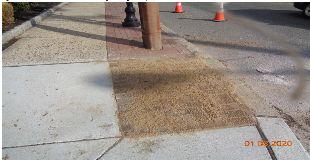
Figure 8: Scovel Avenue East – Resetting existing brick pavers.
