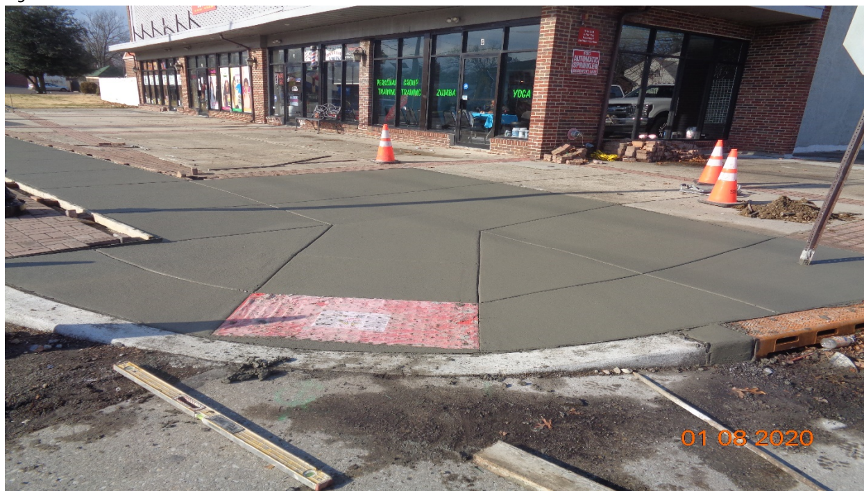
Figure 4: Hillcrest Avenue Construction of west handicap ramp.
