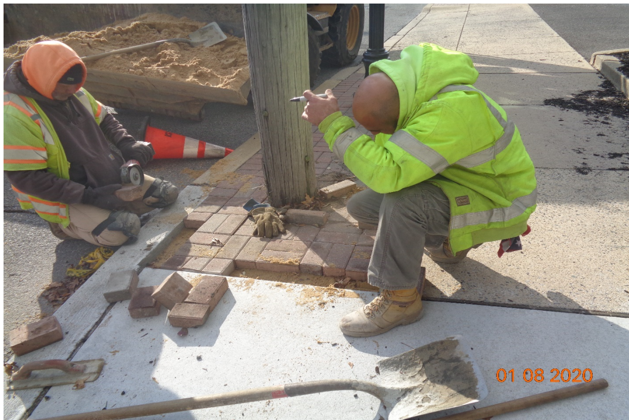
Figure 7: Scovel Avenue West – Resetting existing brick pavers.
